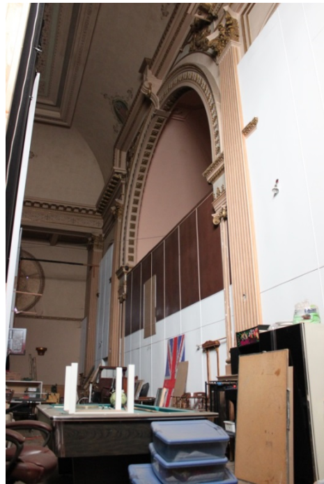
FIGURE 32. CHURCH: SANCTUARY SHOWING SEALED ALTAR NICHES, 2016.
