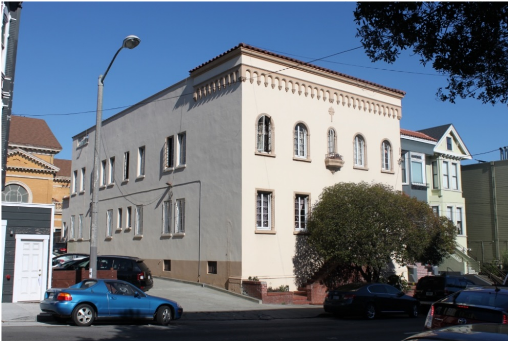
FIGURE 47. CONVENT LOOKING NORTHEAST FROM OAK ST., 2015.
