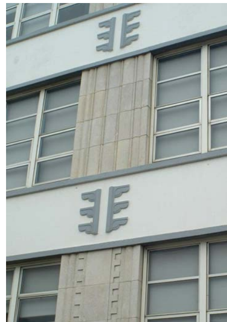
Figure 14. Primary façade, detail of piers, molding, and "tree and leaf" bas-relief ornament; view toward northeast.
