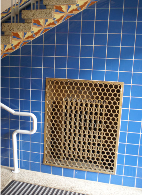
Figure 44. Tiled wainscoting and decorative metal radiator screen.
