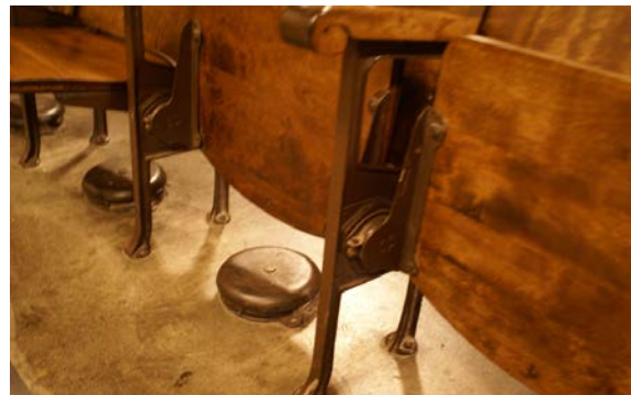
Figure 41. Heating units beneath seats.
