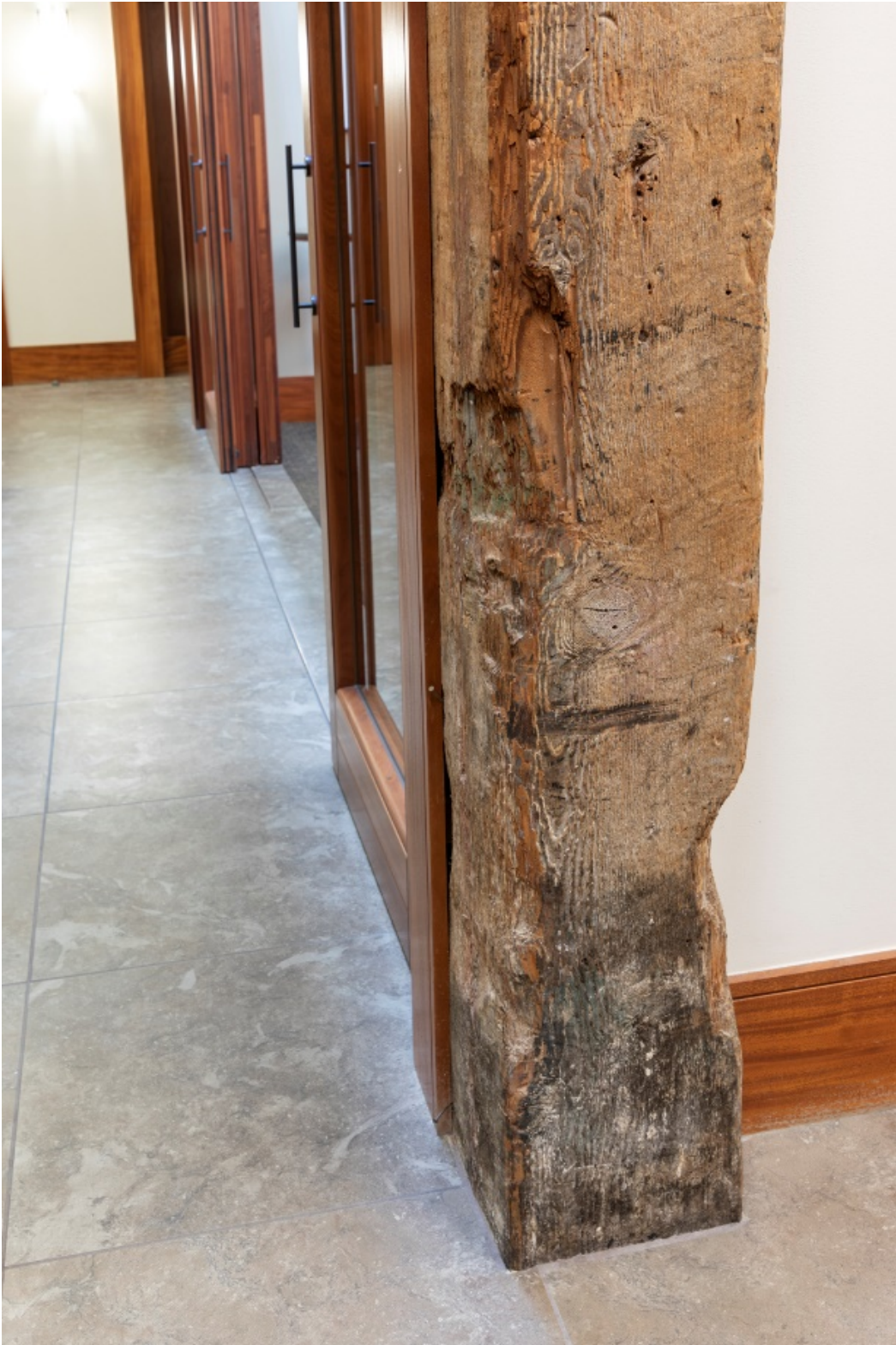
Figure 27: Wood support pillar, ground floor, 2019. Looking north. Courtesy of Henrik Kam.
