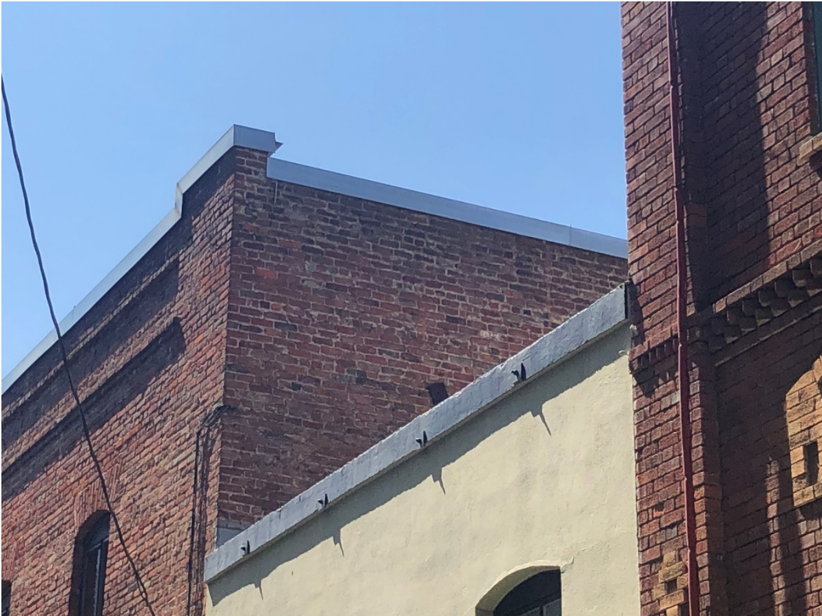
Figure 23: Partially visible north (rear) façade, 2020. Looking southwest.
