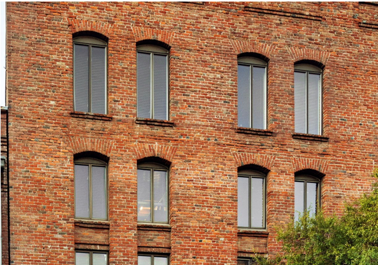
Figure 9: Primary facade 2019, looking north. Courtesy of Henrik Kam.
