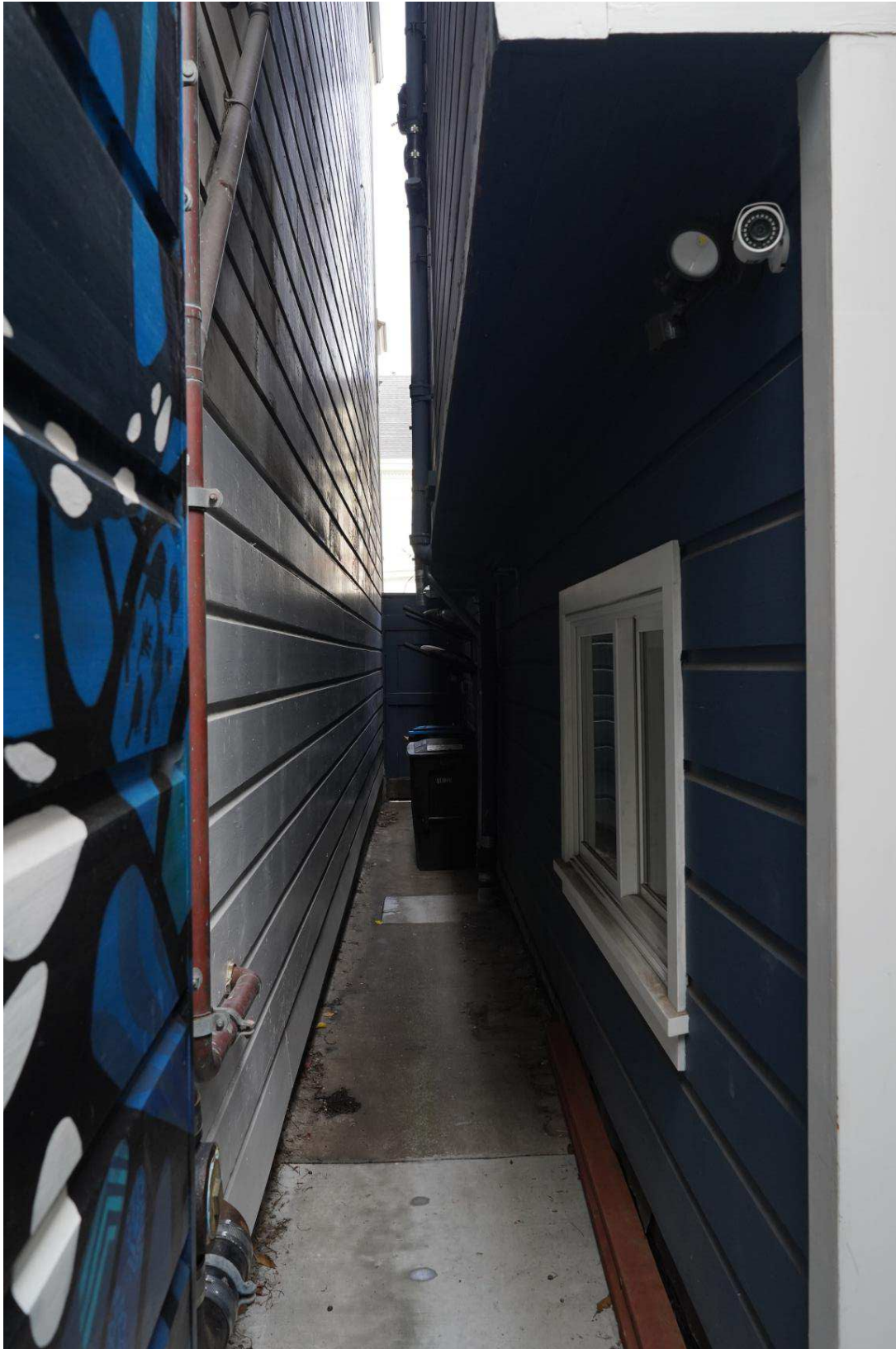
Figure 31. Southeast façade at basement level, view northwest.
