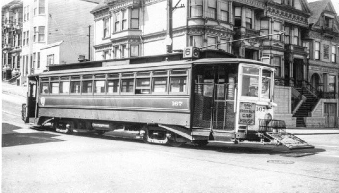
Figure 4. Masonic Avenue and Waller Street, 1937, Whelan House visible far right.
