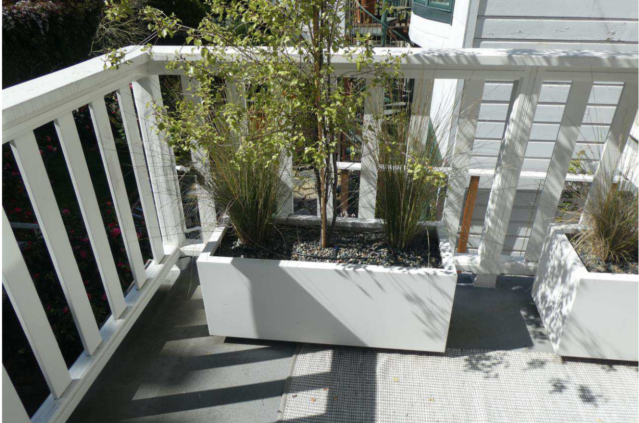
Figure 54: Detail showing the asphaltic roof at the decking above the first floor kitchen.
