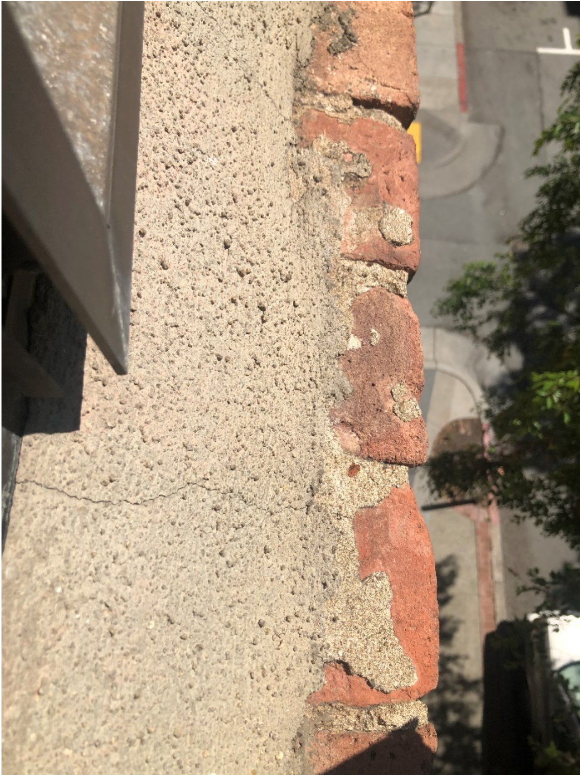
Figure 15: Cementitious parge slope drain in window sill. Looking down, primary façade. 2020.
