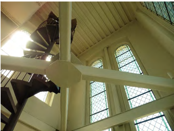
Figure 28. West tower, featuring seismic bracing and a spiral staircase. Source: Page & Turnbull, April 2019.
