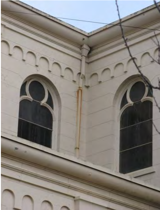
Figure 40a. West façade, showing blocked or perforated drainage which is causing damage to interior plaster.
