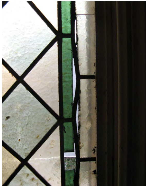
Figure 42c. Breakage and loss of colored glass panes due to distortion of lead comes.
