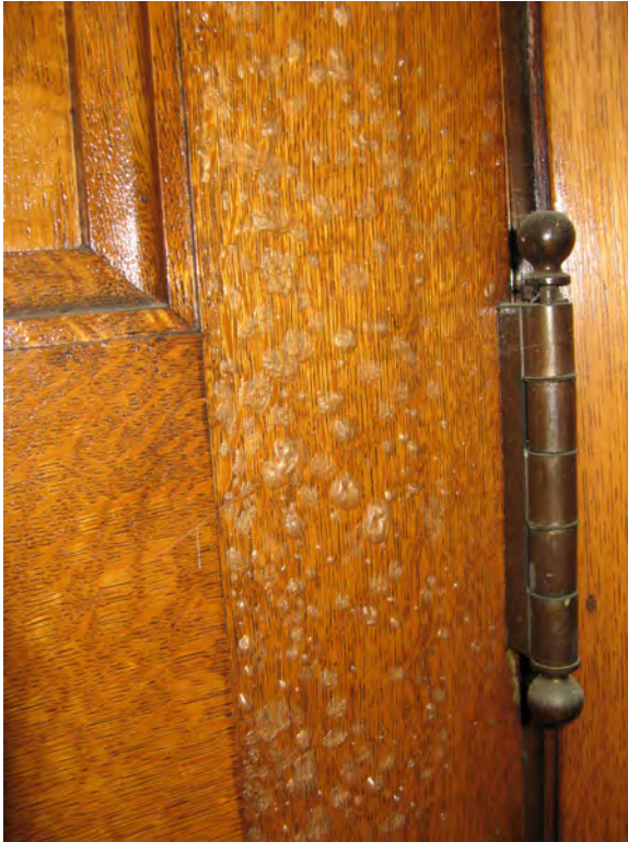
Figure 41a. Blistering of varnish on an oak door caused by moisture penetration.
