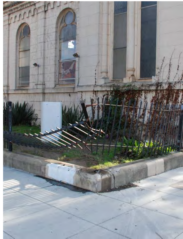
Figure 32b. Damage to metal fence at northeast corner of property.
