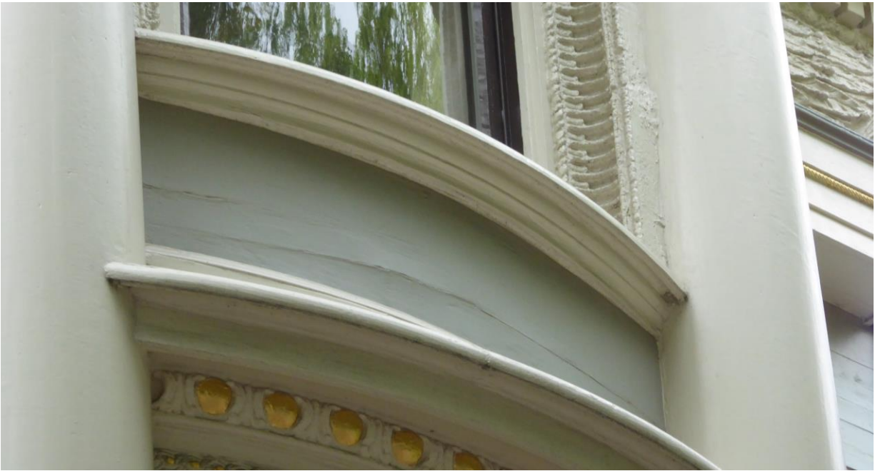
Figure 26: Detail of split wood panel between windows.
