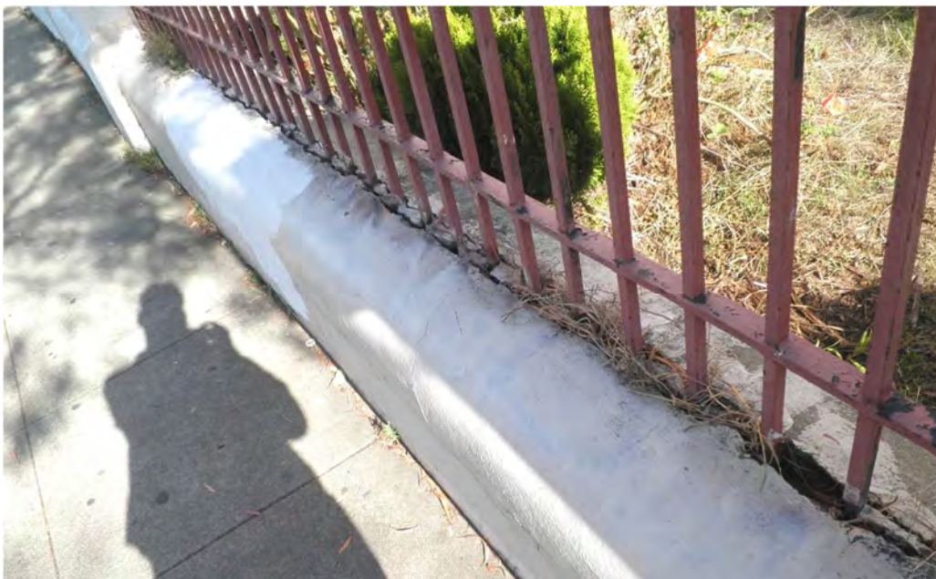
Figure 32c. Low brick wall along Howard Street, showing gaps and voids, corroded metal fence, and graffiti (painted over with mismatched paint).
