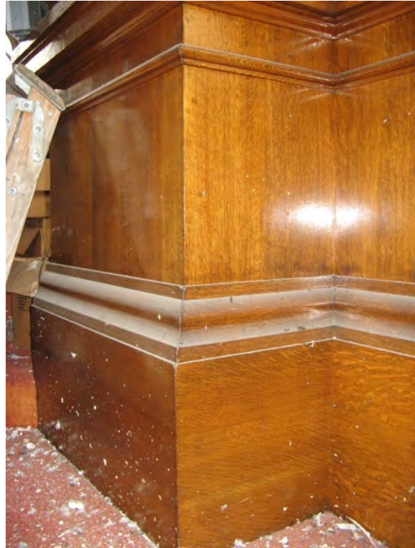
Figure 41b. Dust (on molding) and paint/guano spatters can cause permanent damage to wood finish.
