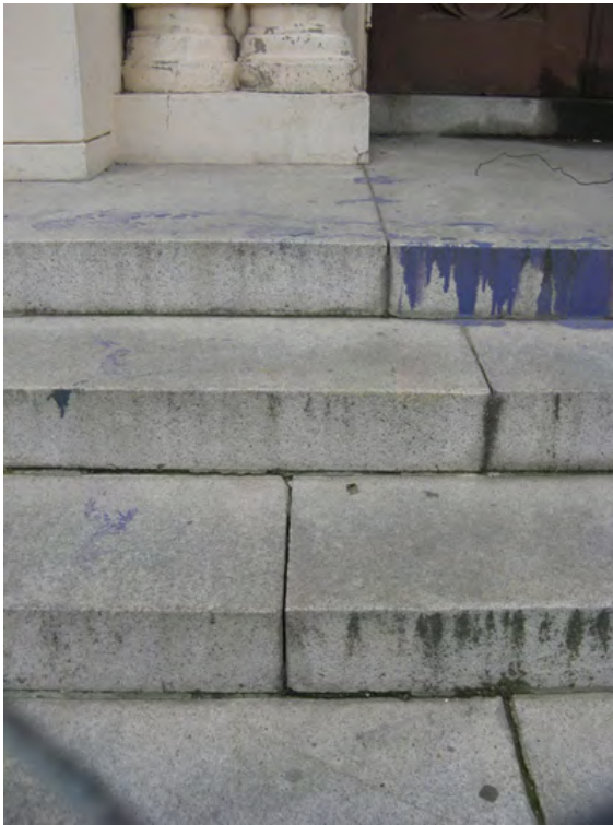
Figure 33a. Main portal steps, showing soiling, paint stains and vertical joints without mortar.
