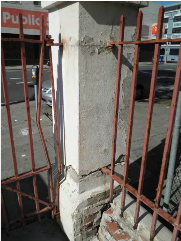
Figure 32a. Pier near west tower, showing large cracks and displaced areas of brick (arrow) and corroded metal fence.
