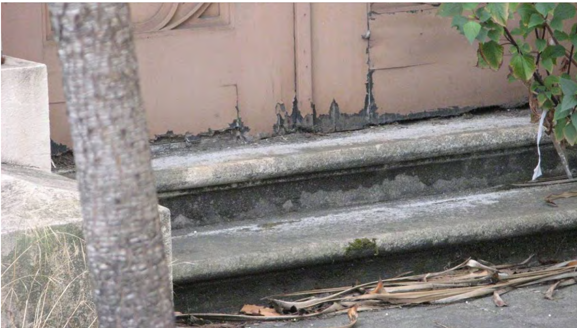
Figure 33c. East transept, north portal steps, showing decorative bull nose with biological growth and soiling.
