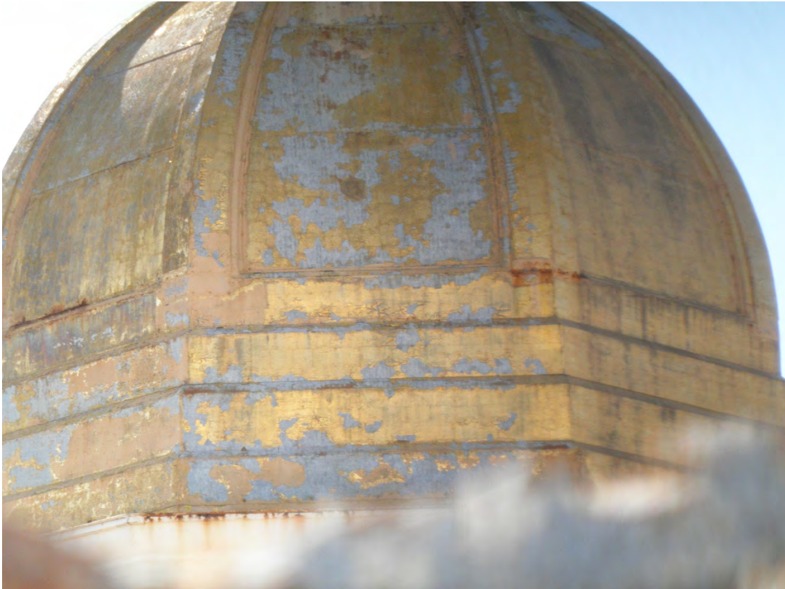
Figure 36c. Detail, corrosion and loss of paint and gilding at domes.
