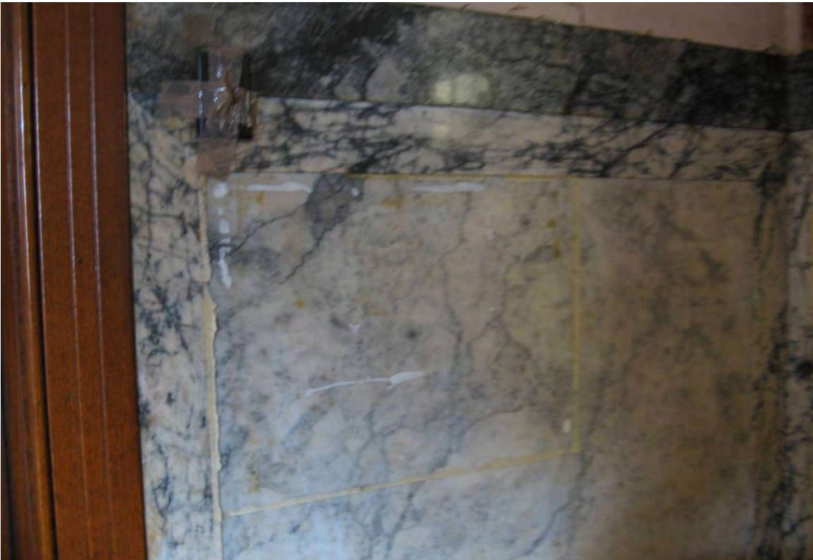
Figure 39b. Detail, showing tape and adhesive residue.
