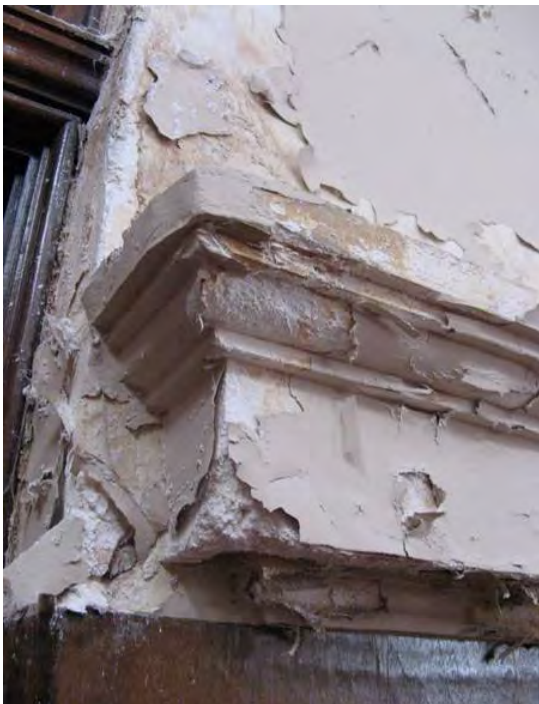
Figure 40c. Softening and deterioration of decorative plaster elements caused by moisture from faulty roofing.
