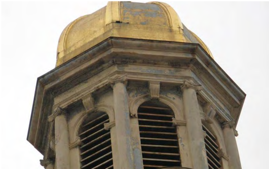
Figure 37c. East tower detail, constructed entirely of pressed sheet metal, showing missing architectural detail, loss of gilding and protective paint, and corrosion stains. Birds were nesting inside the towers.
