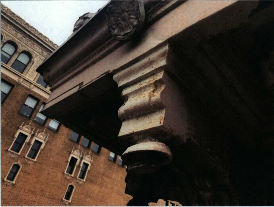
Image 3: Conditions on both the South and West cornices are poor.
