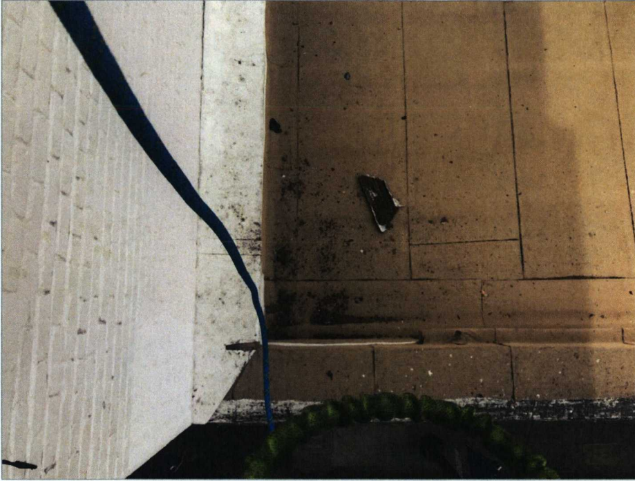
Image 4: Loose sections of the cornice have fallen onto the adjacent rooftop.
