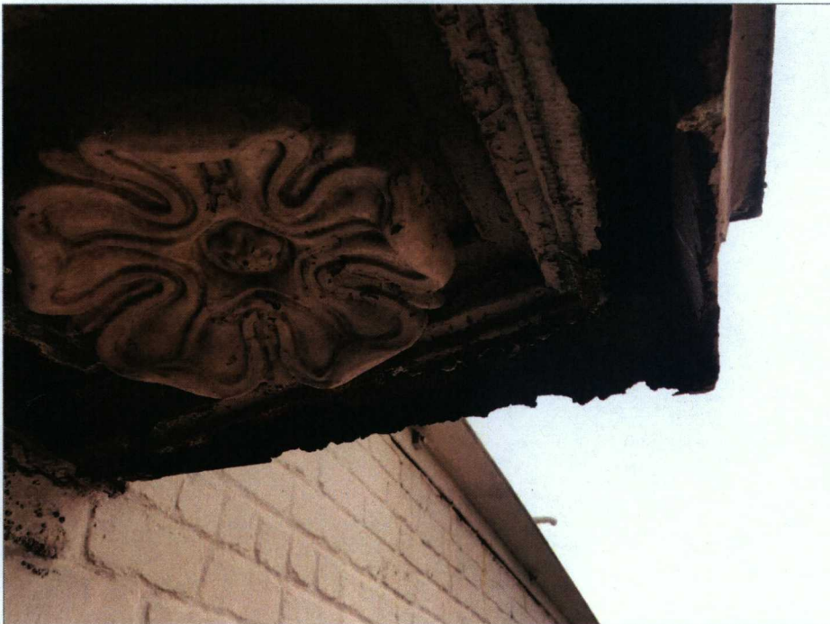
Image 4: Sections of sheet metal have rusted through exposing the interior of the cornice.
