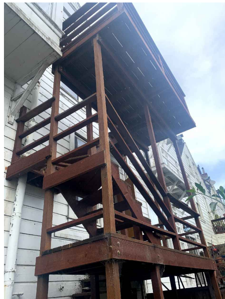
FIG. 3: REAR MULTI-STORY WOOD DECK
