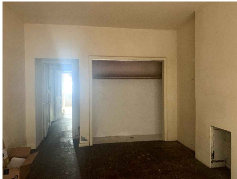
FIG.2: NEW WALLS CONVERTED DOUBLE-PARLOR TO BEDROOM ON ENTRY LEVEL
