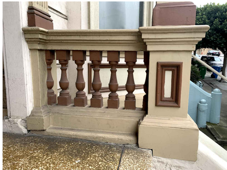
FIG. 2: EXISTING FRONT STAIR LANDING AT PORCH
