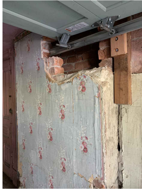
FIG.2: BRICK IN CHIMNEY
