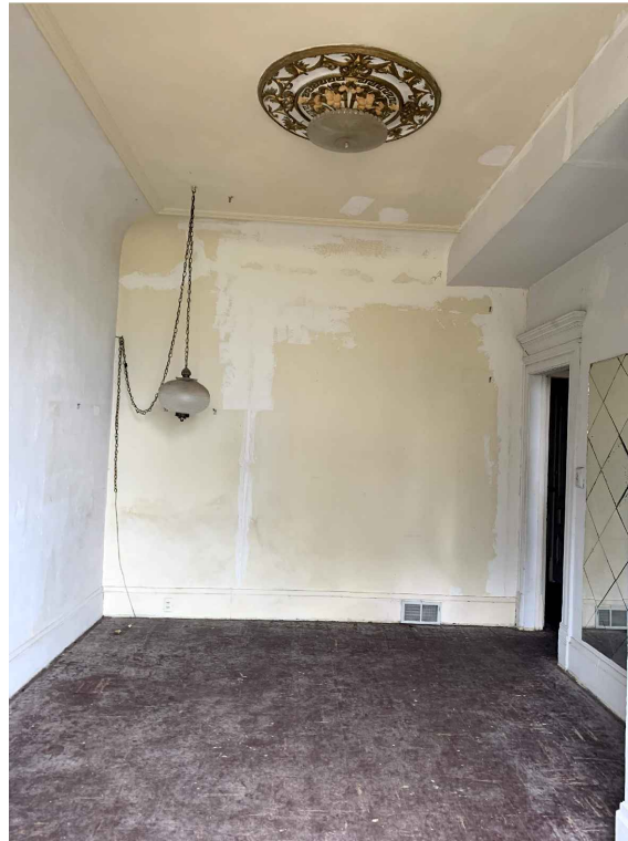
FIG.4: INTERIOR DOOR OPENINGS INFILLED TO CREATE COMMON ENTRY HALL
