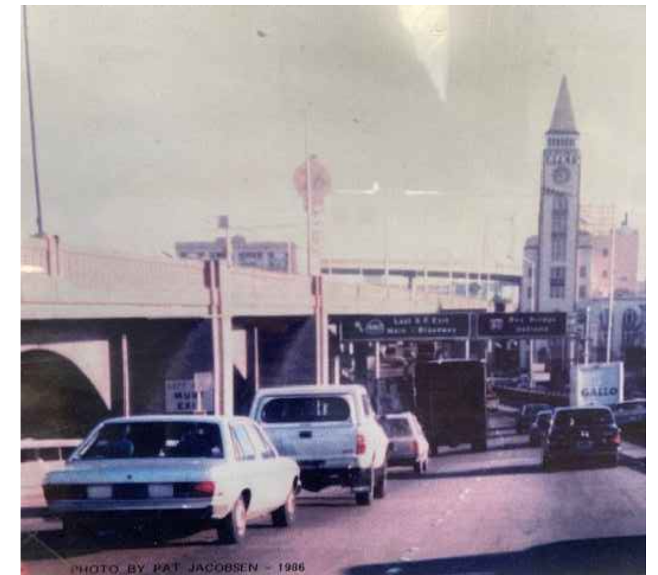
6 VIEW OF CLOCKTOWER BUILDING, 1986 PC: PAT JACOBSEN
