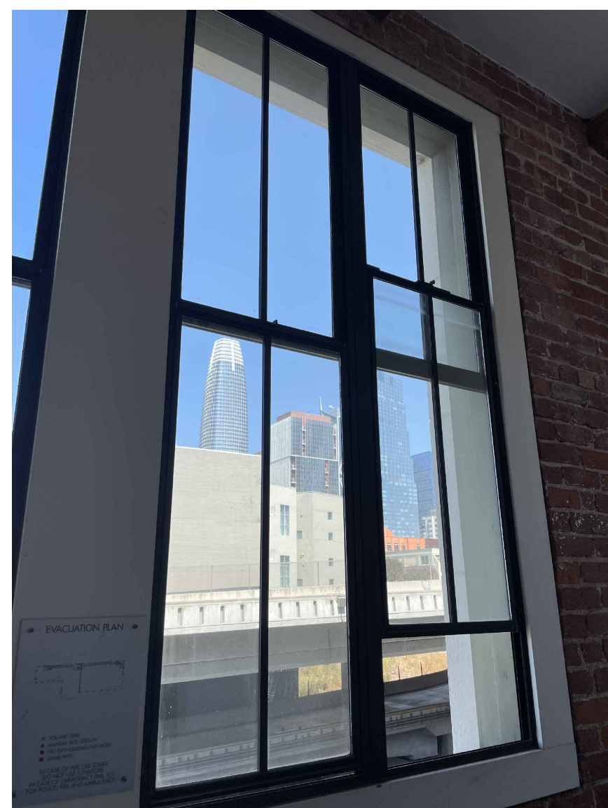
5 EXISTING DOUBLE-HUNG 2-OVER-2 METAL WINDOWS PC: ARG/CS
