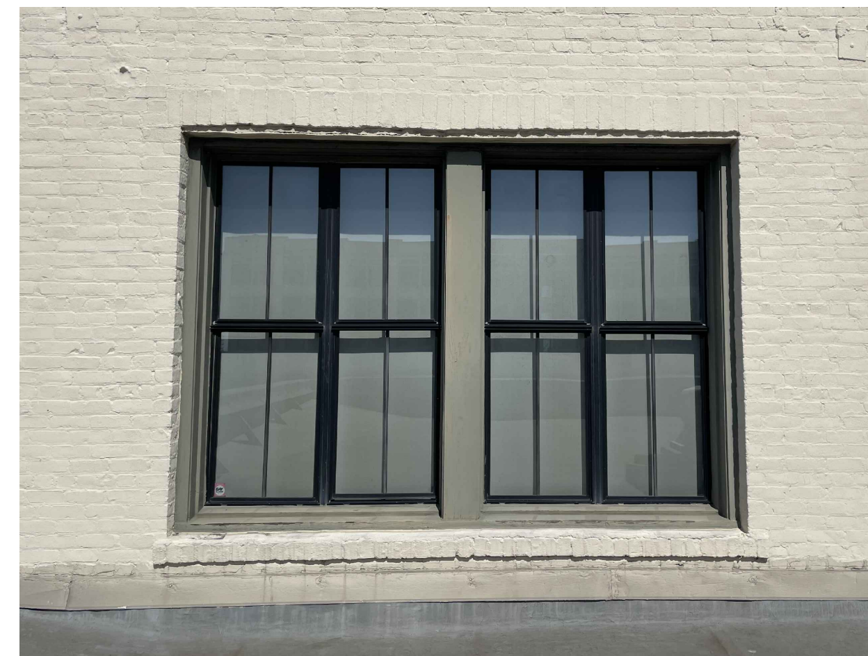
4 EXISTING DOUBLE-HUNG 2-OVER-2 METAL WINDOWS PC: ARG/CS
