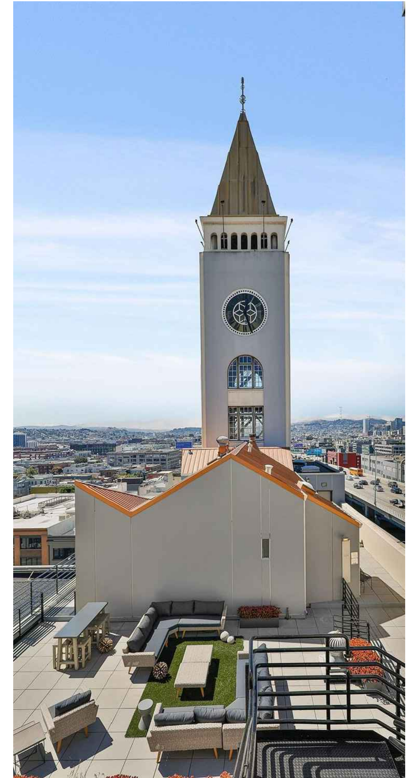
4 EAST ELEVATION, 2019 PC: OPEN HOMES PHOTOGRAPHY, VIA COMPASS.COM
