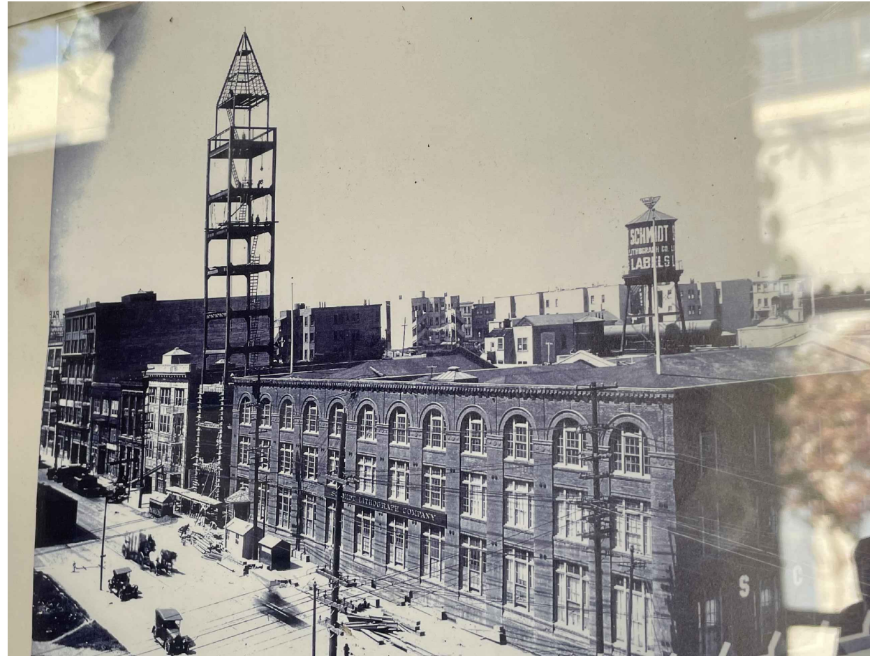
1 STEEPLE TOWER IN CONSTRUCTION, DATE UNKNOWN PC: UNKNOWN
