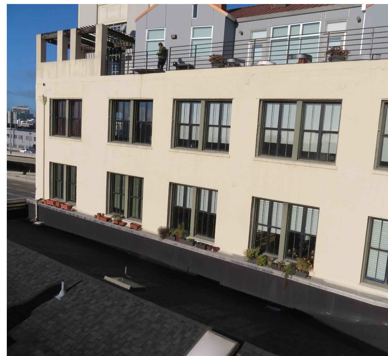
3 EXISTING DOUBLE-HUNG 2-OVER-2 METAL WINDOWS PC: ARG
