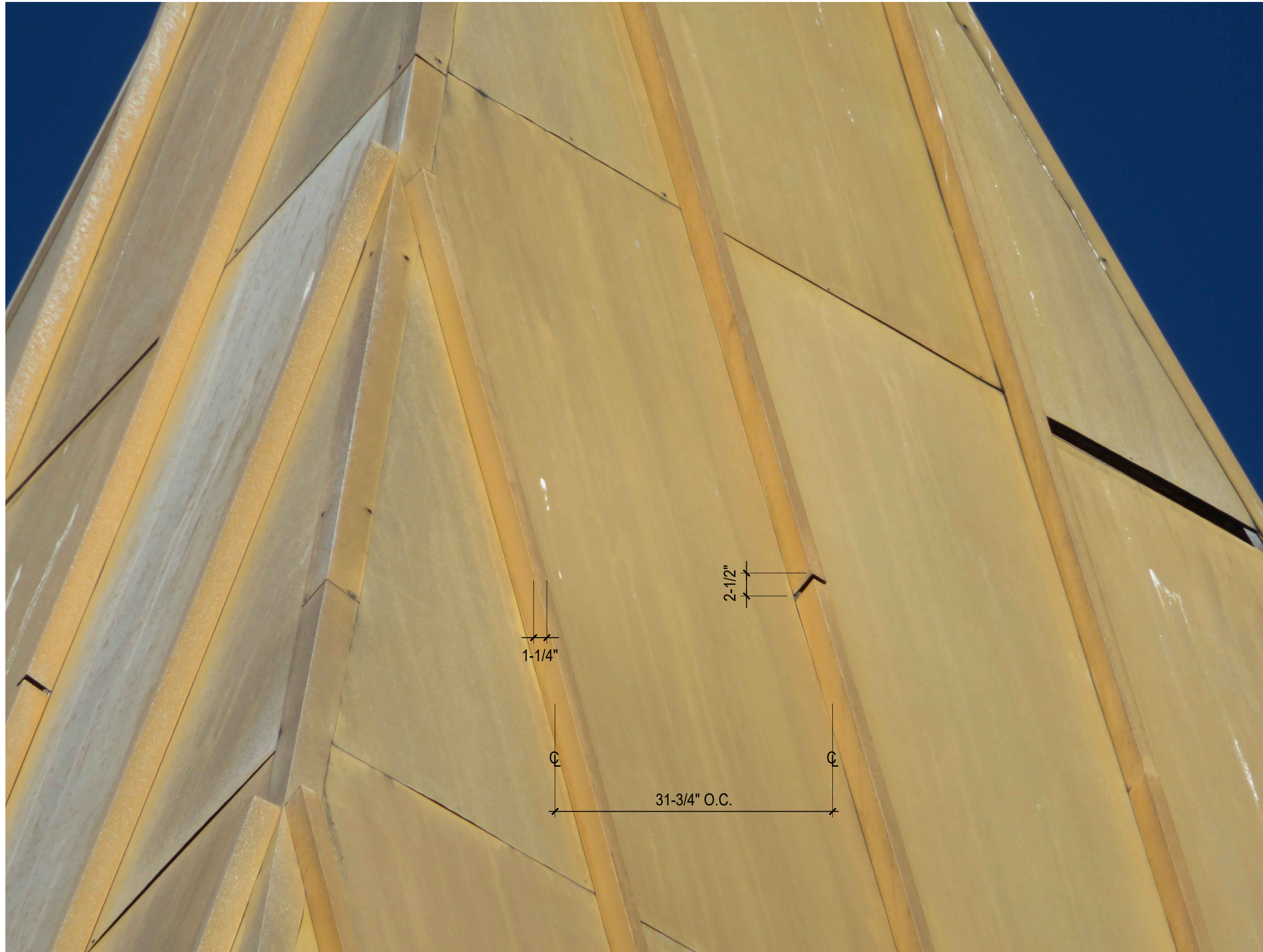
1 EXISTING SNAP-ON BATTEN METAL ROOF DETAIL NOT TO SCALE IMG_6005.JPG
