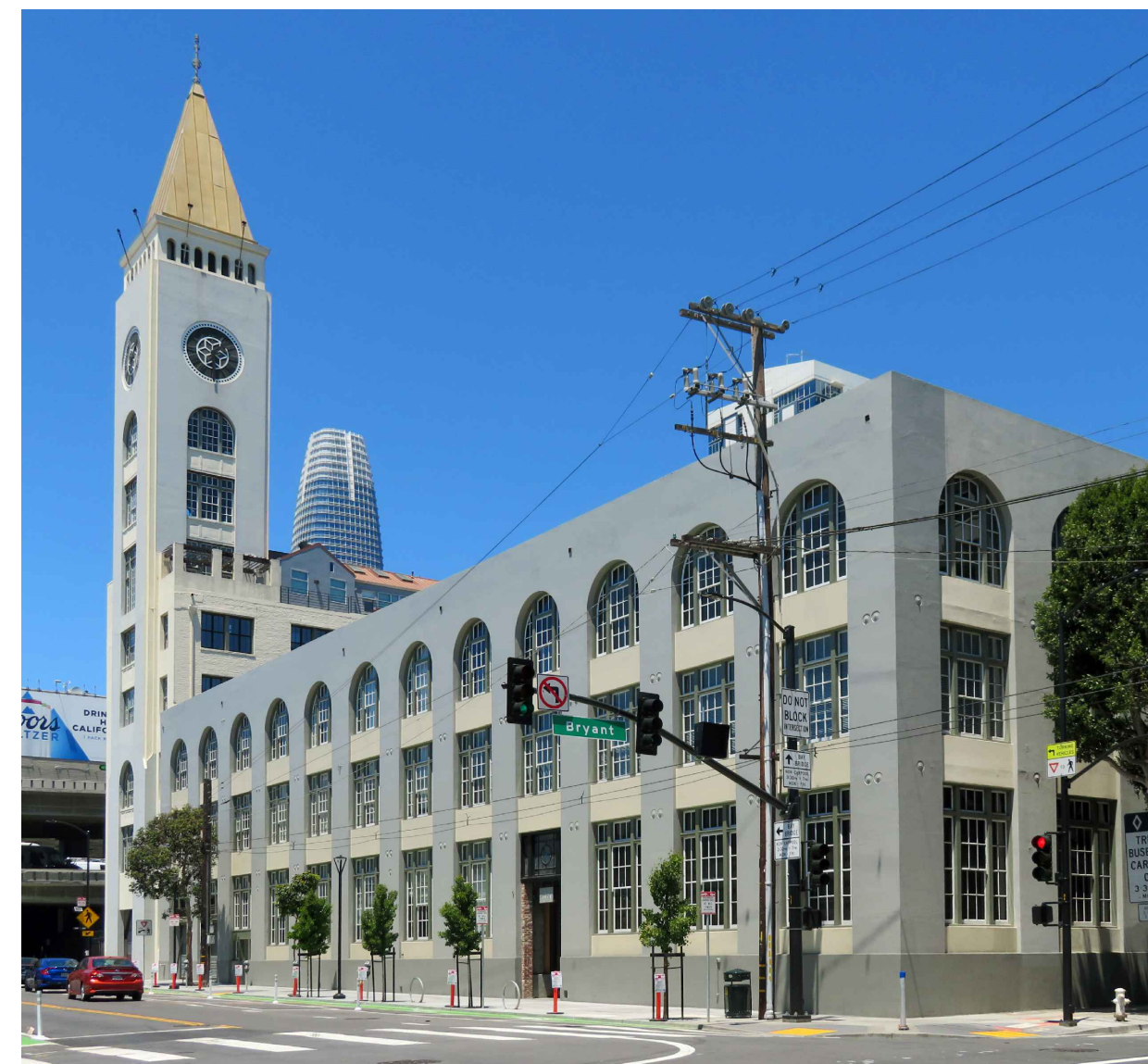
3 VIEW OF SOUTH AND WEST ELEVATIONS, 2021 PC: ARG
