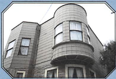
Before the Teevan Restoration
