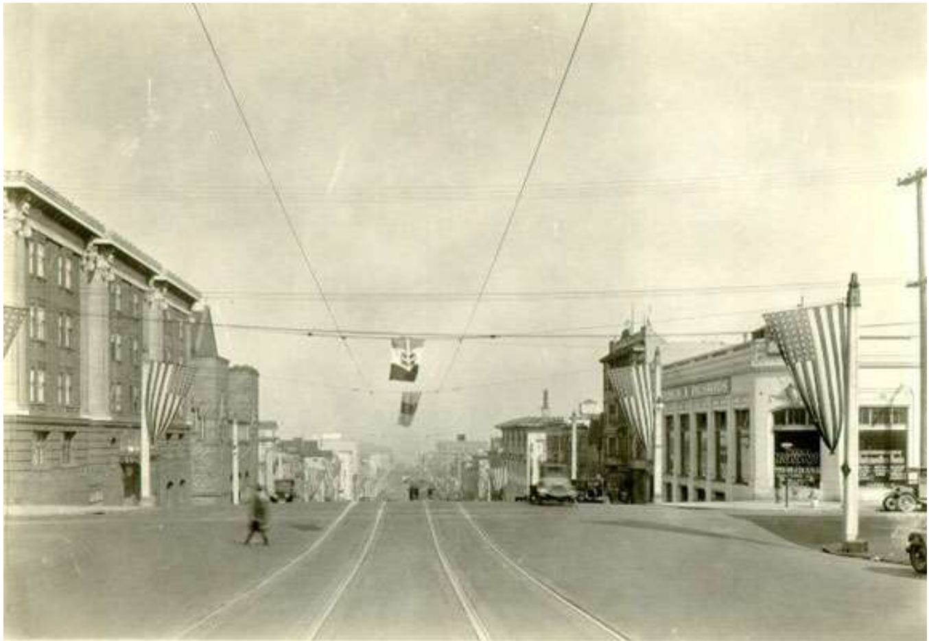
View looking north along Van Ness Avenue from Pacific, in 1926. 2100 Van Ness is at far right. In this photo, the chamfered corner is flat (and thus lacks the three-sided entrance pavilion that has since been added). This corner appears to be devoted to a window (instead of an entrance, as at present) with a transom (since filled in), and is topped by a cartouche with swags (since removed). Transoms can be found at the top of the other window openings as well (these have also since been filled in). The cornice and parapet in this photo seem to be the same as at present. From the San Francisco Public Library, photo AAB-5680.
