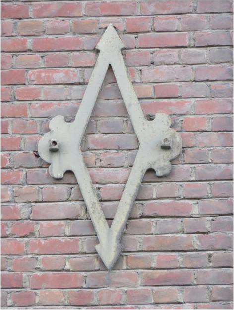
1912 brick building, detail of a diamond-shaped wall anchor plate on the north façade (ARG, November 2019)
