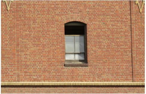
1912 brick building, detail of a two-over-two, wood-sash window on the west façade (ARG, November 2019).
