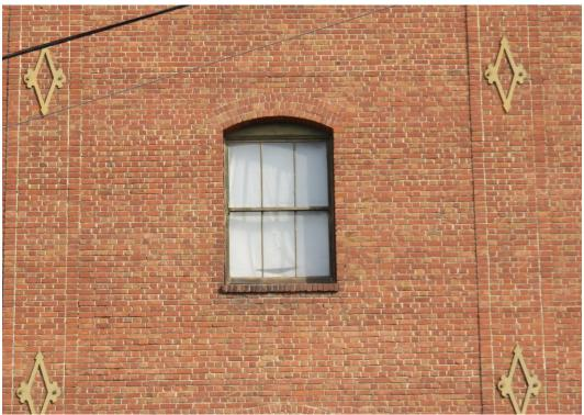
1912 brick building, detail of a three-over-three, wood-sash window on the west façade (ARG, November 2019).
