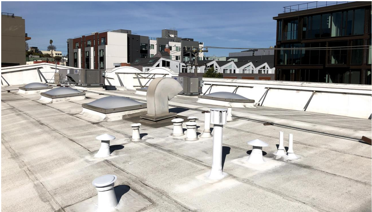
Figure 26. Detail of roof showing roof-mounted vents and mechanical equipment; view toward northwest.
