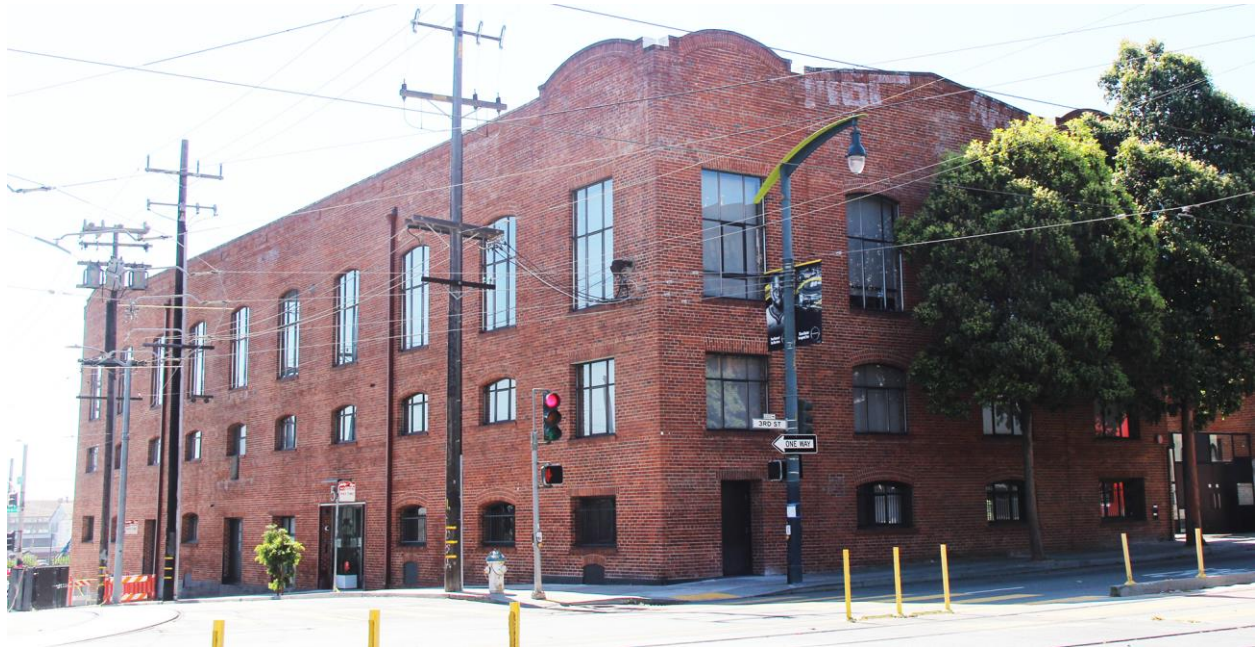
Figure 7. North (left) and west (right) façades.
