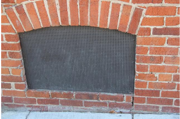
Figure 18. Typical basement window.
