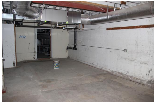
Figure 28. Basement storage room.
