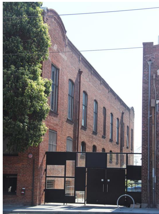
Figure 8. South façade from 3 rd Street.
