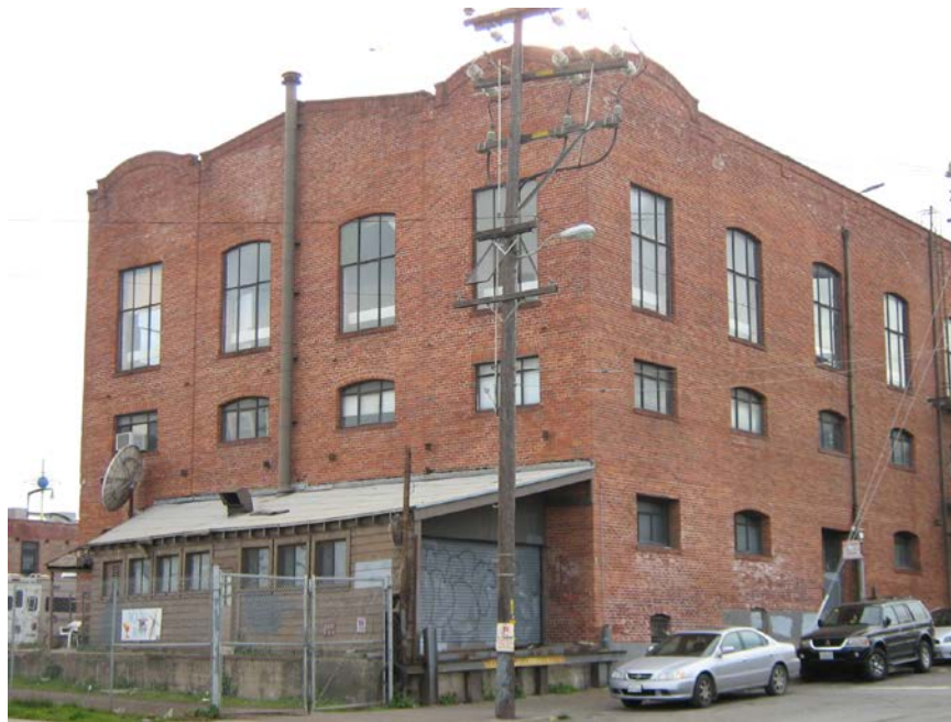
Illinois Street (east) façade with train shed (6 February 2007)
