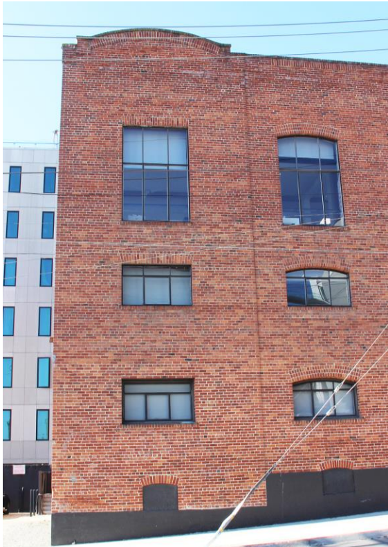
Figure 10. Corner pavilion facing 19 th Street.
