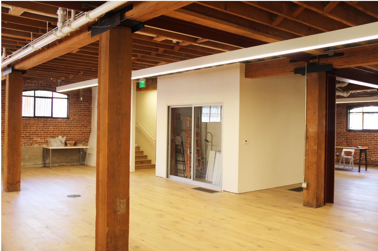
Figure 43. Heavy timber frame at first-floor level; view toward northwest.
