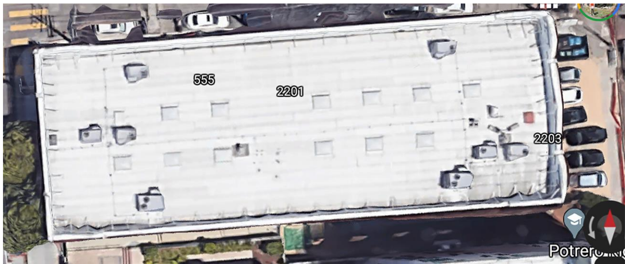
Figure 24. Roof of 555 19 th Street.
