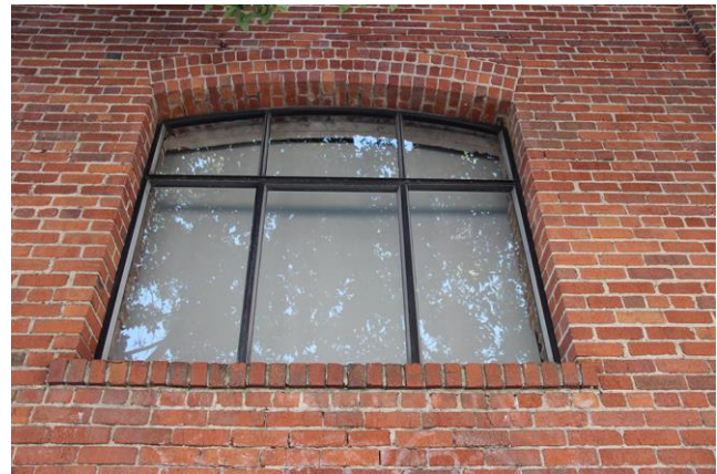
Figure 17. Typical segmental-arch window.
