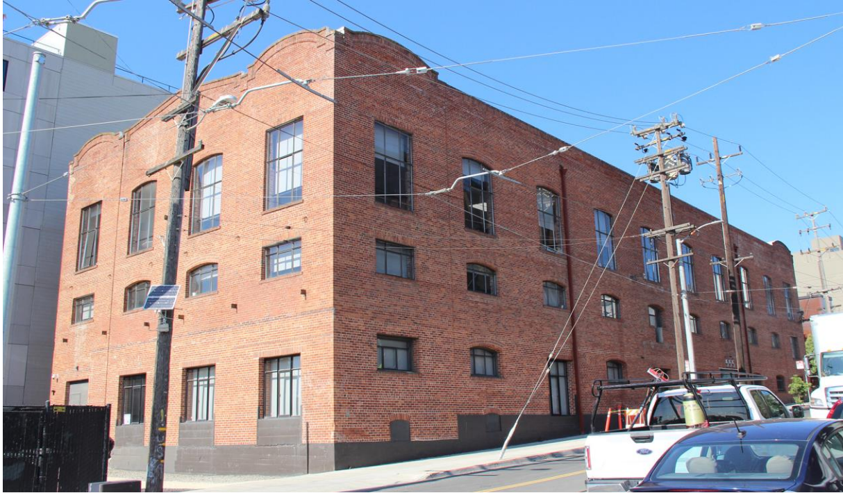
Figure 9. North (right) and east (left) façades.
