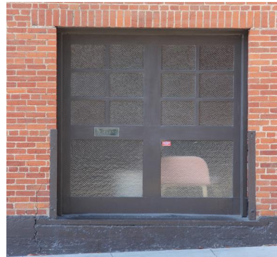
Figure 23. Freight door on 19 th Street.
