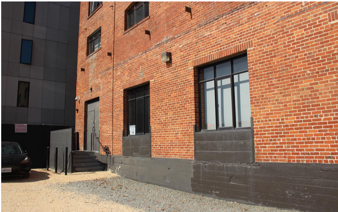
Figure 14. Concrete foundation and loading docks facing Illinois Street.
