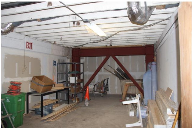
Figure 27. Basement storage room; note moment frame.
