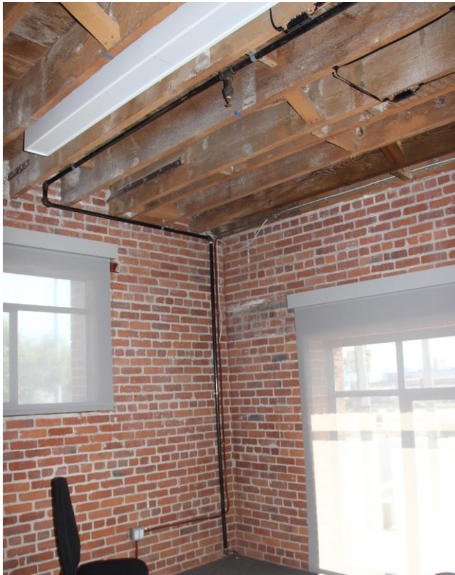
Figure 31. First-floor level; northeast corner.
