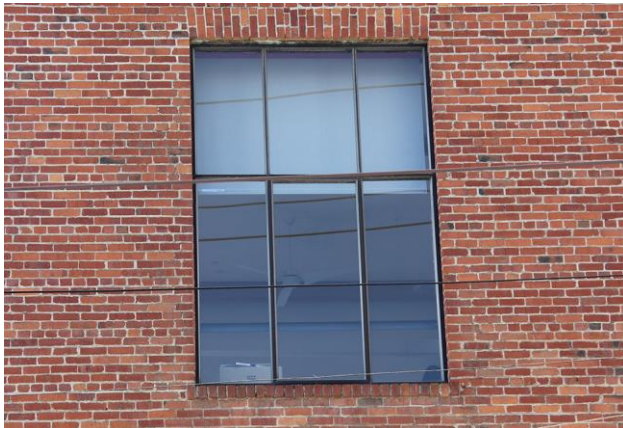
Figure 16. Typical jack-arch window.
