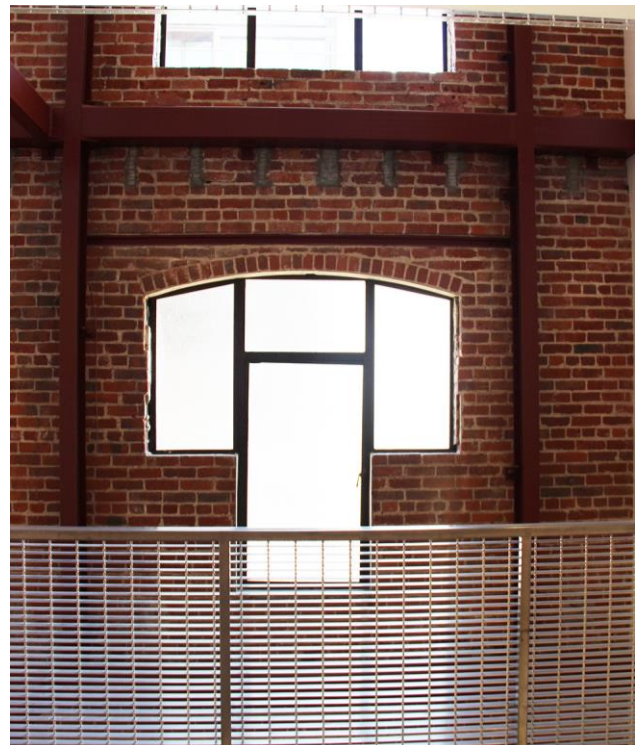
Figure 36. View of exposed brick walls and moment frame at second-floor level.
