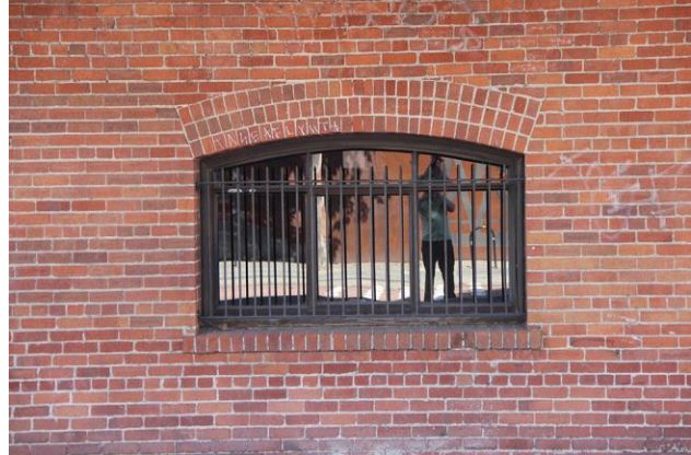
Figure 19. Typical first-floor window.
