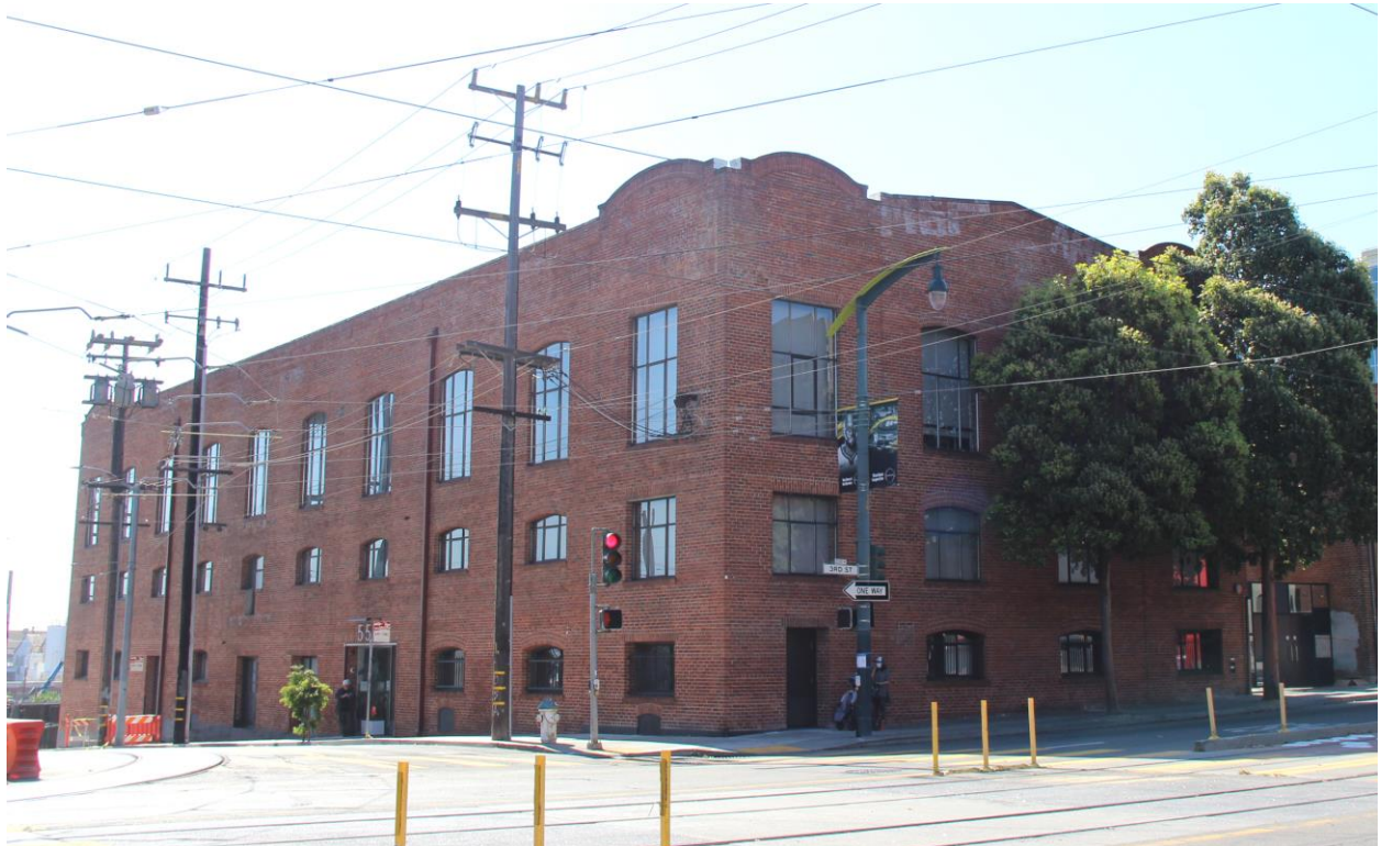
Figure 2. 555 19 th Street; view toward southeast from intersection of 3 rd and 19 th streets.
