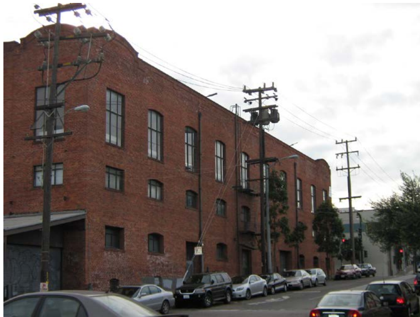
19 th Street (north) façade (6 February 2007)
