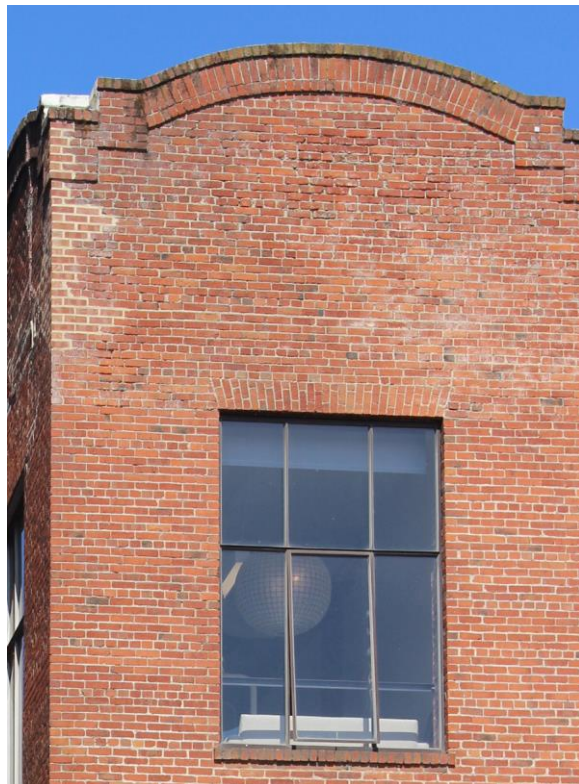
Figure 11. Detail of parapet and window opening facing Illinois Street.
