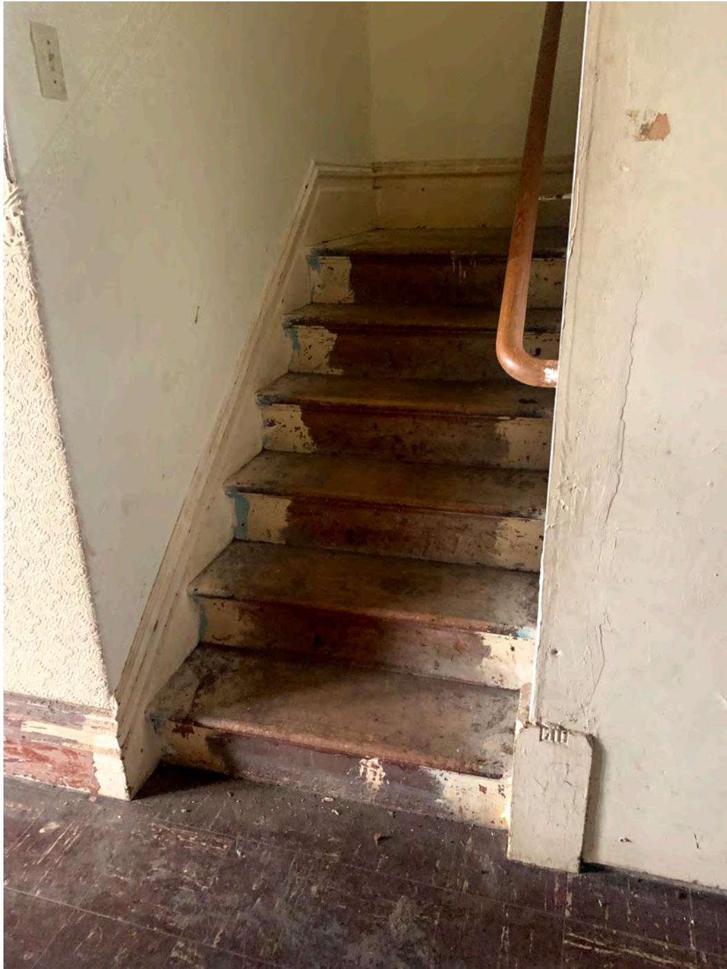
Photograph 46: Stairs to attic level
