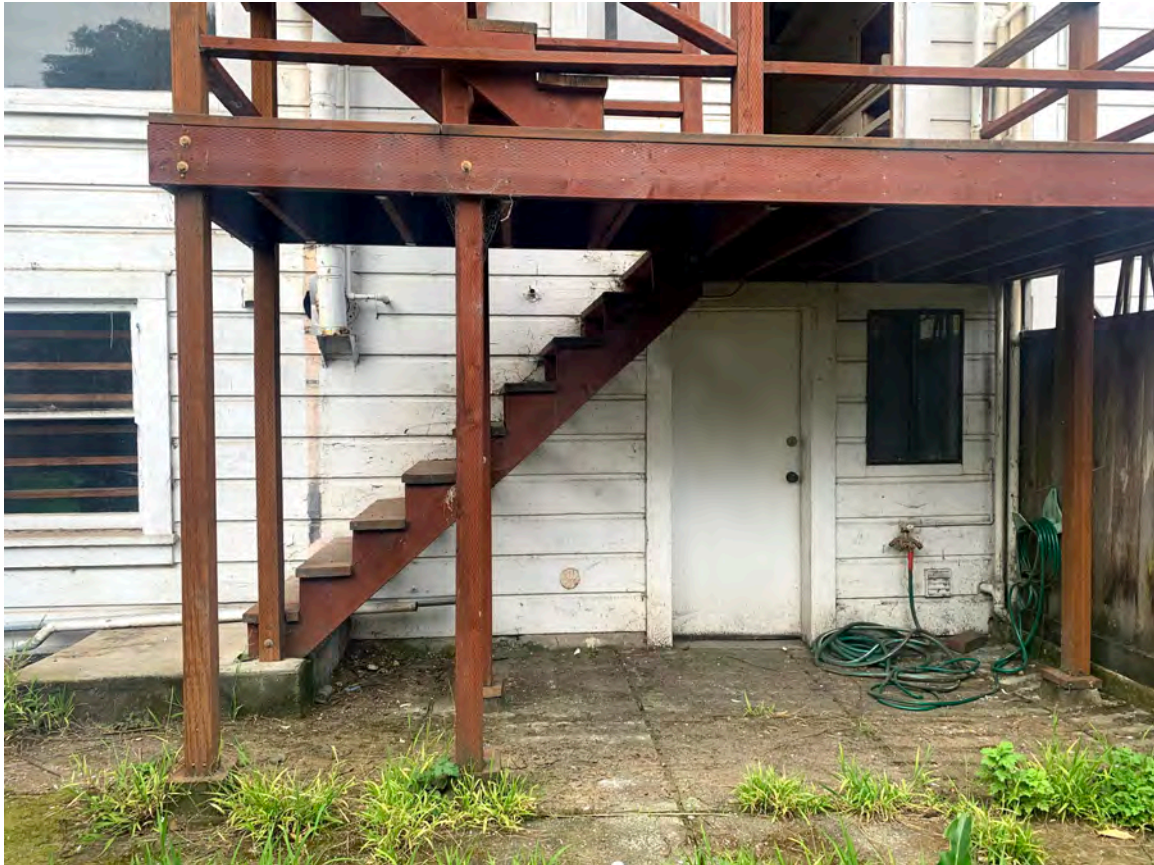
Photograph 31: Detail of rear, east façade, stairs, paved yard and secondary door.
