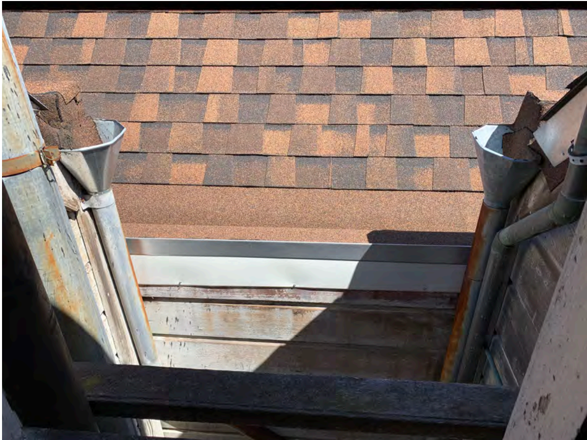
Photograph 33: Detail of light well and roof shingles
