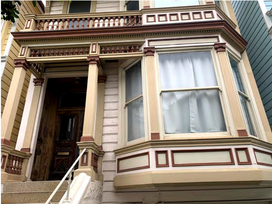
Photograph 17: 714 Steiner, primary Steiner Street façade, detail of porch and bay window
