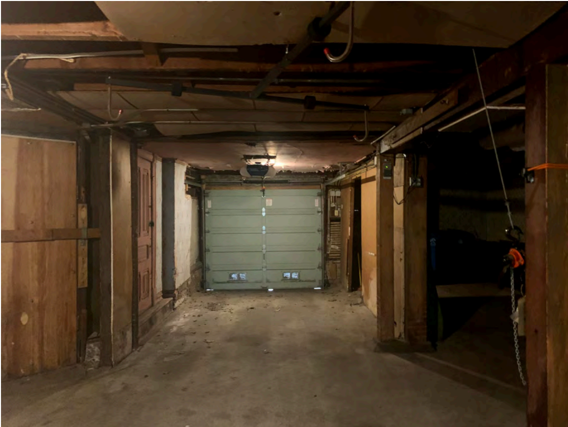
Photograph 51: Garage showing inserted door
