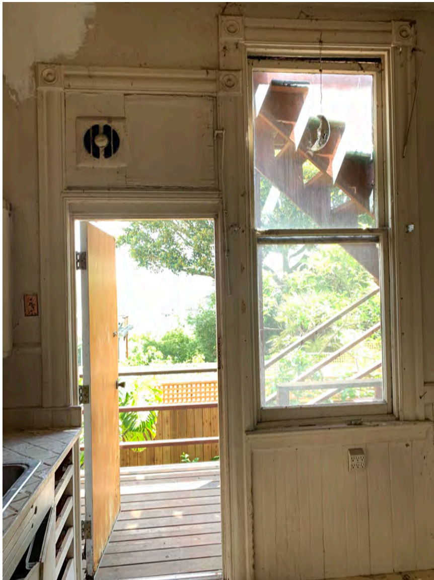
Photograph 40: Rear door at kitchen first floor
