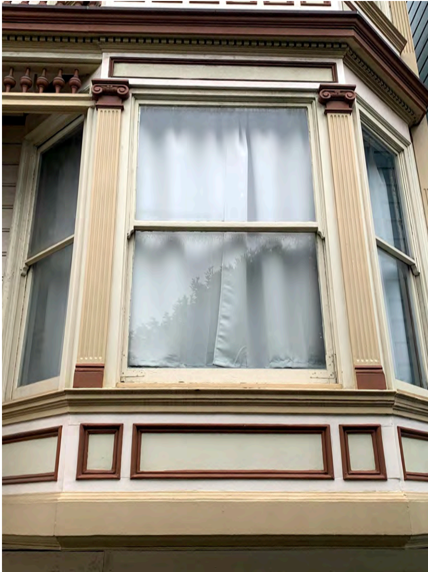
Photograph 18: 714 Steiner, primary Steiner Street façade, detail of bay window
