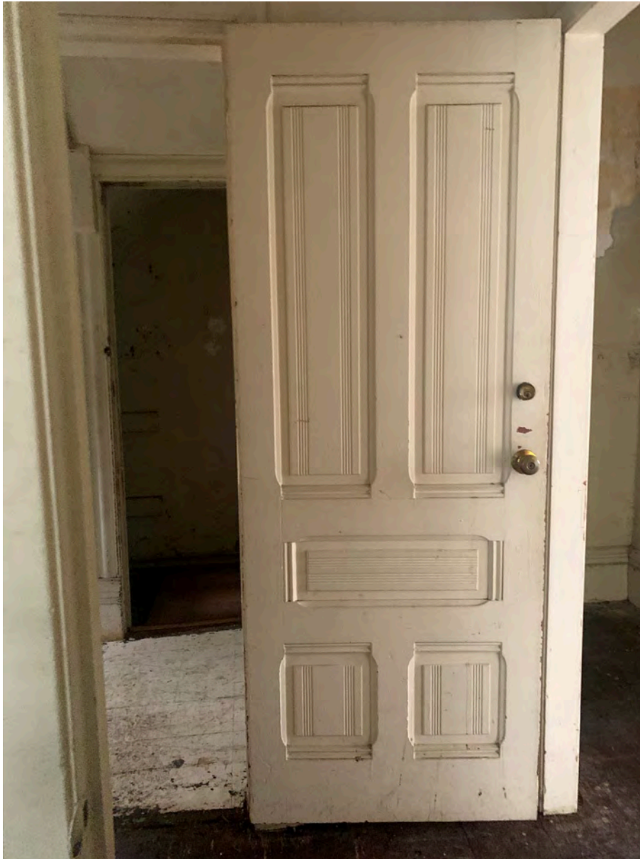
Photograph 36 Typical door first floor hallway
