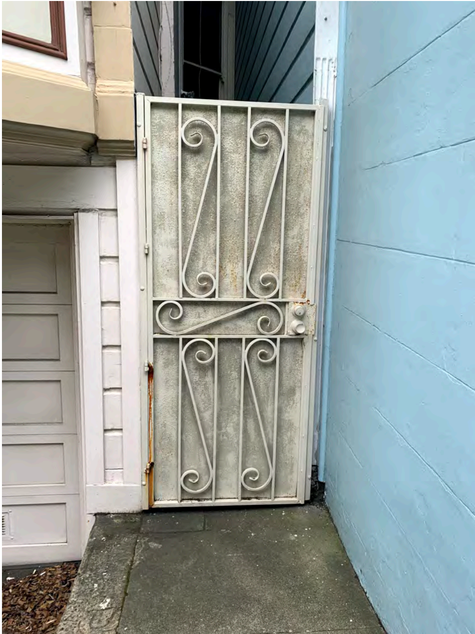
Photograph 4: 714 Steiner, primary Steiner Street façade, detail of side walkway access gate
