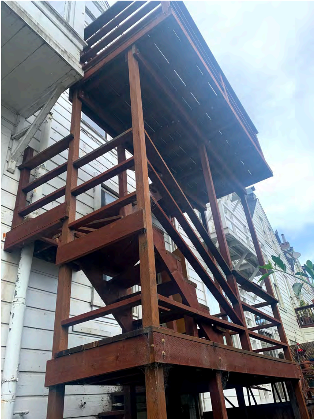
Photograph 30: Detail of rear, east façade, stairs to upper level deck
