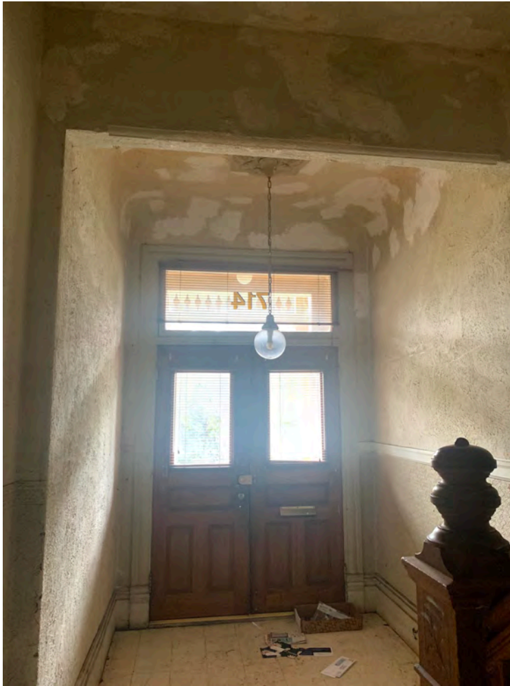
Photograph 35: View of entry hall looking toward front door
