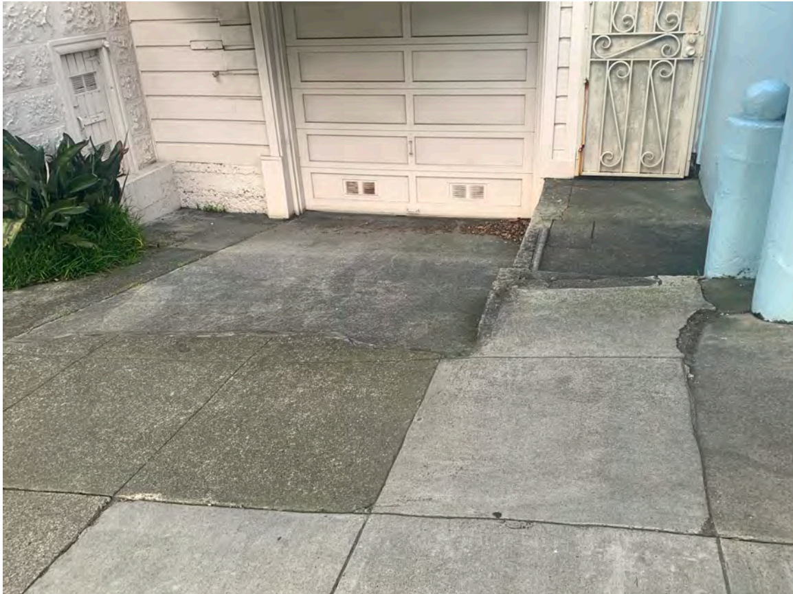
Photograph 5: 714 Steiner, primary Steiner Street façade, detail of driveway
