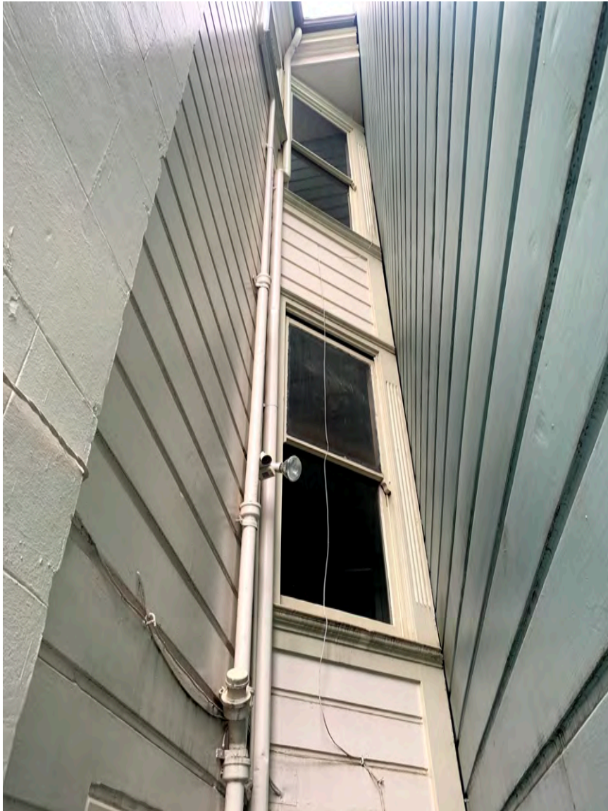
Photograph 24: 714 Steiner, south façade, detail of windows.
