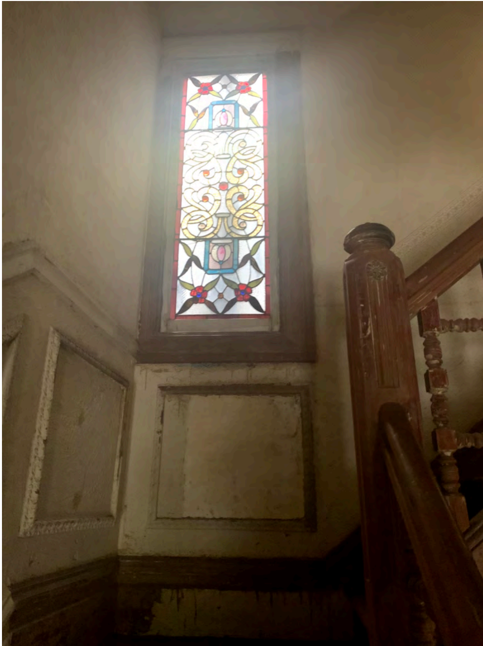
Photograph 37: Stair landing and stained glass window
