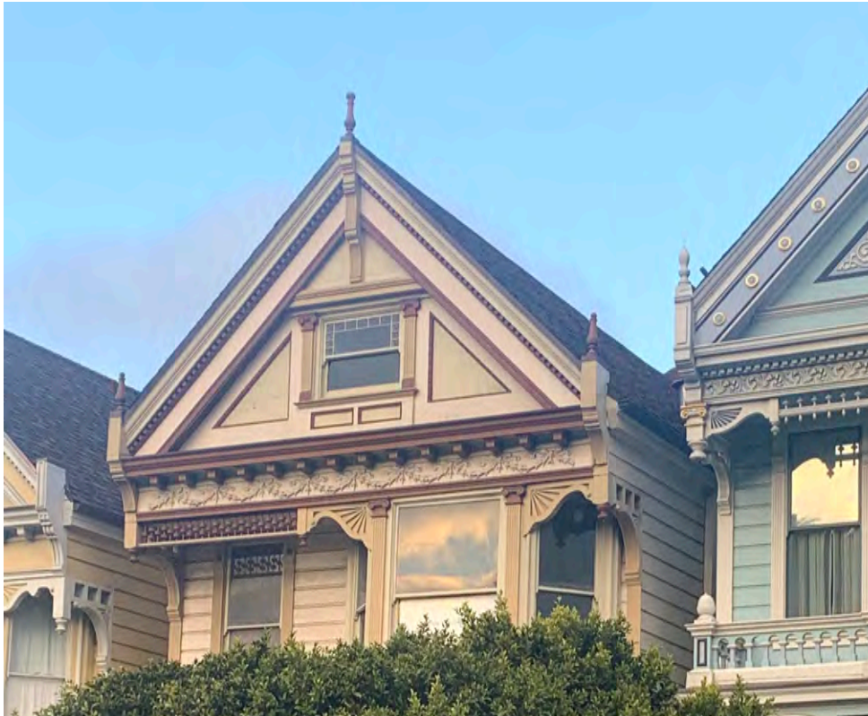
Photograph 19: 714 Steiner, primary Steiner Street façade, detail of upper story
