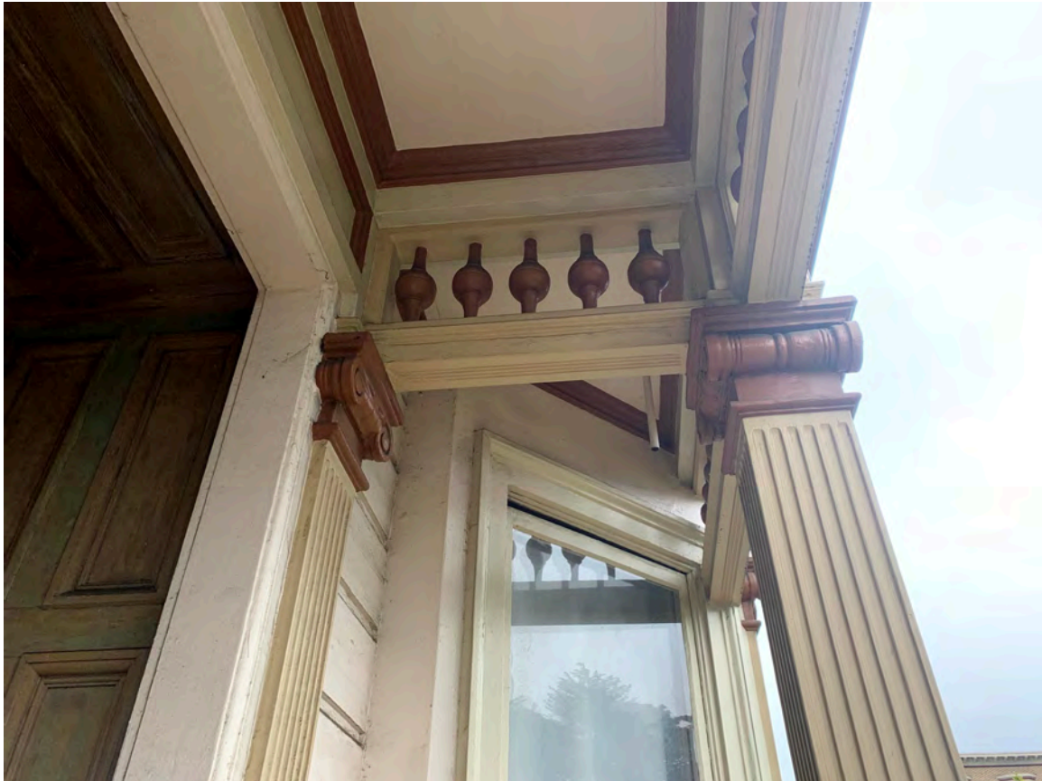
Photograph 15: 714 Steiner, primary Steiner Street façade, detail of porch posts, engaged pilasters and capitals
