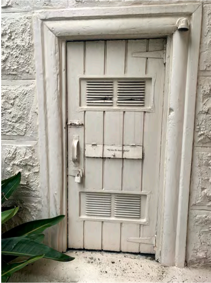
Photograph 7: 714 Steiner, primary Steiner Street façade, close up detail of under-stair door
