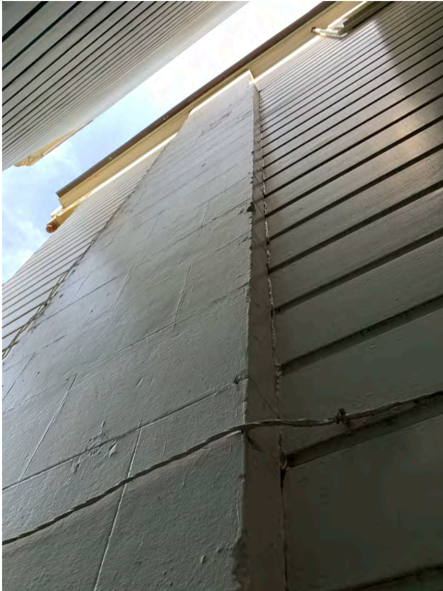
Photograph 25: 714 Steiner, south façade, detail of brick chimney with stucco scoring.
