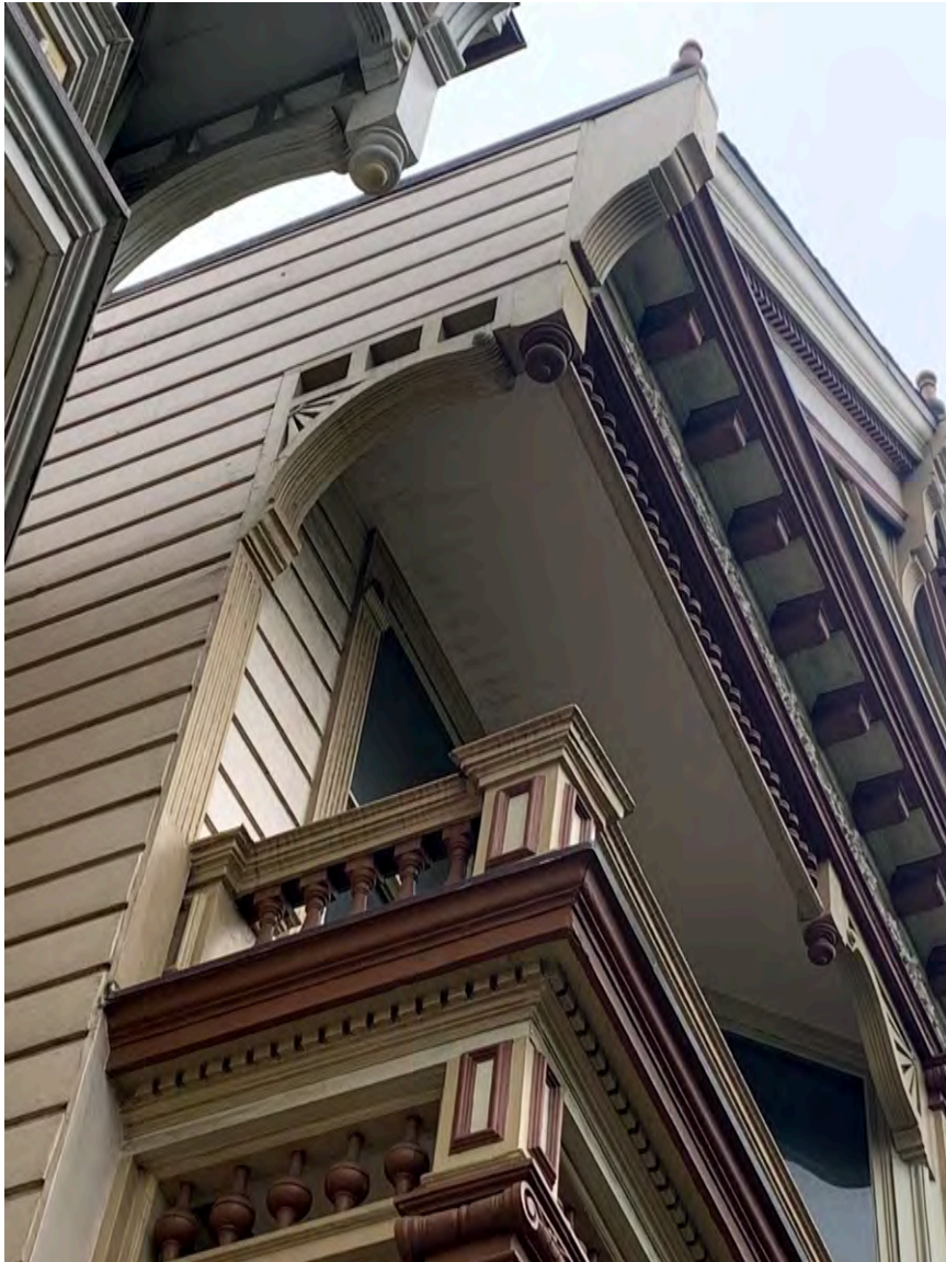
Photograph 22: 714 Steiner, primary Steiner Street façade, detail of balcony above porch
