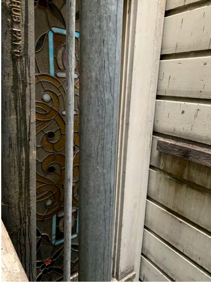
Photograph 32: Detail of lightwell at stained glass window
