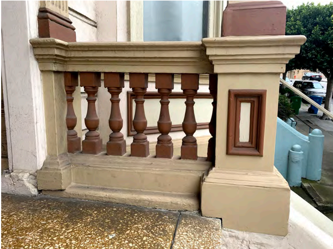
Photograph 14: 714 Steiner, primary Steiner Street façade, detail of stair landing and balustrade
