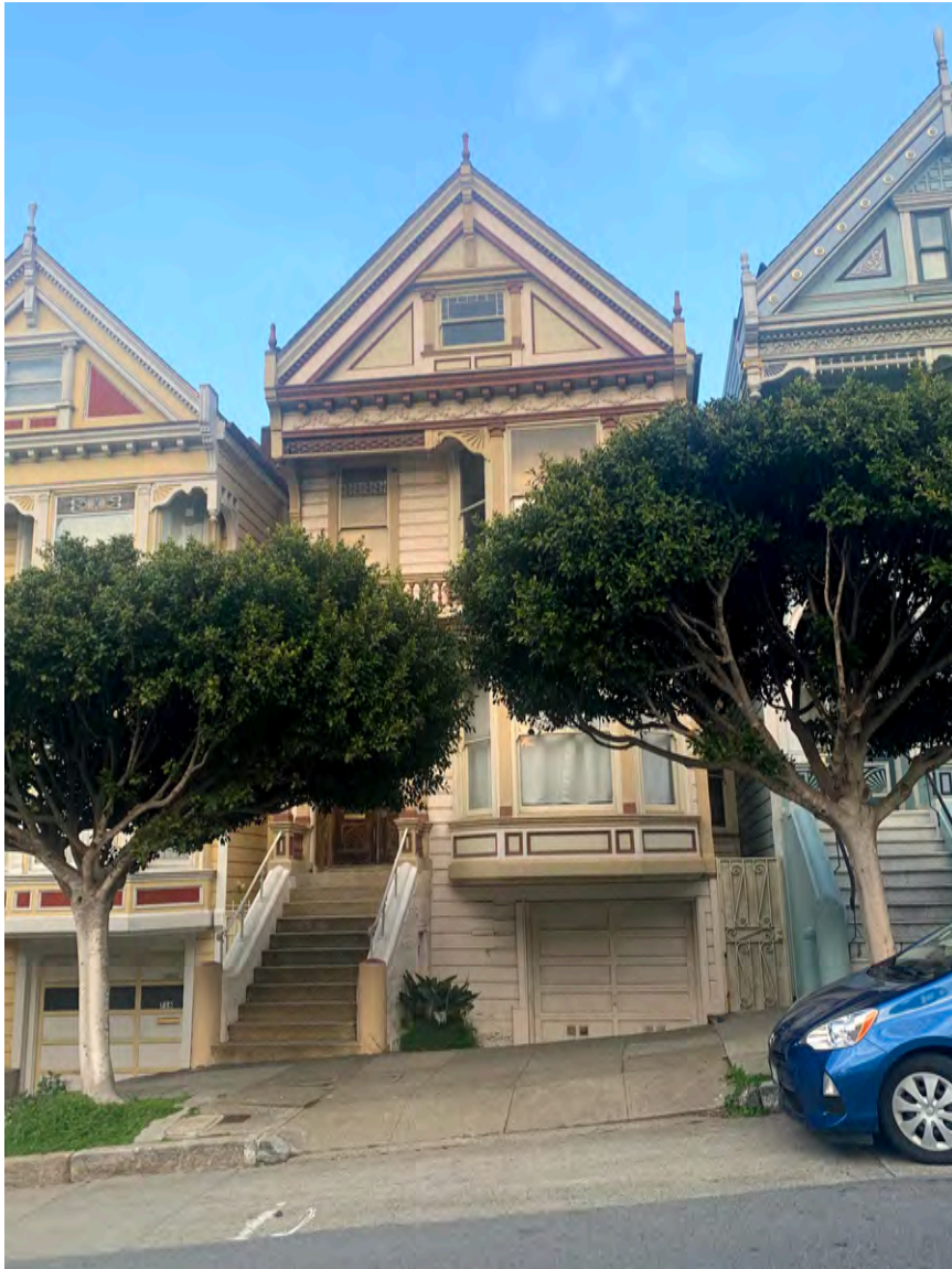
Photograph 2: 714 Steiner, primary Steiner Street façade, overview with street trees.
