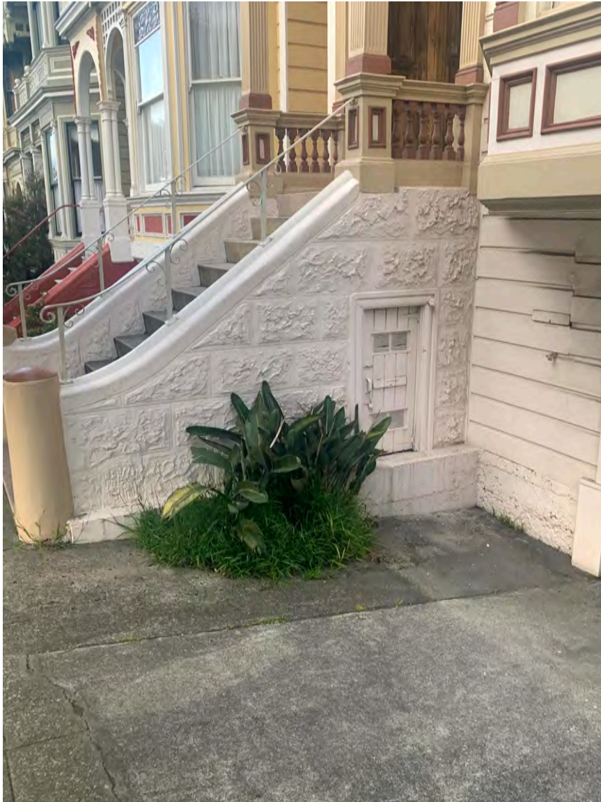
Photograph 6: 714 Steiner, primary Steiner Street façade, detail of under-stair door
