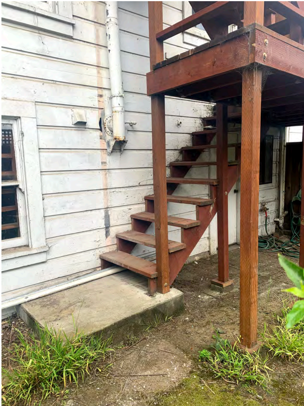
Photograph 29: Detail of rear, east façade, stair and secondary door underneath.
