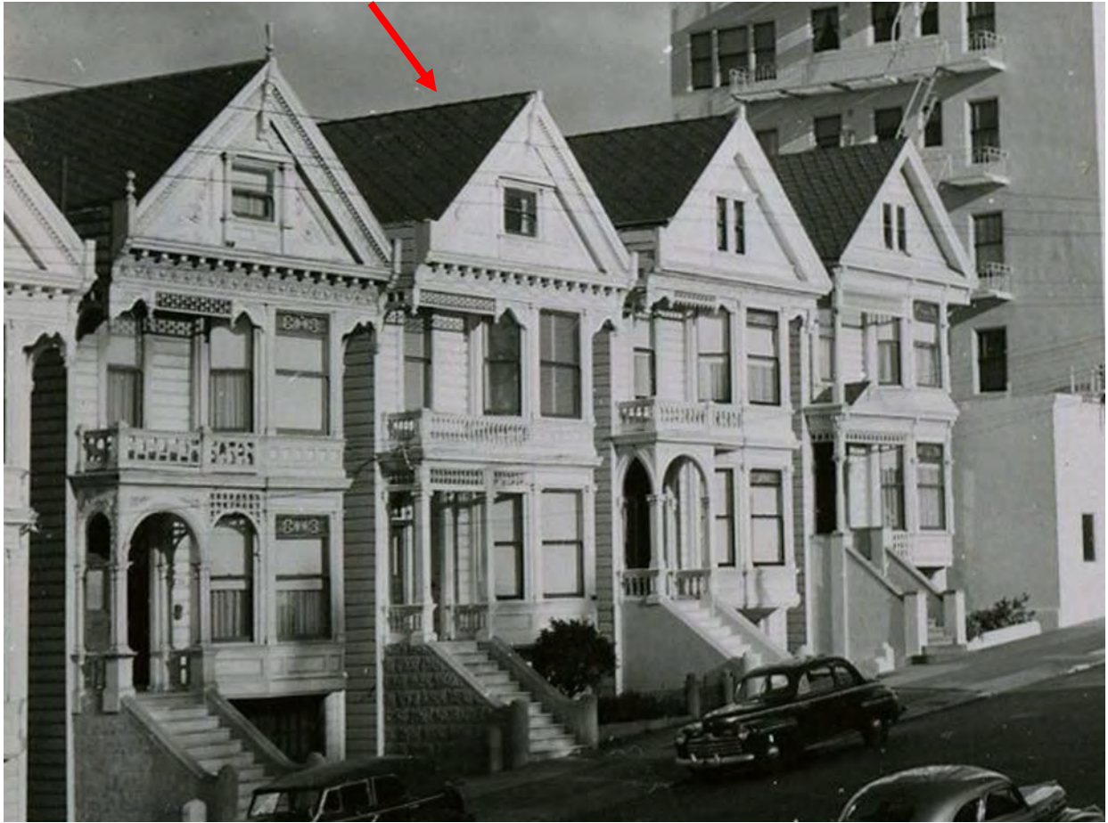
Historic Photograph 6: Detail of historic photograph 5. The low wall, gate and landscaping in front of 714 Steiner Street, including the bollards. Source: Owner, 712 Steiner Street.
