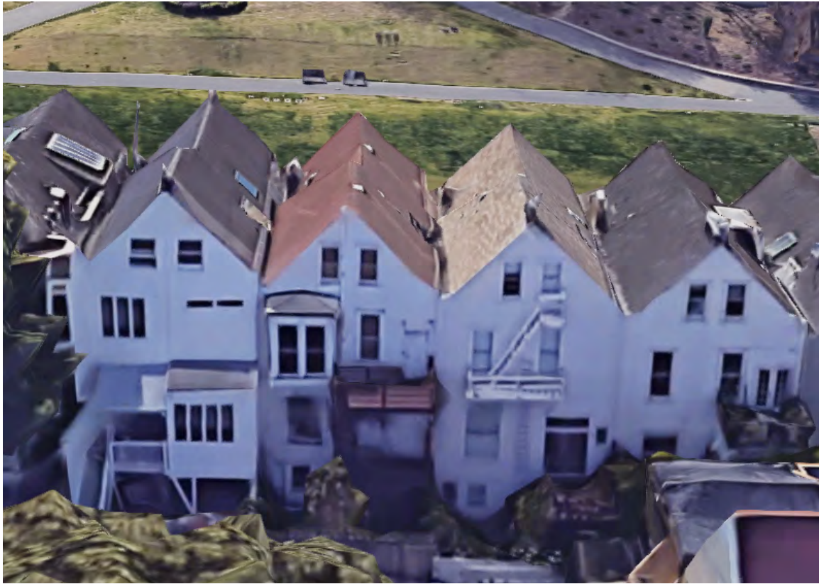
Photograph 26: Aerial photograph showing of rear, east façade with project box bay and porch
