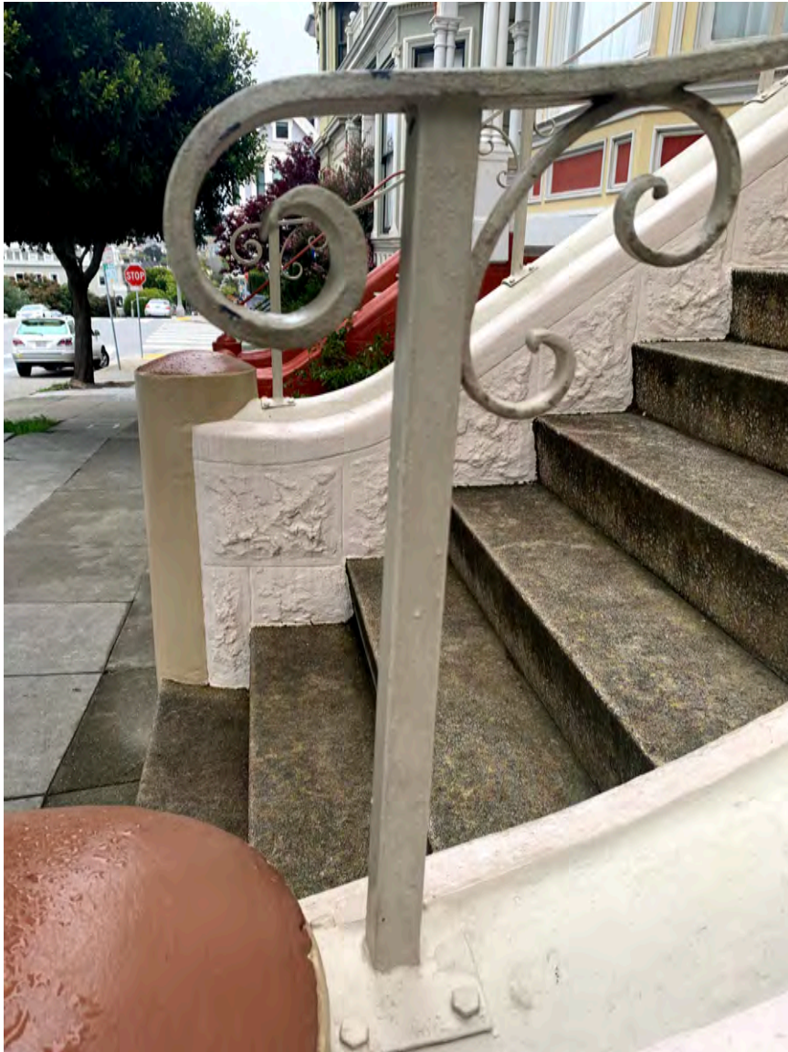
Photograph 12: 714 Steiner, primary Steiner Street façade, detail of stair railing
