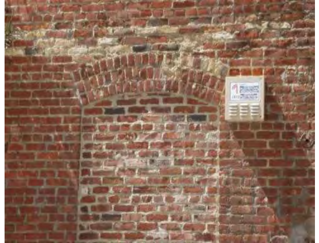
Figure 16. Close-up view of filled-in brick doorway.
