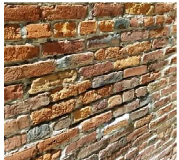
Figure 10. Close-up of brick and grout variation.
