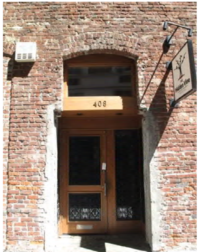
Figure 18. Rear/side (south) façade widened doorway.
