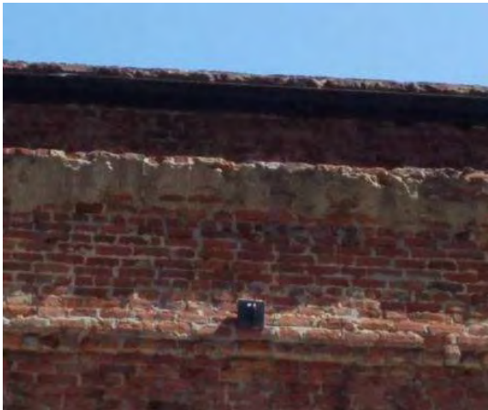
Figure 36. Close-up of patched bricks at belt course where cornice was damaged.
