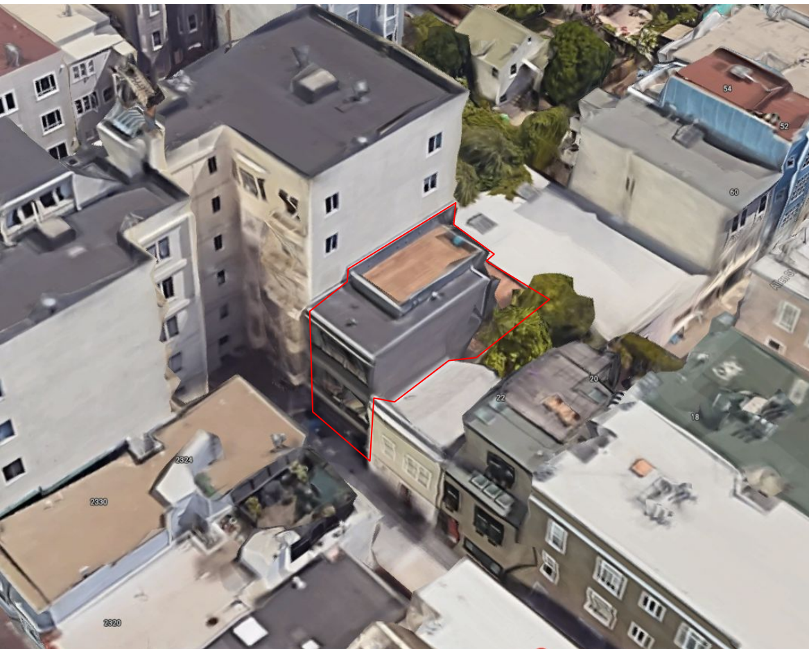
22 Moore Place - Aerial View
