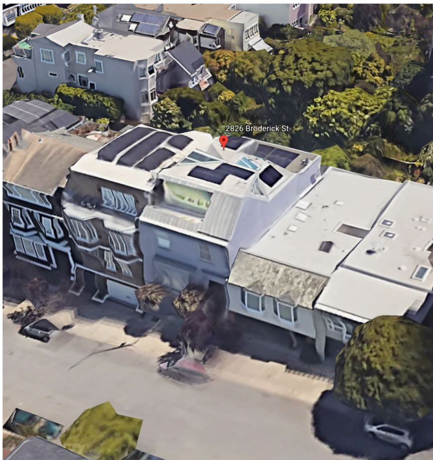
2826 Broderick Aerial View
