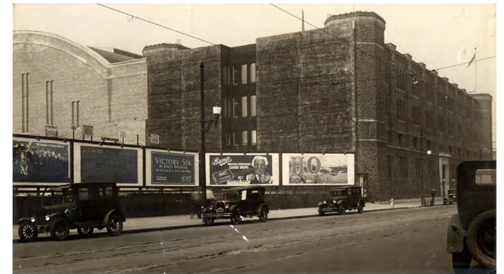
LEFT: View from Mission Street, c. 1970s TOP: View from Mission & 14th Street, c. 1970s BOTTOM: View from 15th Street, 1928 IMAGE SOURCE: www.sfpl.org
