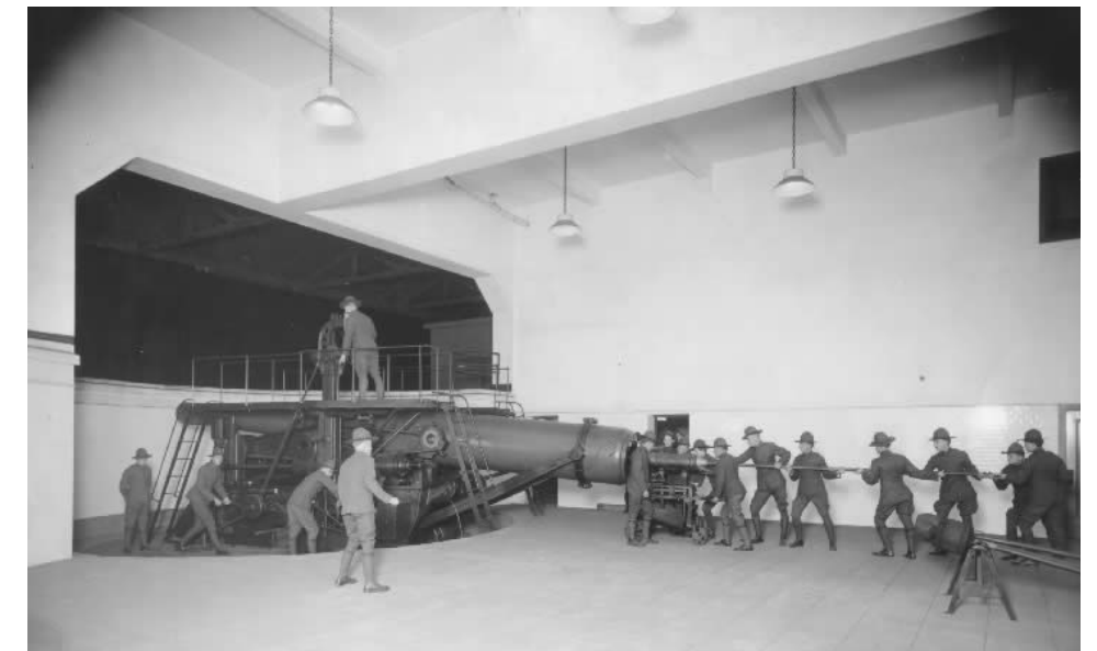
TOP: Rendering of State Armory San Francisco BOTTOM: 250th Coast Artillery Loading a Gun, 1934 IMAGE SOURCE: www.sfarmory.com
