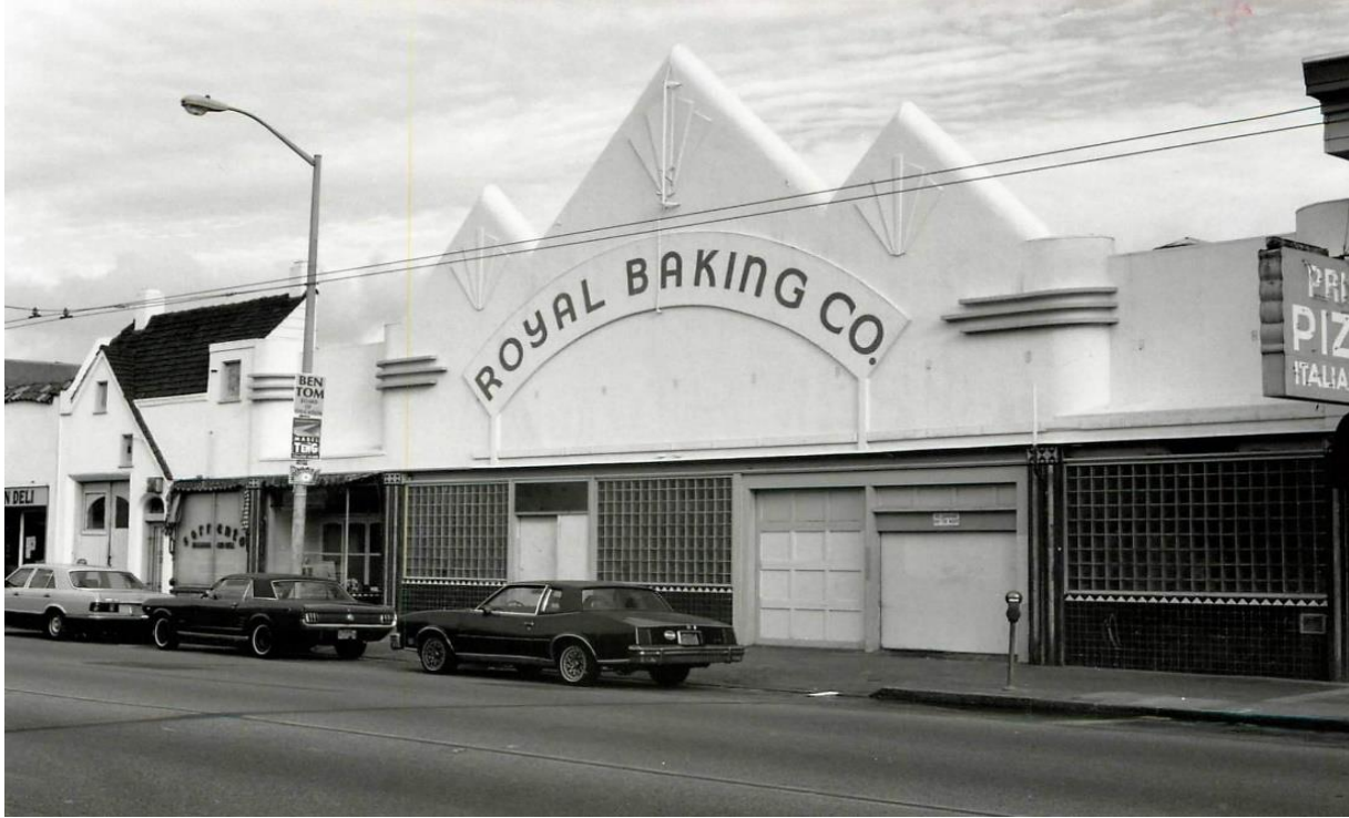
4769-4773 Mission Street, November 1990. Source: San Francisco Heritage.
