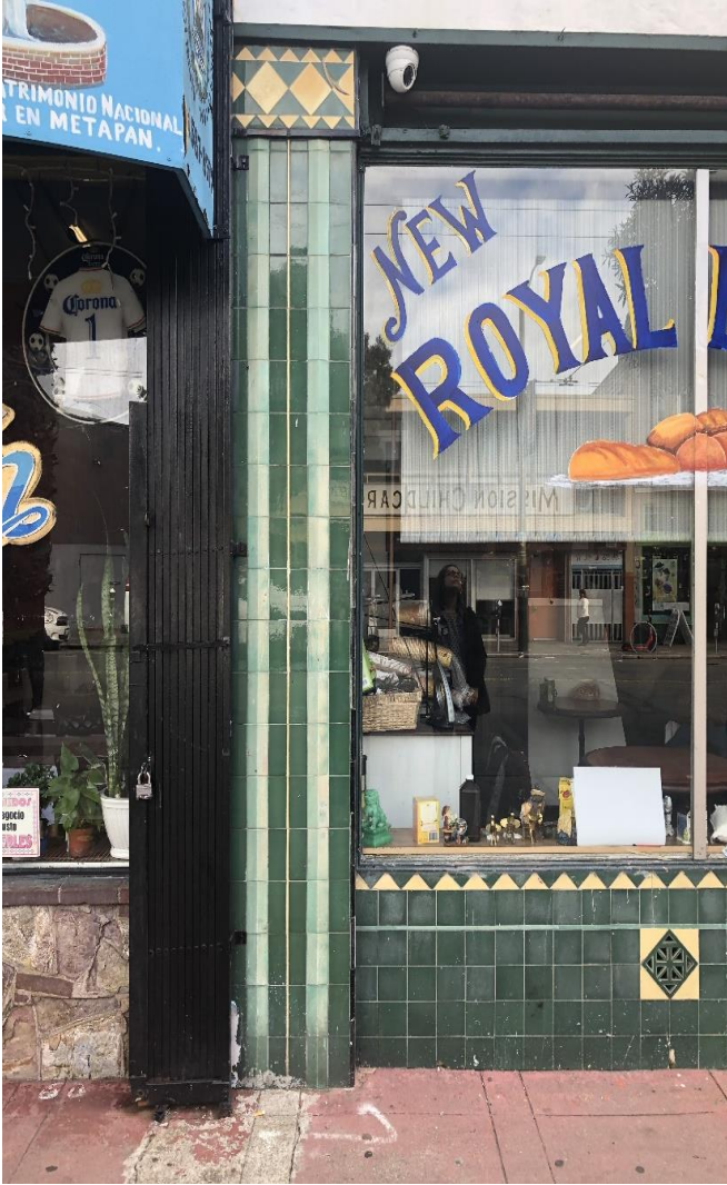
Original ceramic tile pier, bulkhead, and storefront glazing at 4773 Mission Street, January 2020.
