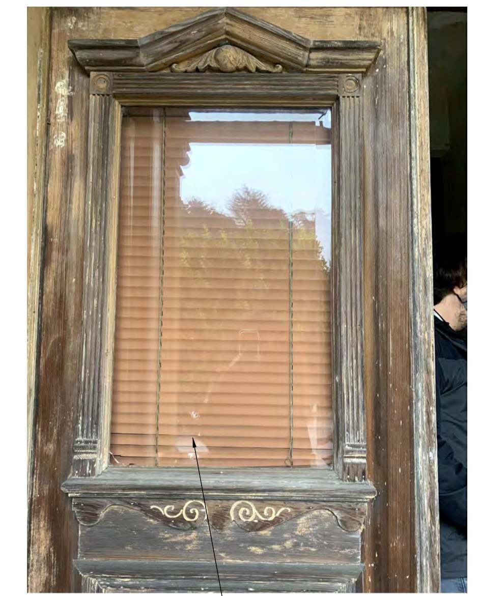
BROKEN BEVELED GLAZING FIG. 1: FRONT DOOR
