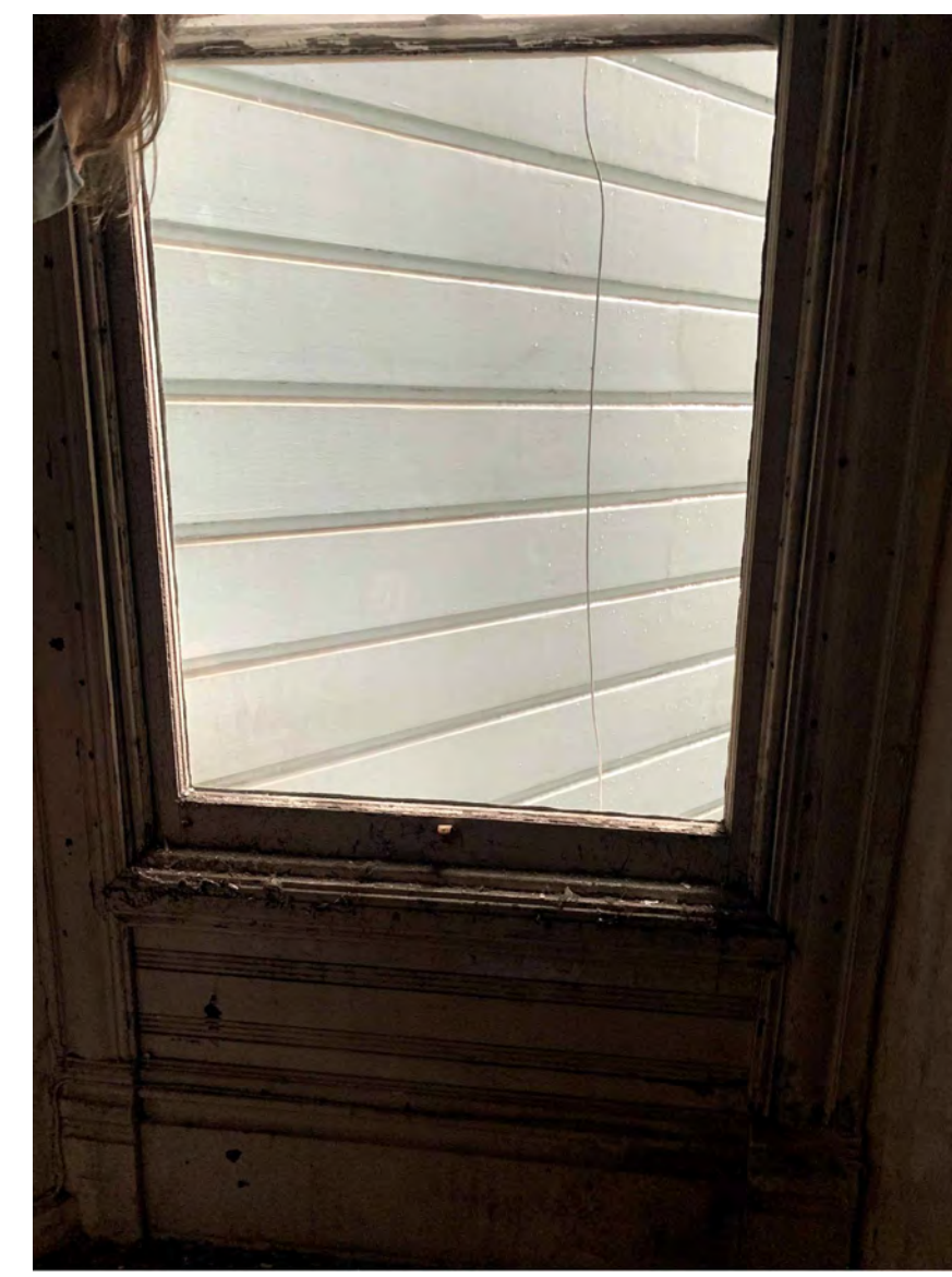
CORNER CUT OUT OF WINDOW RAIL AND BOTTOM SASH
