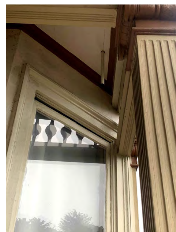
FIG. 2: EXISTING PORCH ROOF DRAIN PIPE
