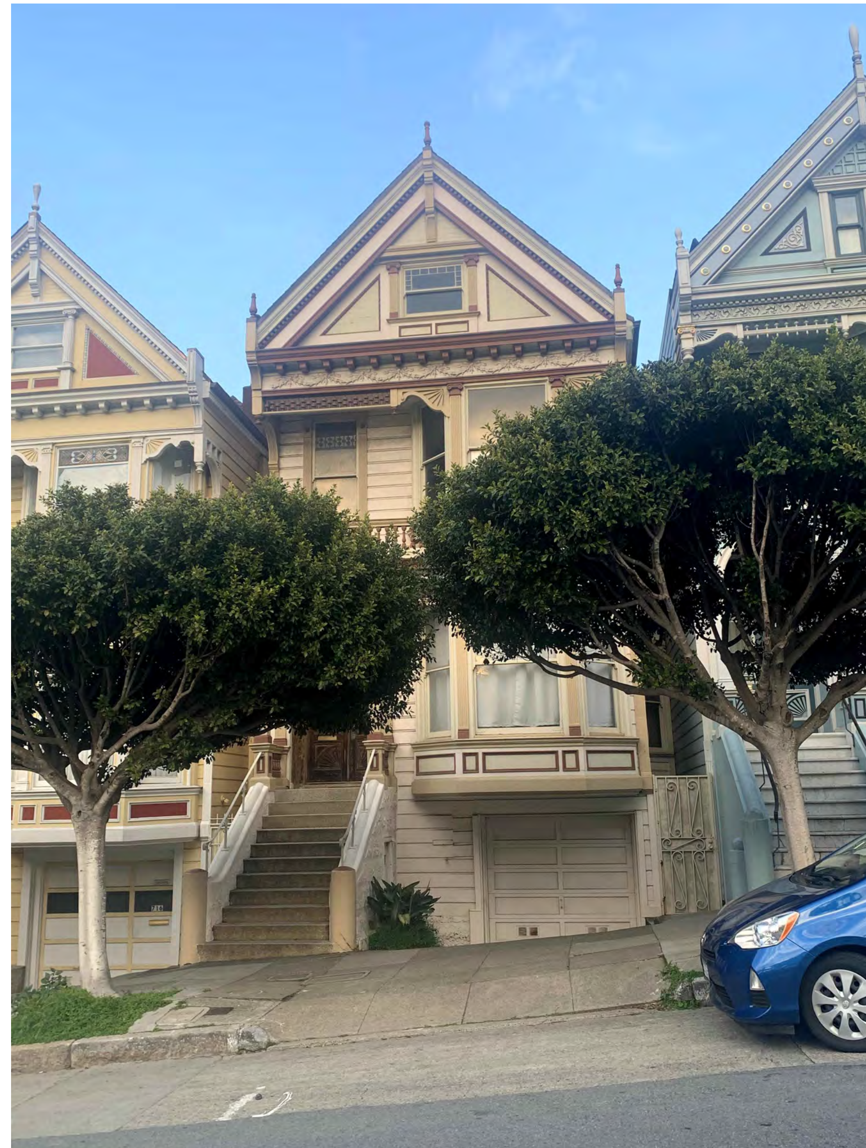
714 STEINER STREET FRONT FACADE 7
