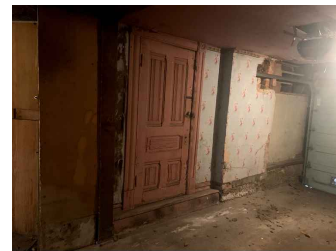
FIG. 1: EXISTING DOOR IN GARAGE COVERED BY SIDING
