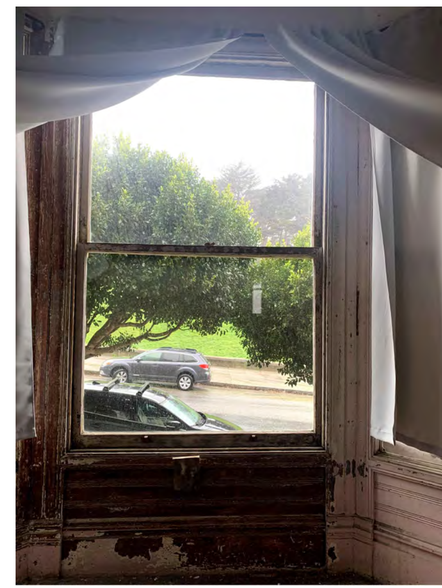
FIG. 3: WINDOWS WITH TYPICAL INTERIOR SASH CONDITIONS SUCH AS WATER DAMAGE
