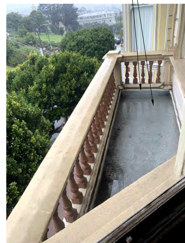
FIG. 1: EXISTING SHEET METAL ROOFING
