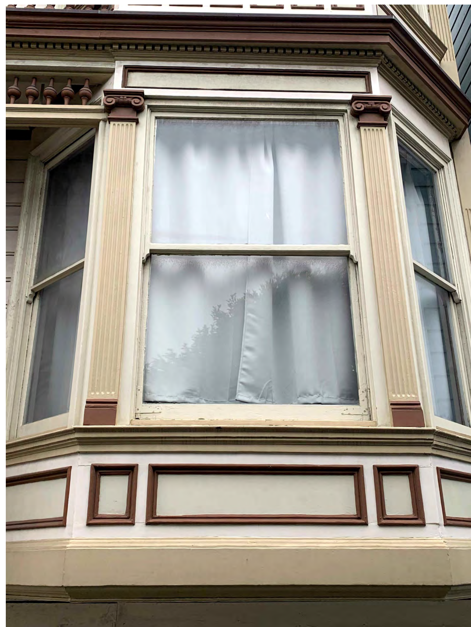
EXISTING FRONT BAY WINDOW SASH 2
