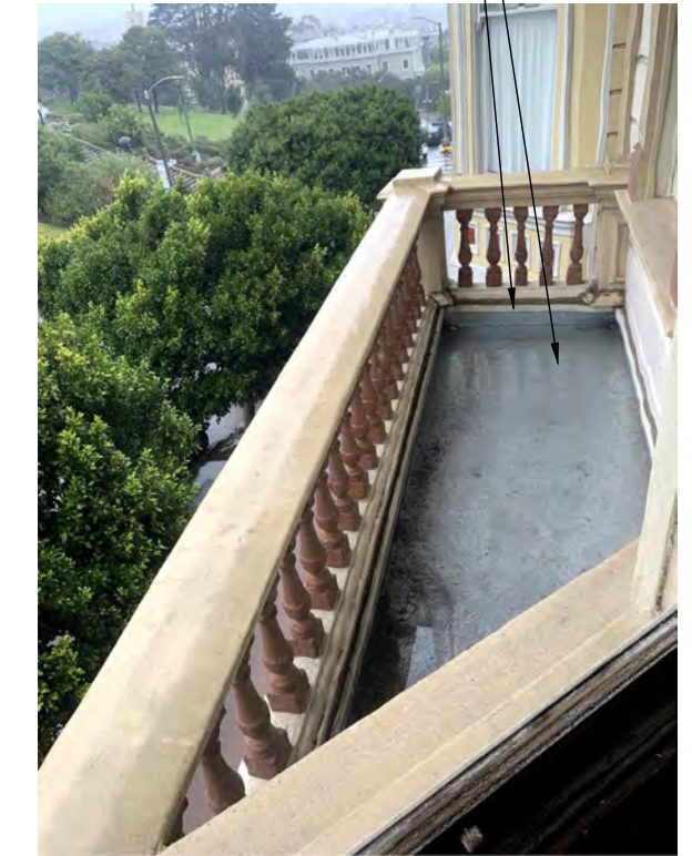
FIG. 1: EXISTING SHEET METAL ROOFING
