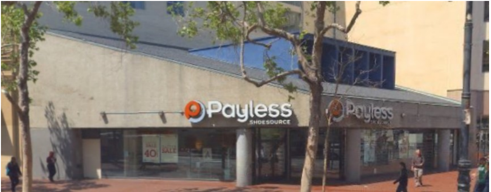
*Market Street (southern) and Cyril Magnin Street (eastern) facades viewed looking northwest from Market Street.
