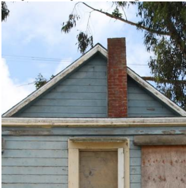
Masonry chimney stack alongside rear gable
