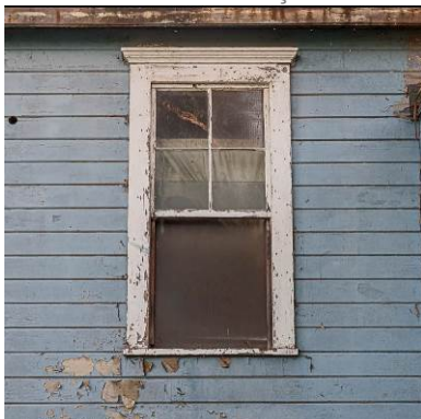
Molded window trim at secondary façades: central window at northwest façade; two windows at southeast façade
