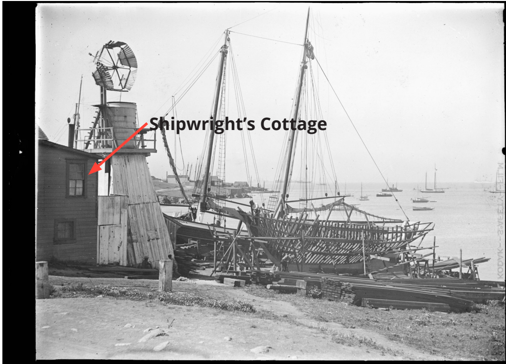
Snark (built 1907; schooner, 2m; yacht), under construction at Anderson & Cristofani's yard, scow schooner Matilda in background, San Francisco, Calif., ca. 1907, R. weinstein photographer, San Francisco Maritime National Historical Park, A04.16.813n (SAFR 21374).
