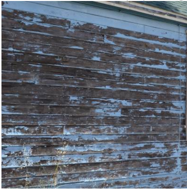
Horizontal wood shiplap siding
