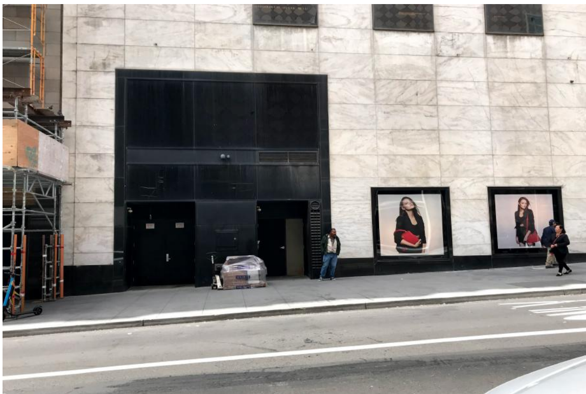
Left service entrance and two display windows, east facade.
