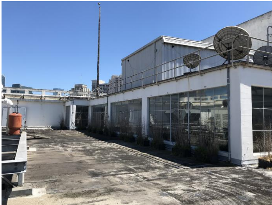
Eleventh story penthouse, looking southeast. (Property owner)
