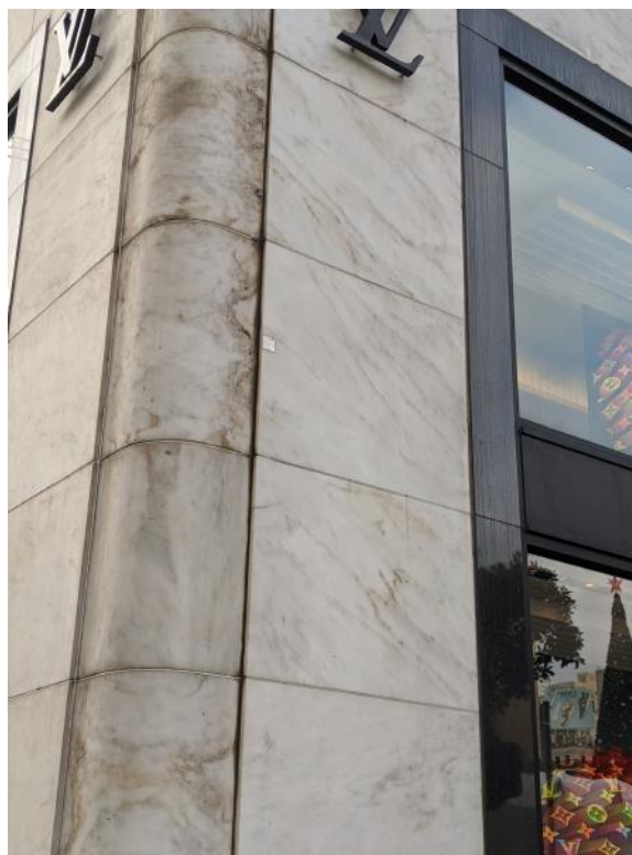
Detail of rounded northeast corner.
