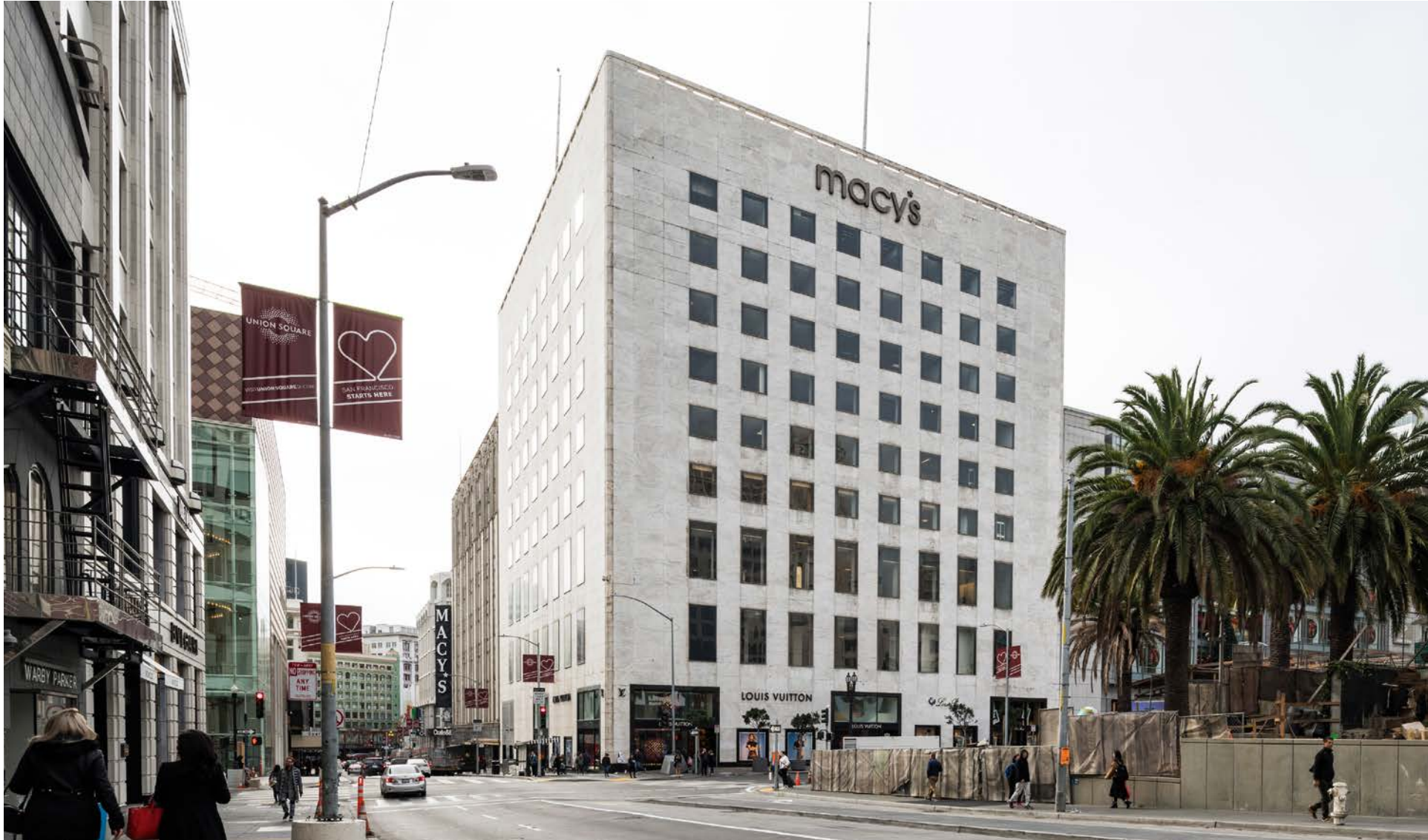
View 1: From Stockton looking south
