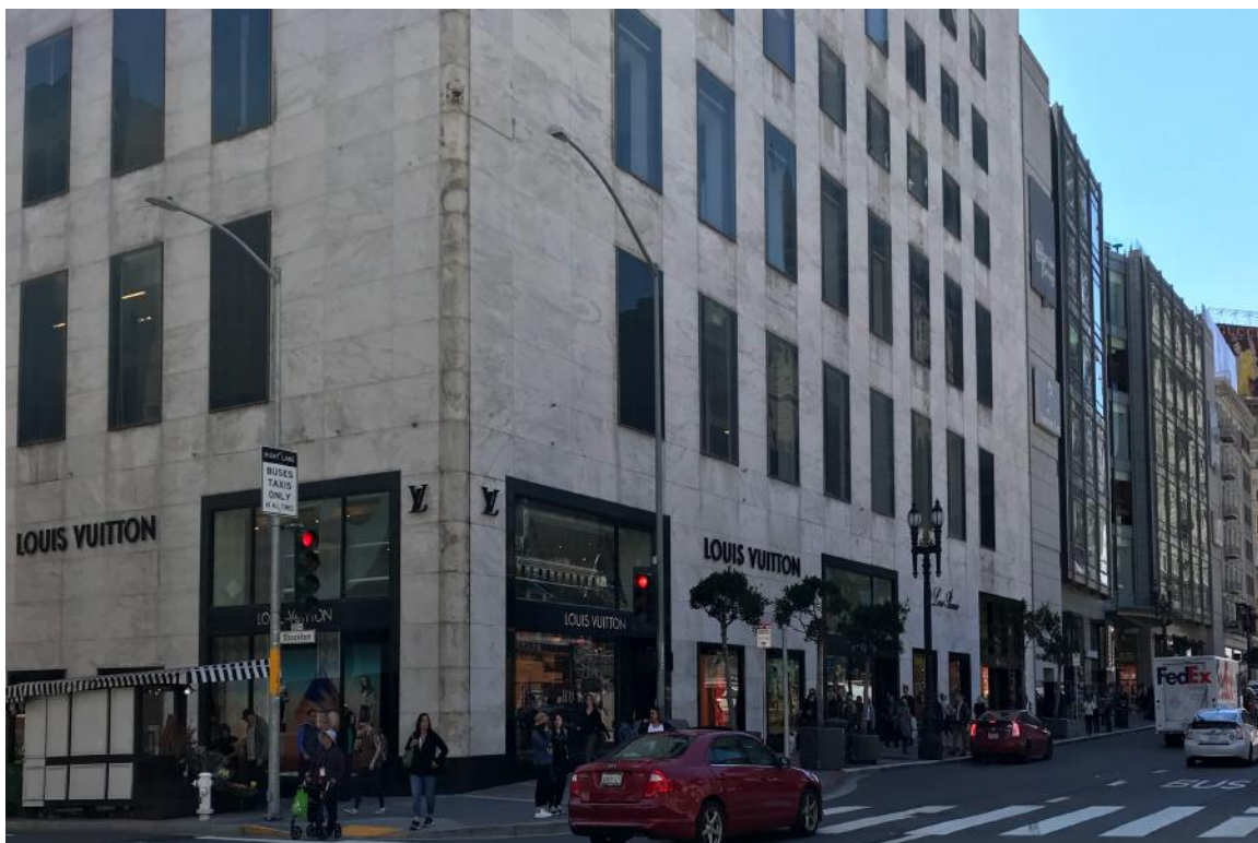
View of lower stories, northeast corner and along north facade.
