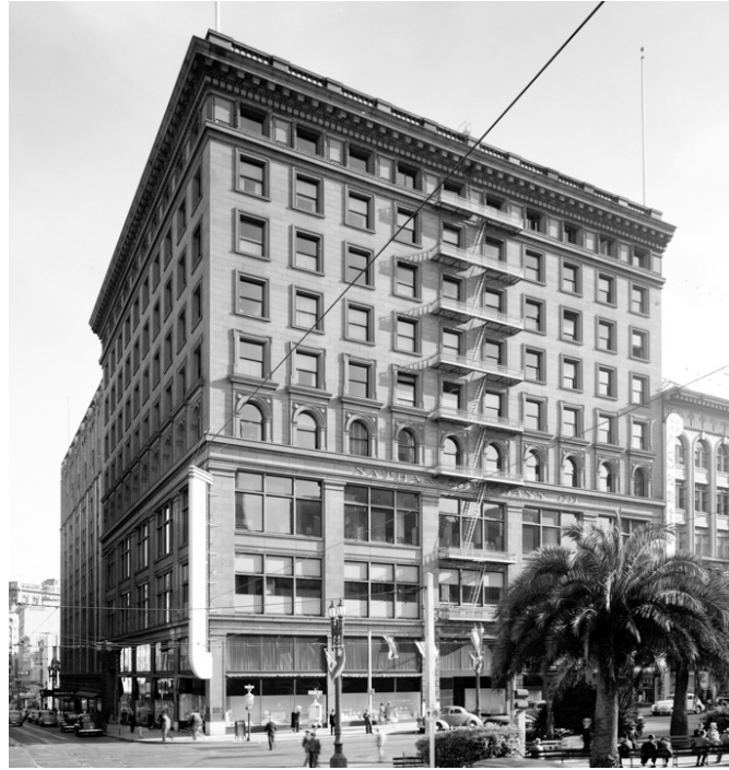
Circa 1905 , the Beaux Arts style mixed-use "Butler Building" supported medical offices and commercial retail uses.
