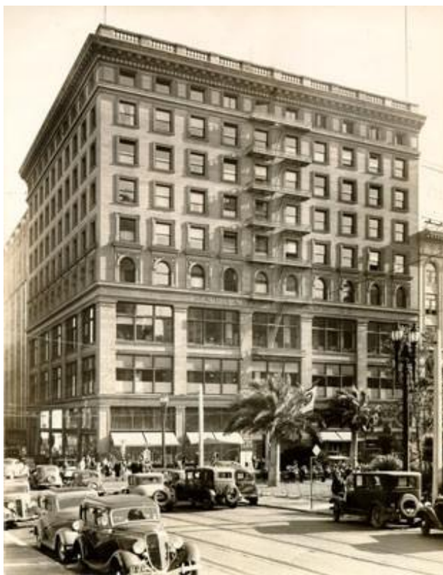
Butler Building 1935. (San Francisco Public Library AAC-7265)
