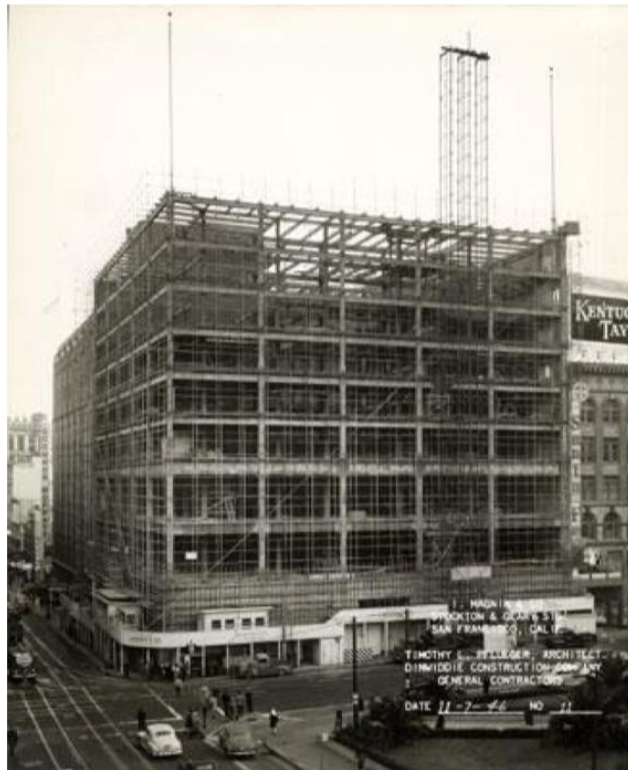
Remodeling in progress, November 1946. (Property owner)
