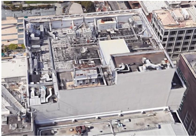
Exposed portion of south facade and rooftop, looking north. (Google Maps)
