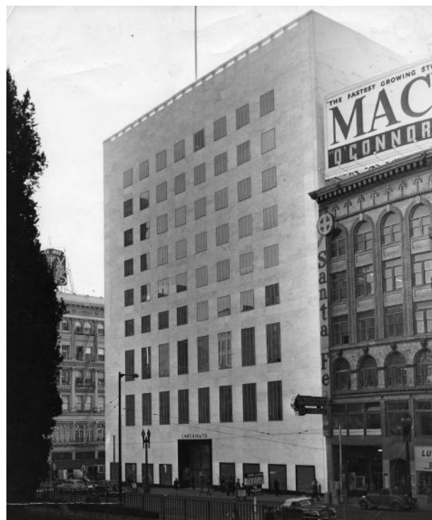
Upon completion of remodeling, 1948. (Property owner)
