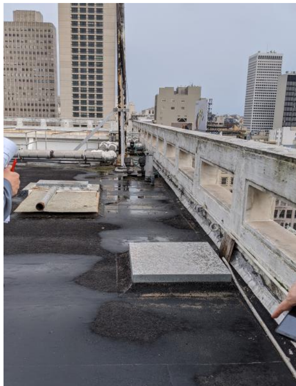
Detail of parapet wall from roof.
