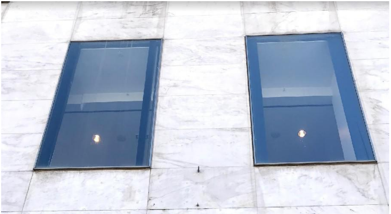
Detail of upper story windows showing projecting metal frames.
