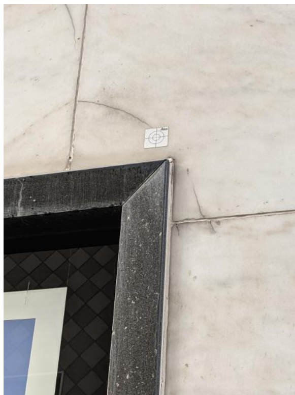
Detail of canted black granite trim around openings.
