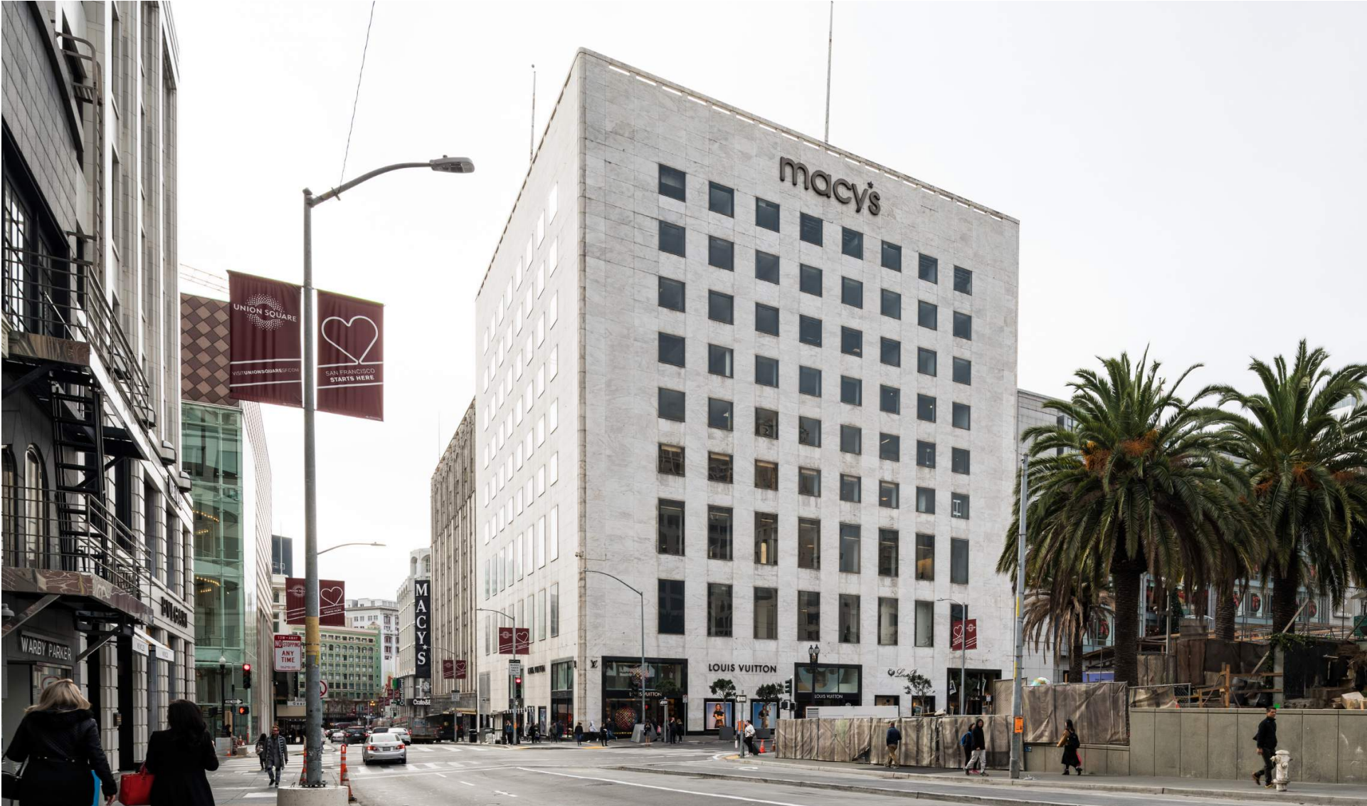
View 1: From Stockton looking south
