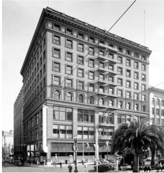
Circa 1905 , the Beaux Arts style mixed-use "Butler Building" supported medical offices and commercial retail uses.
