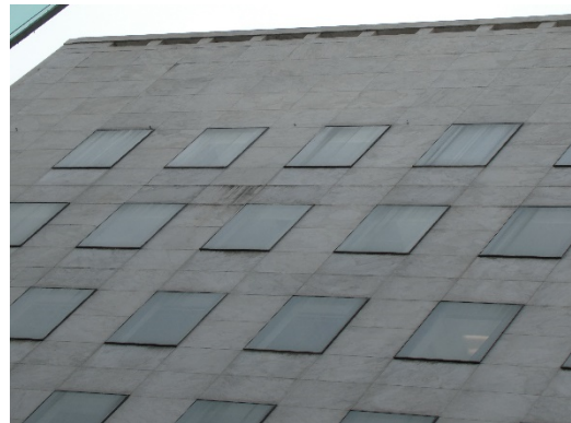
Figure 4: Note soiling across marble panels
