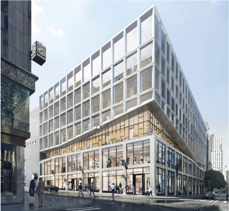
100 Stockton Street - As proposed and currently under construction
