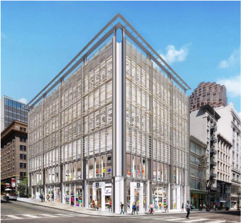
300 Grant Avenue - As proposed and currently under construction
