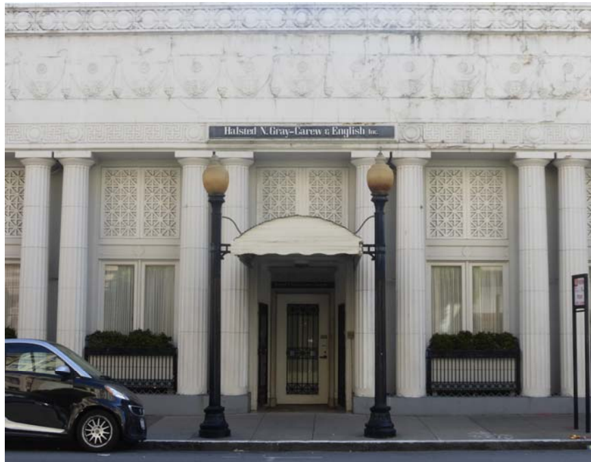
Figure 3. Entrance detail (ARG, October 2019).
