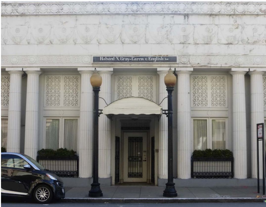
A-2. North elevation, detail of main entry vestibule (ARG, October 2019)
