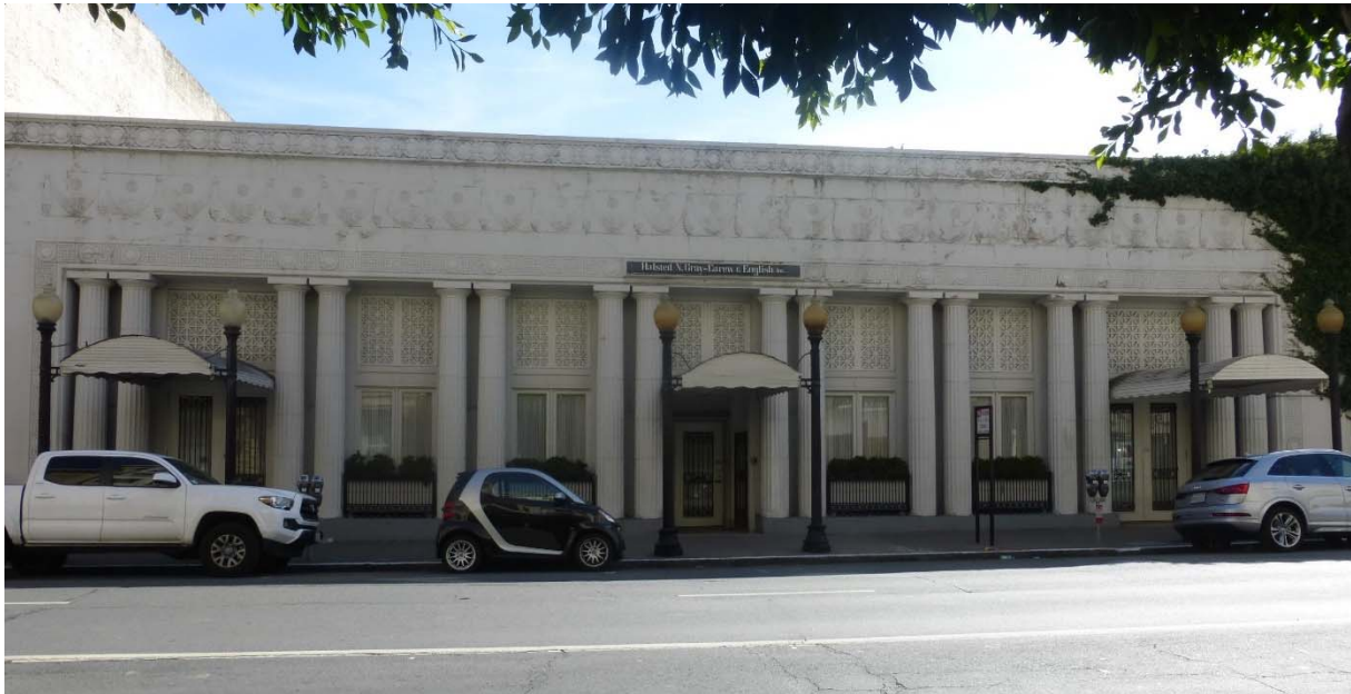
A-1. North elevation, view south from Sutter Street (ARG, October 2019)
