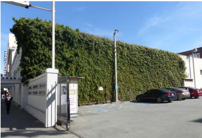
Figure 4. West elevation (ARG, October 2019).
