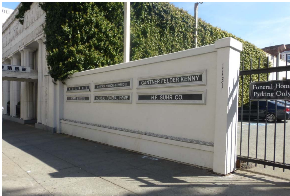
A-4. North elevation, detail view of concrete wall enclosing the parking lot (ARG, October 2019)
