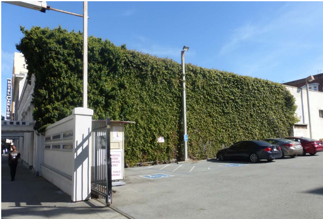
A-5. West elevation, view southeast from Sutter Street (ARG, October 2019)
