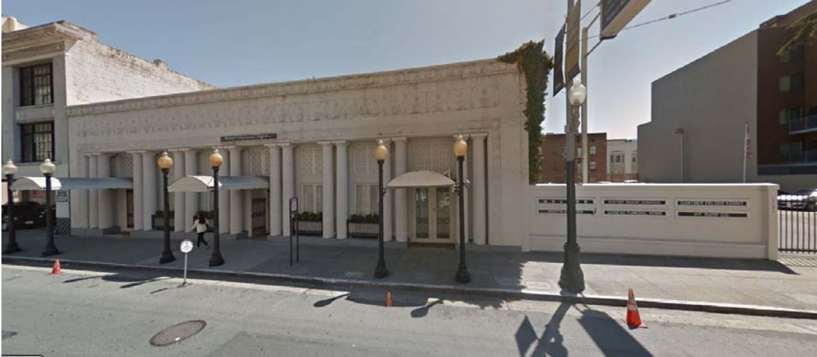
Figure 2. Google Street View of 1123 Sutter Street, primary (north) elevation.
