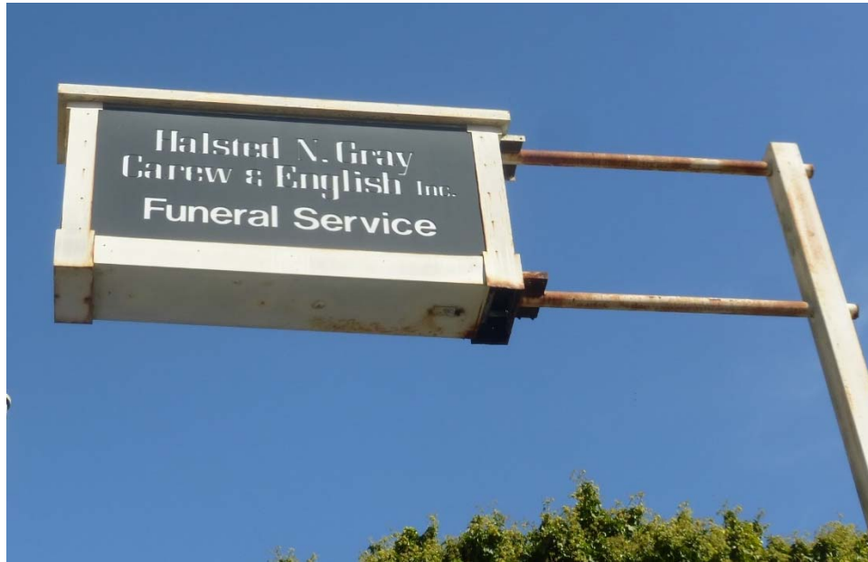
A-4. North elevation, detail view of signage (ARG, October 2019)
