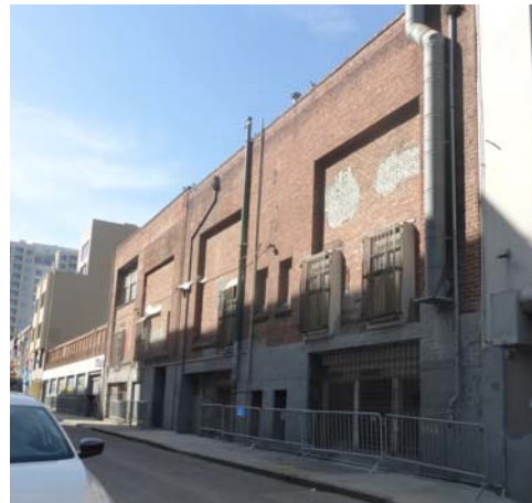
Figure 5. Rear (south) elevation (ARG, October 2019).
