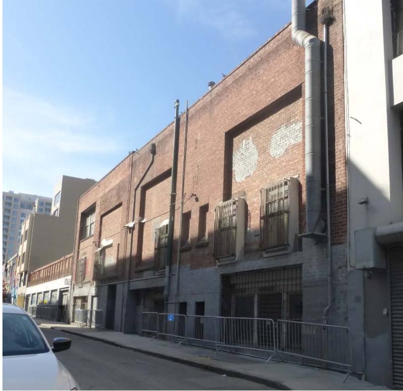
A-6. South elevation, view northwest from Hemlock Street (ARG, October 2019)
