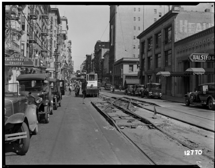
Figure 13. View showing reconstruction of streetcar tracks along Sutter Street, between Polk and Larkin Streets, September 6, 1931; note Halsted & Co. building at 1123 Sutter Street to the right of frame (SFMTA Photo Archive, photo no. U12770, SFMTA.com/Photo ).
