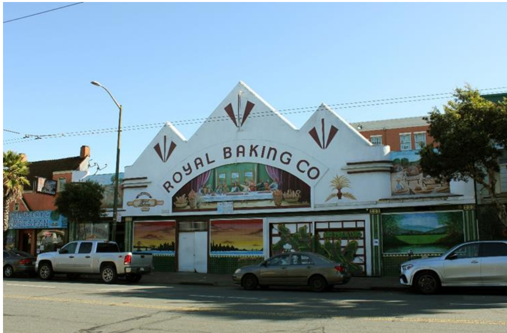
4773 Mission Street façade, January 2020.
