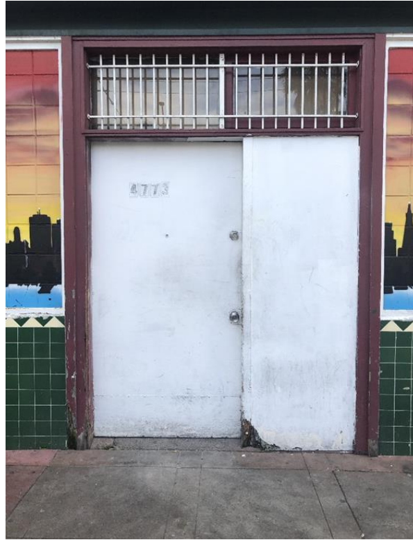
Original storefront entrance opening with replacement door and surround, 4773 Mission Street, January 2020.
