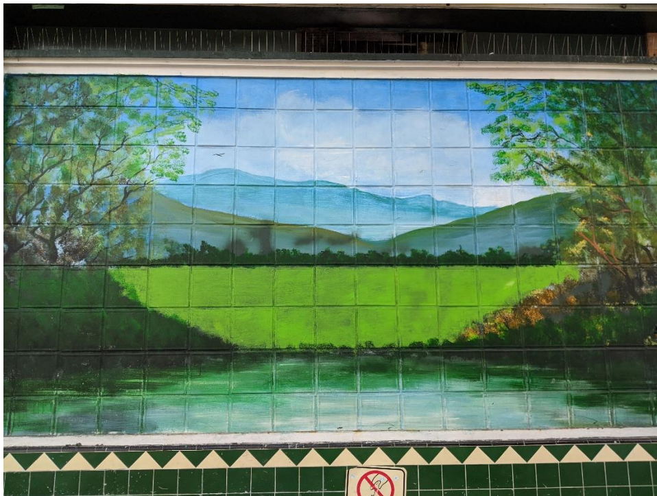
Glass block and ceramic tile infill storefront at 4773 Mission Street, January 2020.
