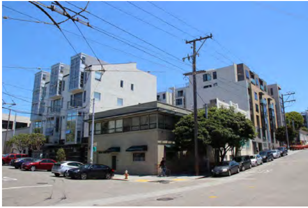
Figure 2. 2440 Mariposa Street (foreground).
