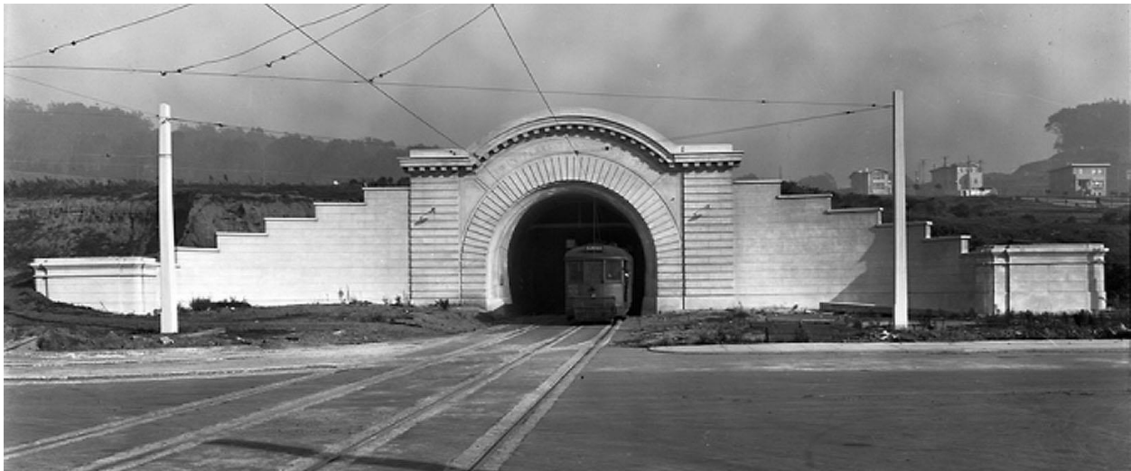
Figure 86. West Portal of Twin Peaks Tunnel, 1919.
