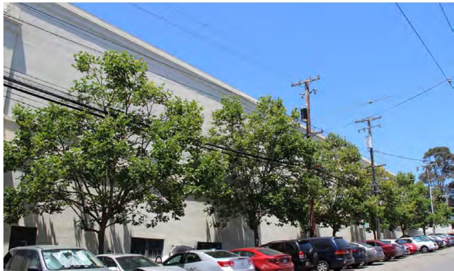
Figure 42. Middle section of secondary façade, looking northwest.
