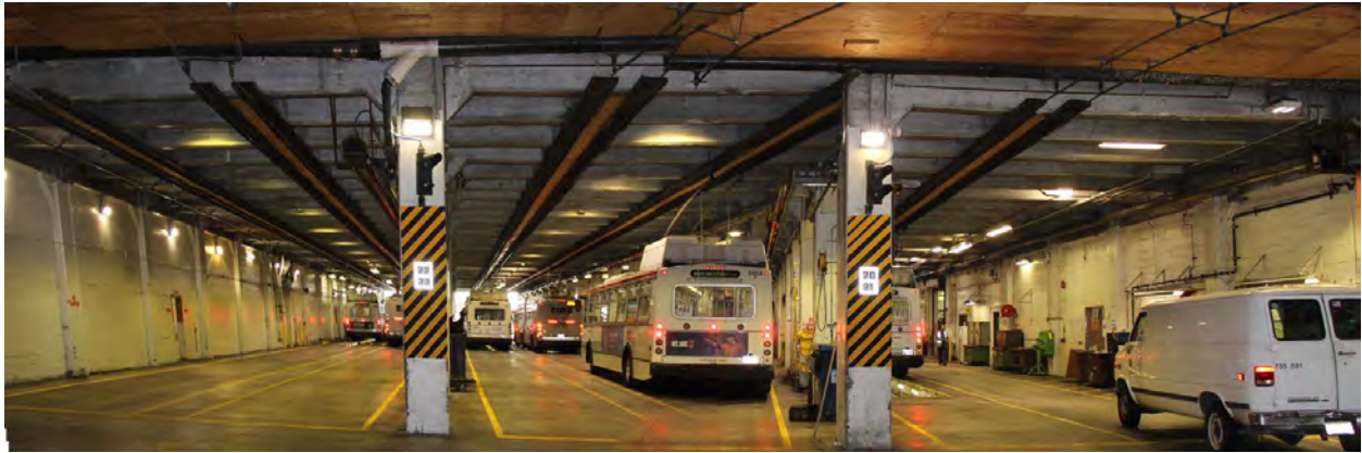
Figure 53. Maintenance bays, looking south.
