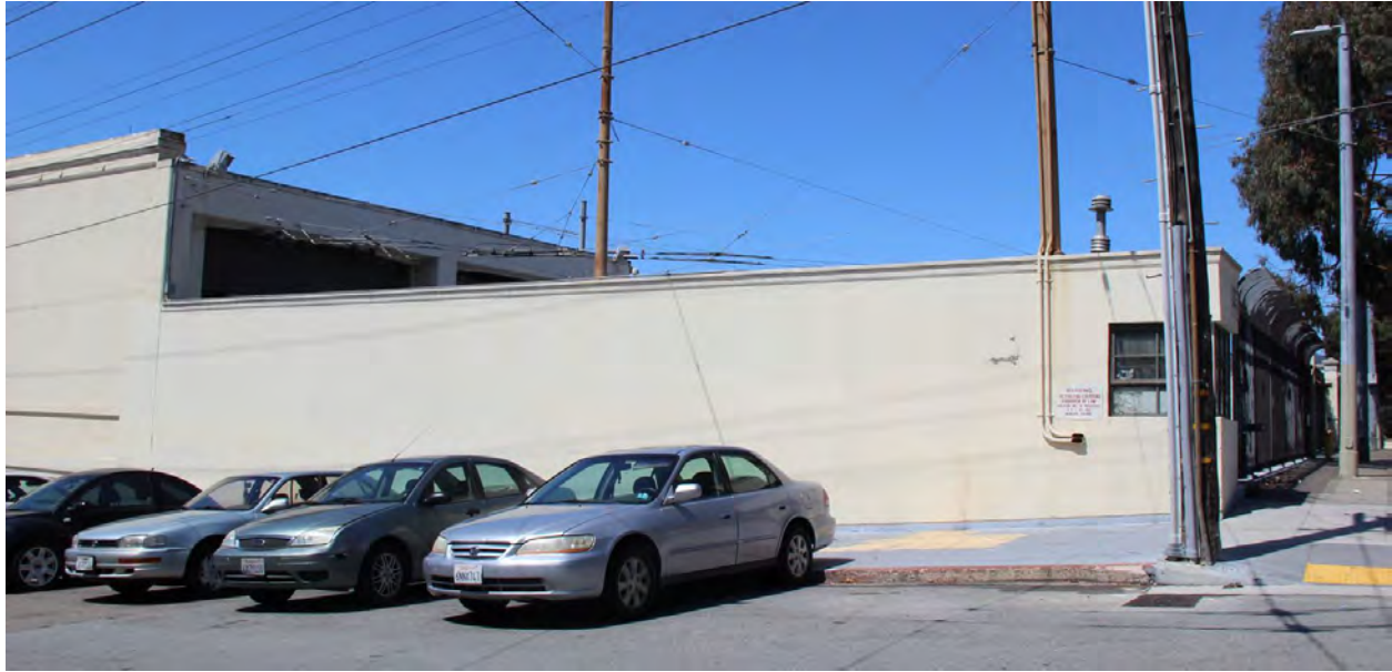
Figure 43. Northern section of secondary façade, looking southwest from Hampshire and 17 th Streets.
