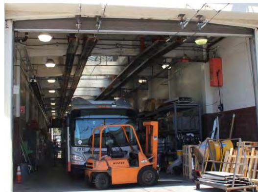
Figure 61. Second floor maintenance shop, looking north.
