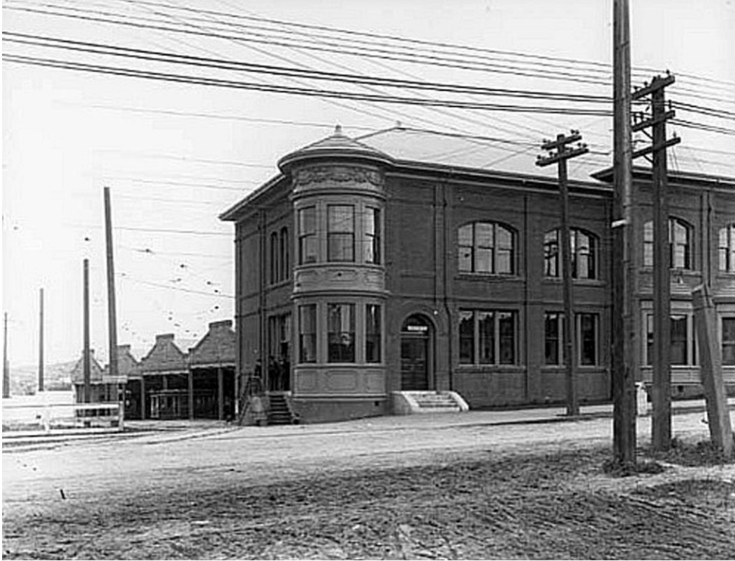
Figure 88. Geneva Car Barn and Powerhouse at San Jose and Geneva Avenues, ca. 1905; built 1901 and repaired 1906.
