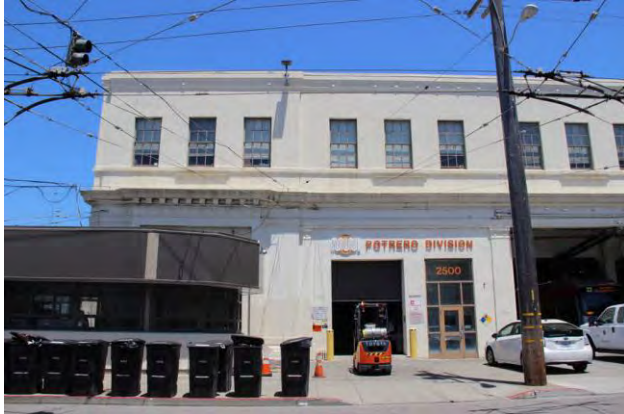
Figure 28. Paved setback in front of maintenance/operations building, looking north.
