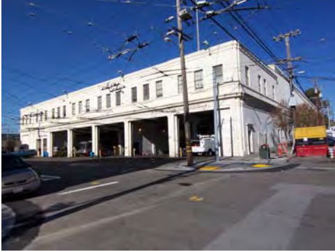
100_5706.JPG, 11/20/2007, view to SW
