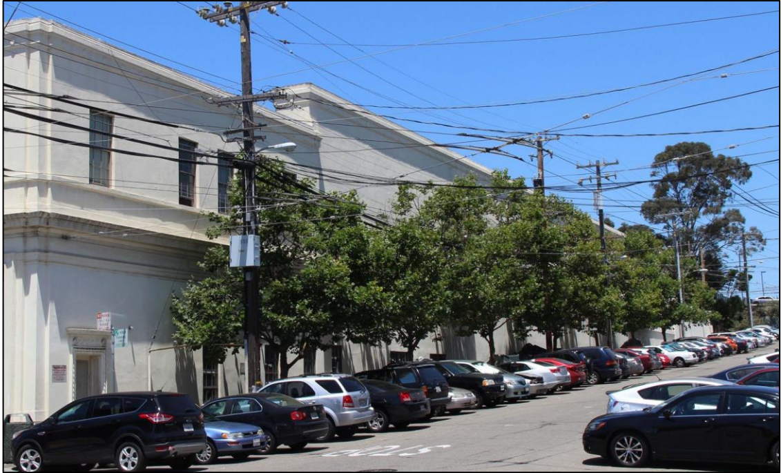
Figure 2: SFMTA Potrero Trolley Coach Division Facility, view northwest of east elevation facing Hampshire Street, (photo courtesy of HRE Part 1). The two story office wing connection is visible where the two parapet walls meet.
