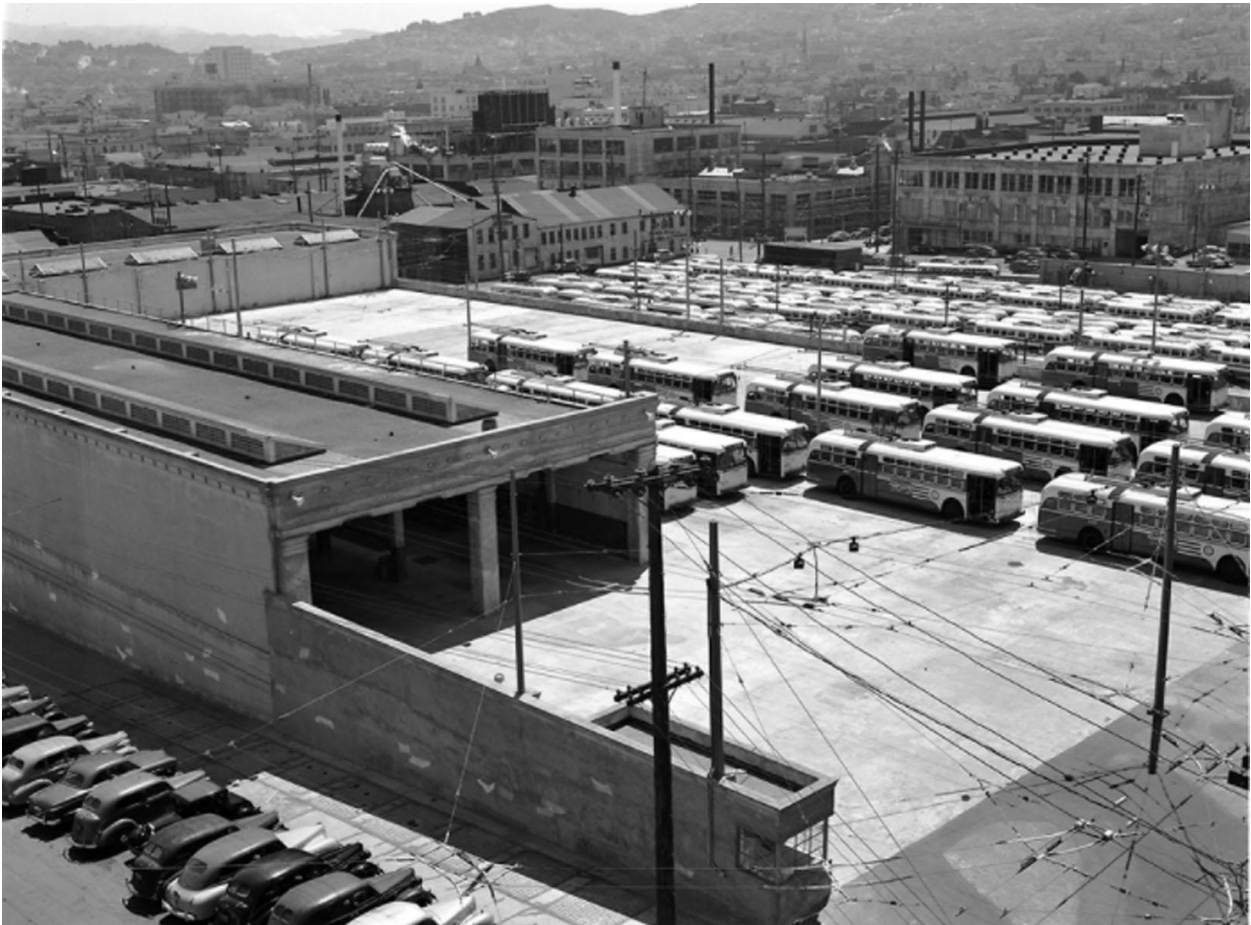
Figure 82. Appearance of the Potrero Trolley Coach Division Facility following 1949 remodel. Source: SFMTA Photography Department and Archive, Image No. X2104
