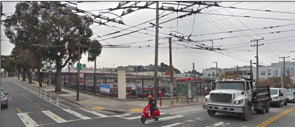
Figure 3: SFMTA Potrero Trolley Coach Division Facility, bus parking lot that occupies the western half of the site, view southeast at the corner of Bryant and 17 th streets, (photo courtesy of Google maps). The surface parking lot that takes up the western portion of the site is visible from this vantage point.
