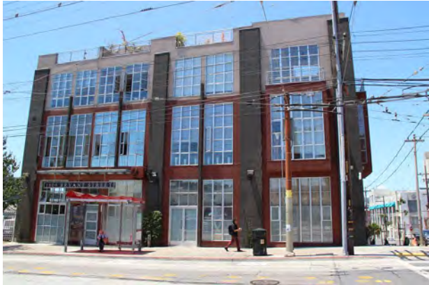
Figure 12. 1800 Bryant Street, looking west.
