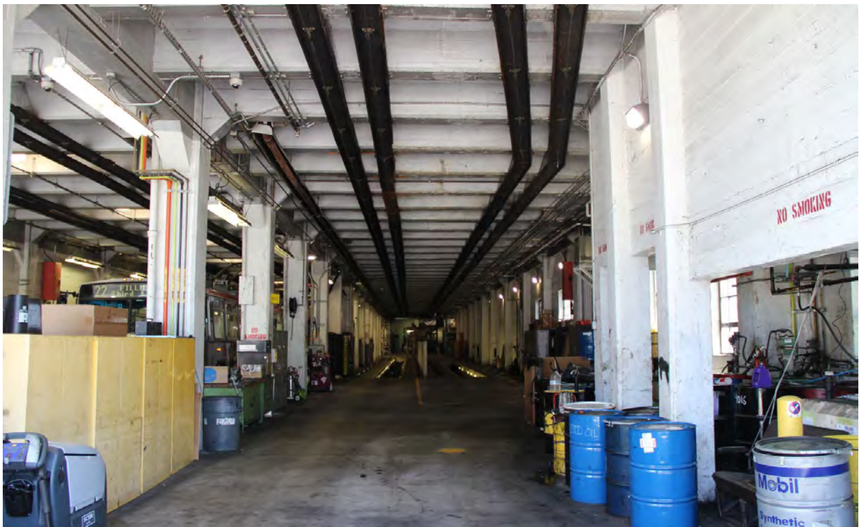
Figure 54. Detail of Bay 29, looking north.
