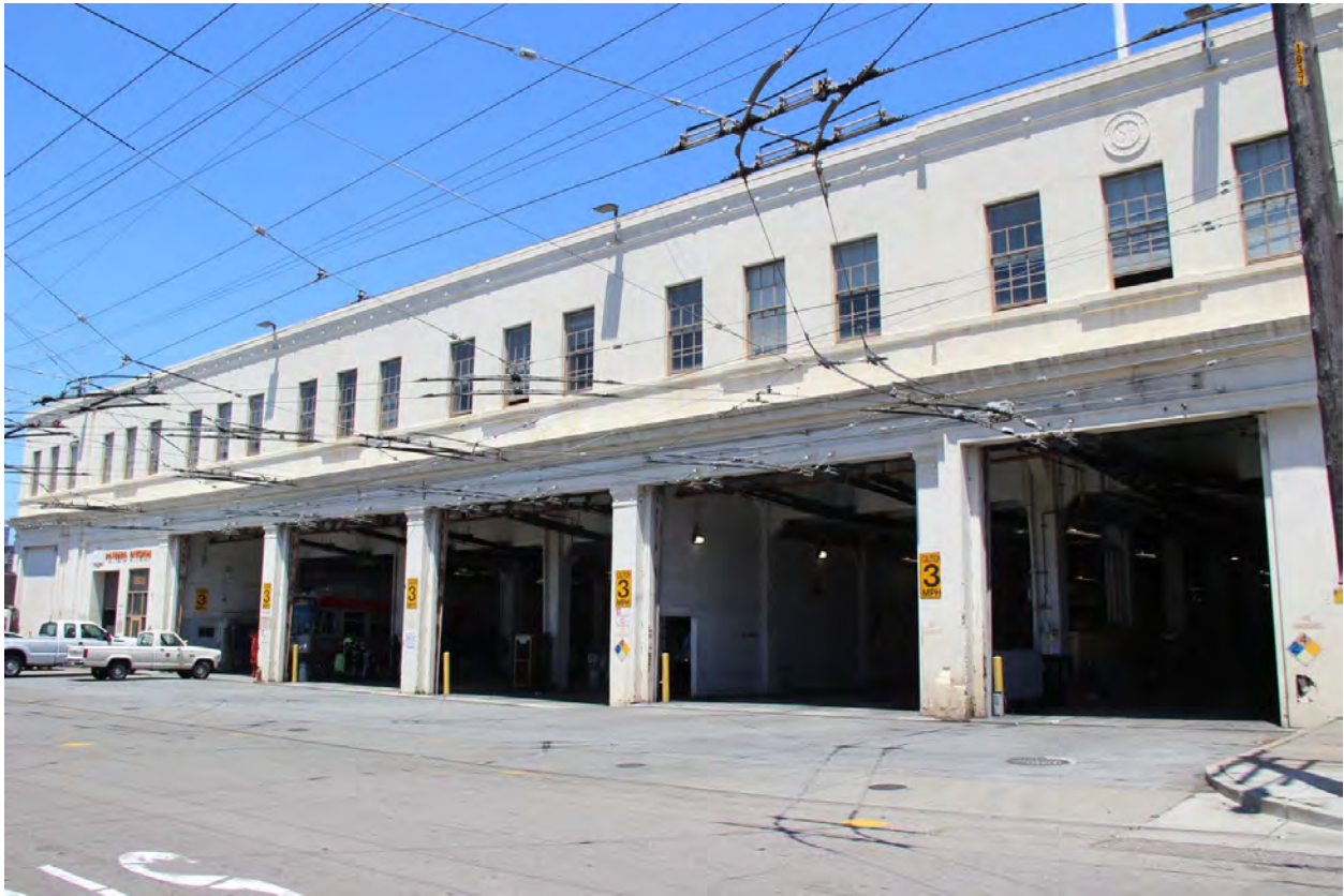
Figure 36. Primary façade, looking northwest.
