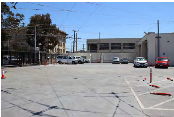
Figure 26. Parking deck, looking east.
