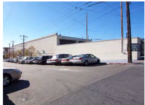
100_5687.JPG, 11/20/2007, view to W, Hampshire St. elevation
