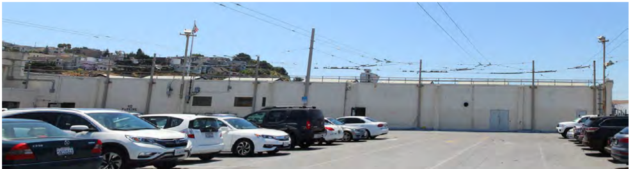
Figure 46. North façade of second floor office wing, looking south from parking deck.
