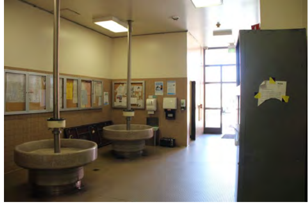
Figure 58. Hand wash station near toilet rooms on west side of first floor level, looking west.
