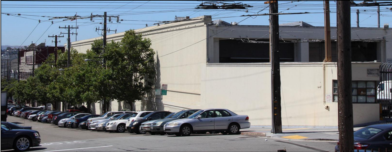
Figure 3: SFMTA Potrero Trolley Coach Division Facility, view northwest of east elevation facing Hampshire Street, (photo courtesy of HRE Part 1). The end of the shops wing is visible here along Hampshire Street at the intersection of Hampshire and 17 th Street.
