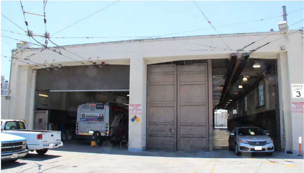
Figure 45. North façade of second floor maintenance shops, looking south from parking deck.
