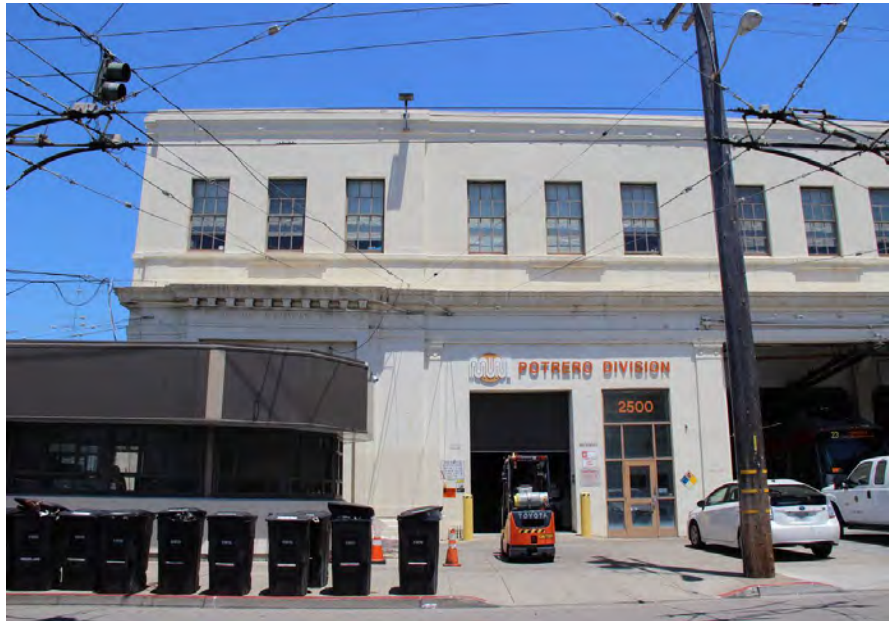
Figure 35. Two westernmost bays of the primary façade, looking north.
