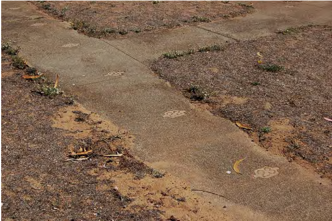
Photo 24. Detail of paved lane layout in trap field with embedded metal tag yardage markers (typical to Fields 1, 2, and 3) (D. Bradley, September 2013).
