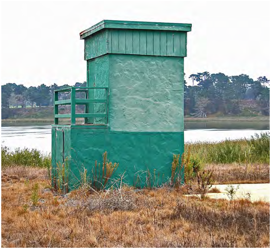
Photo 12. High House (contributing feature) for Skeet Field 5; facing northeast; 15 October 2019.
