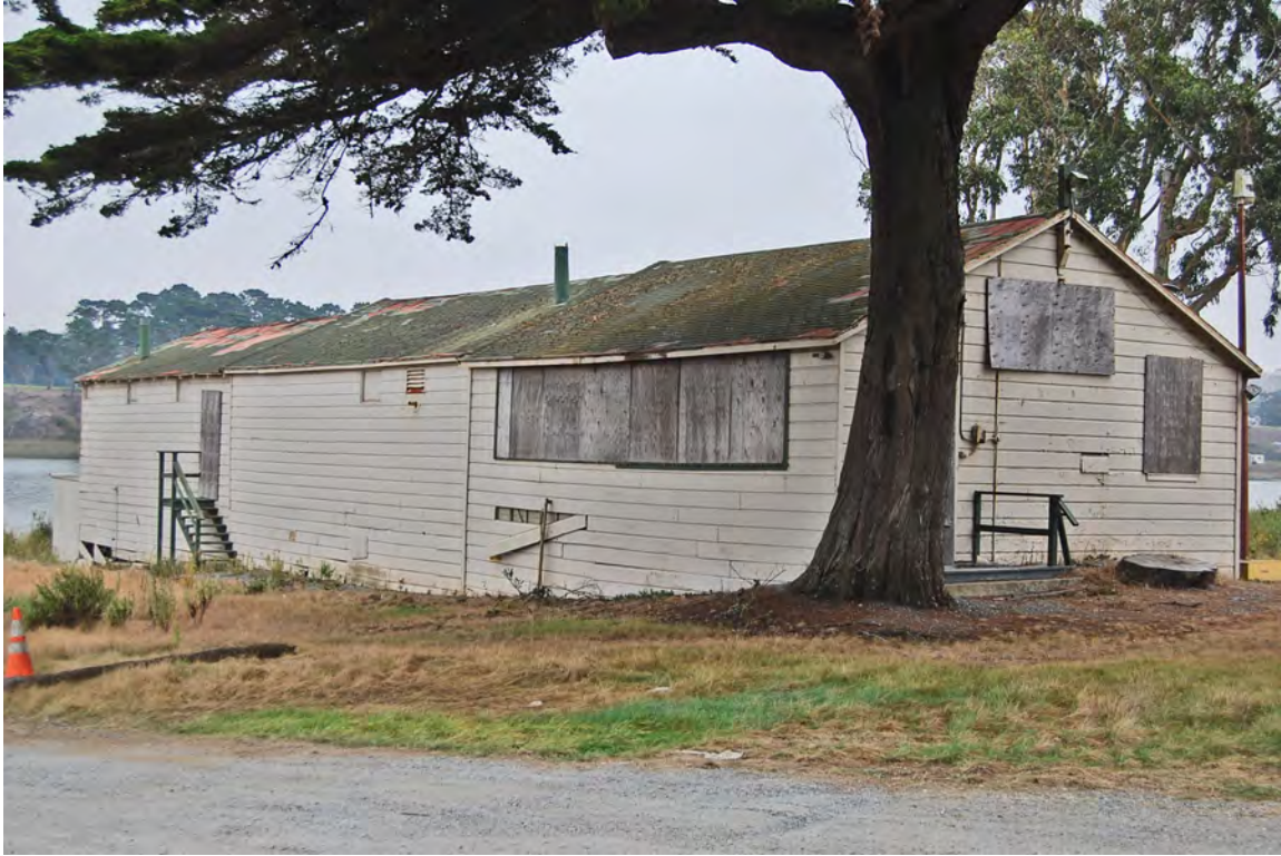
Photo 23. Rifle Range Building (contributing building); facing northeast; 15 October 2019.
