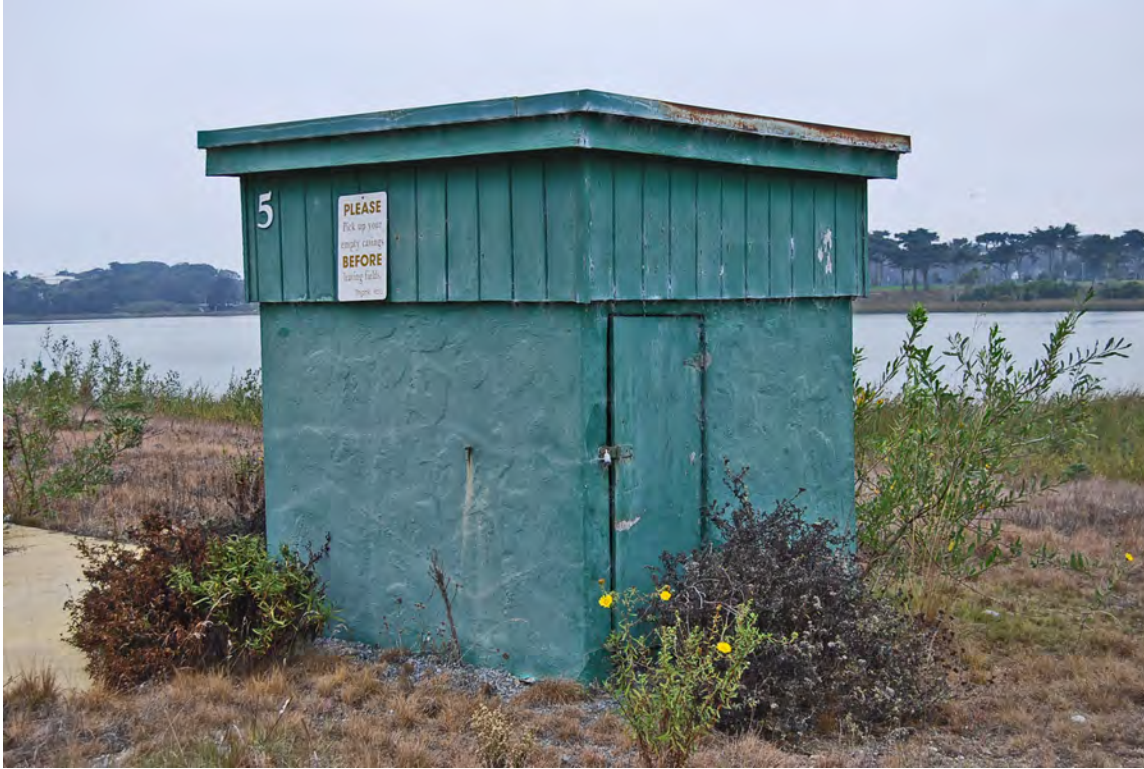
Photo 13. Low House (contributing feature) for Skeet Field 5; facing northwest; 15 October 2019.
