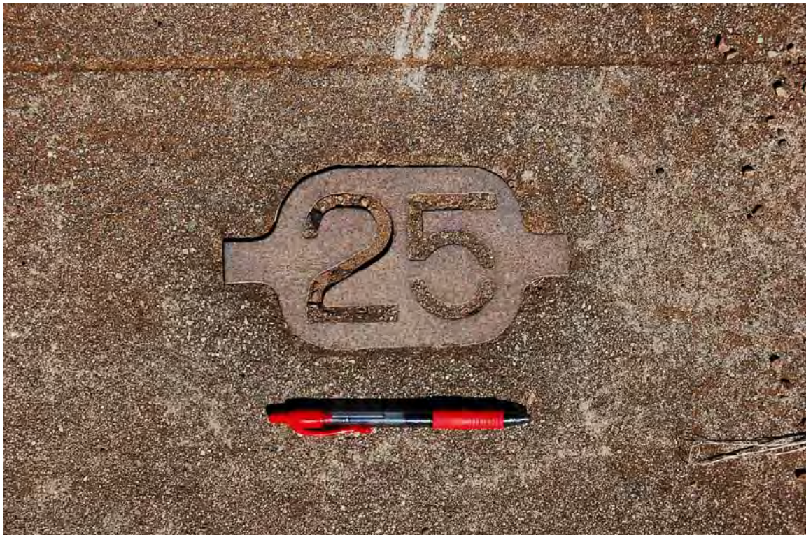
Photo 25. Detail of embedded metal tag yardage markers shown on the paved lane in Photo 24 (D. Bradley, September 2013).
