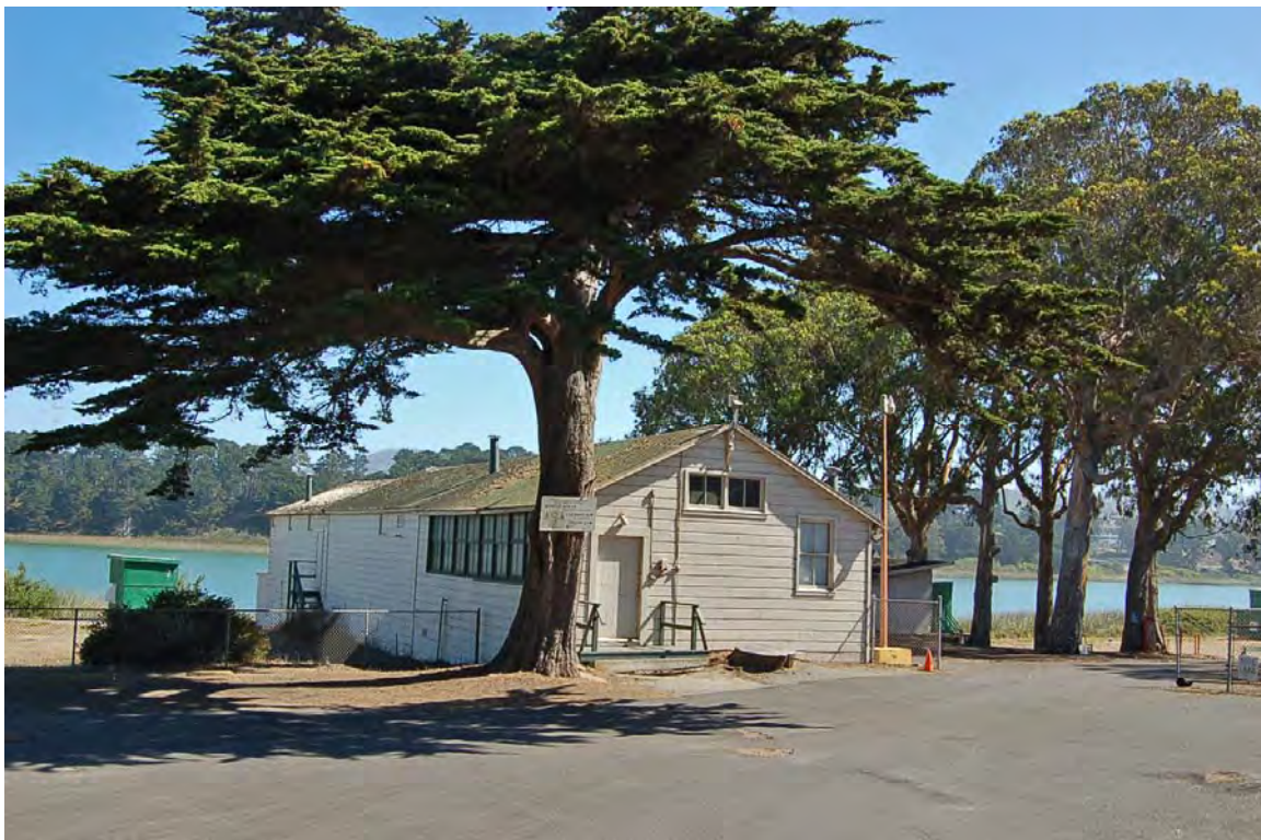
Photo 31. Rifle Range building; entrance flanked on west side by a Monterey cypress (stump of corresponding tree remains on east side of entrance); view to NE (D. Bradley, September 2013).
