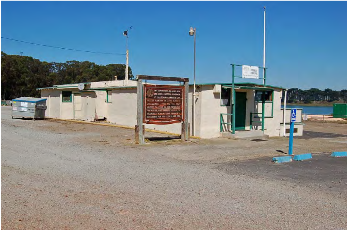
Photo 5. Shell House (ca. 1939-1948) and sign commemorating Merced Rancho (to left); view to N (D. Bradley, September 2013).
