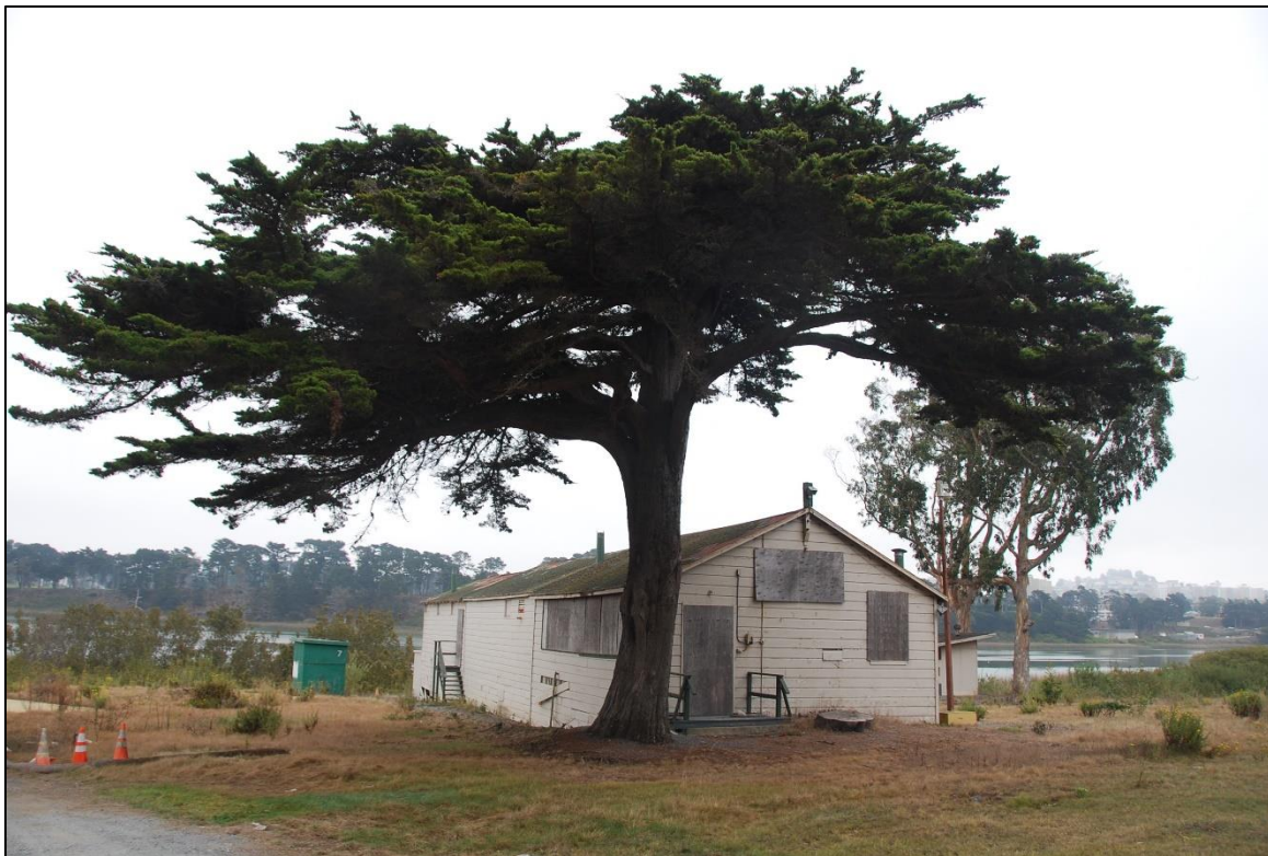
Figure 5: Rifle Range building, a contributing feature (view southeast of west and south elevations)
