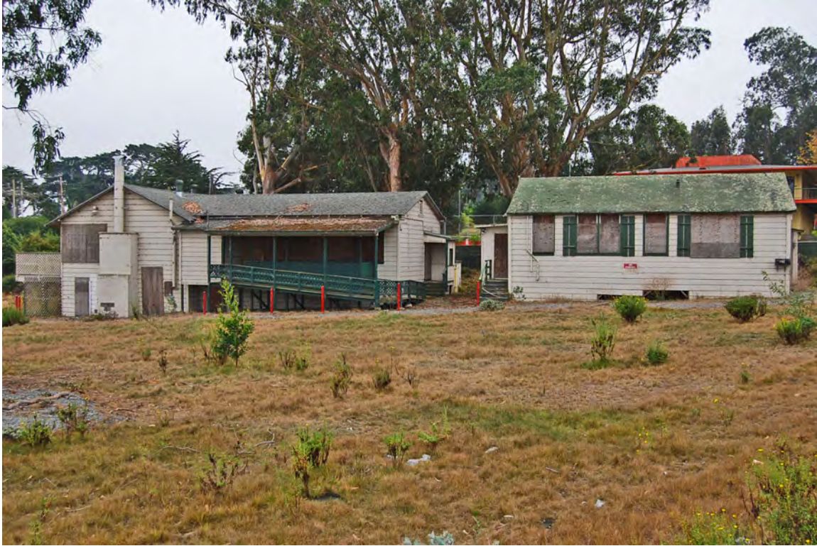
Photo 25. Clubhouse (contributing building) on left and Caretaker's House (contributing building) on right; facing south; 15 October 2019.
