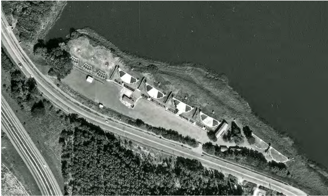
Historic Image 17. Aerial view in 1969. Changes since 1965 aerial (Historic Image 16) include addition of concrete trap yardage marker pavement to the interior of Fields 6 and 7. Source: Pacific Aerial Surveys.
