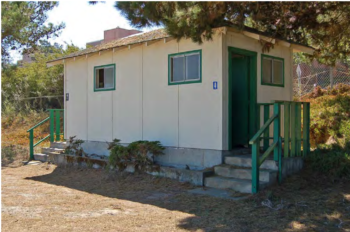
Photo 4. Restroom Building (ca. 1958-1965); view to SE (D. Bradley, September 2013).
