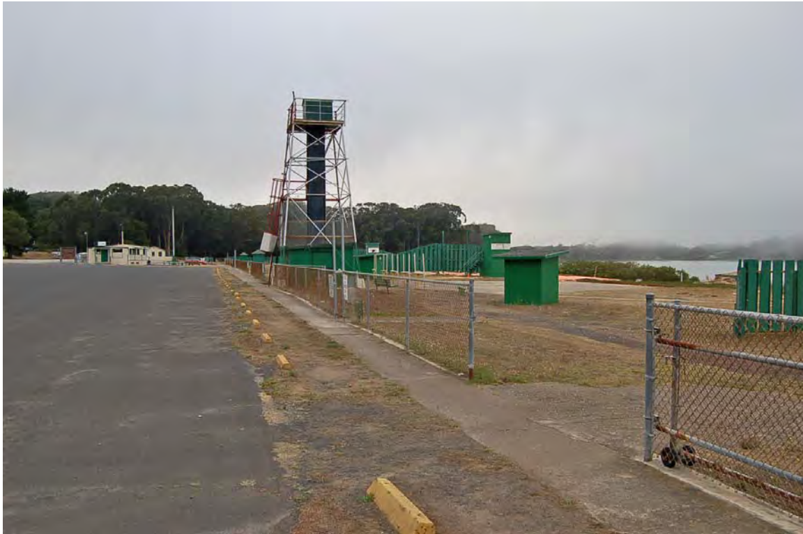
Photo 10. Overview of skeet field complex; also showing sidewalk and remains of planting strip that run along the outer edge of field complex; view to NW (D. Bradley, September 2013).
