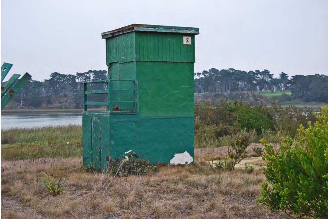
Photo 15. High House (contributing feature) for Skeet Field 6; facing northeast; 15 October 2019.
