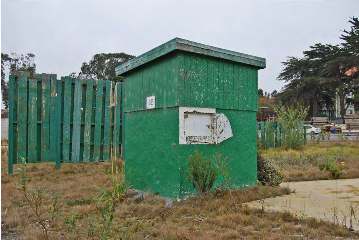
Photo 16. Low House (contributing feature) for Skeet Field 6; facing southeast; 15 October 2019.
