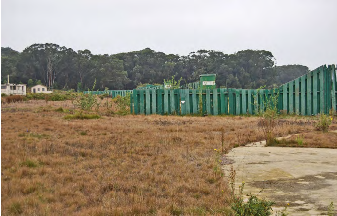
Photo 21. Overview of Skeet Fields 4 to 7 (contributing features) showing linear arrangement (contributing spatial organization characteristic) and level terrace (contributing topographic characteristic); facing west/northwest; 15 October 2019.
