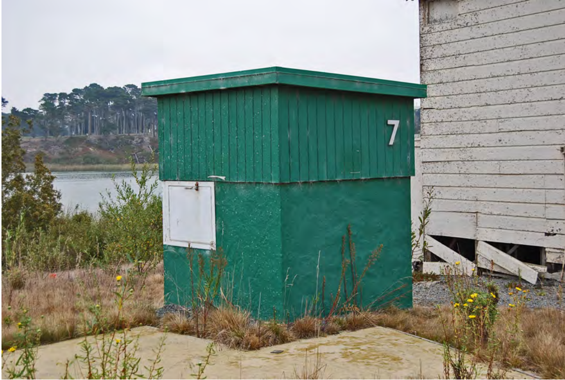
Photo 19. Low House (contributing feature) for Skeet Field 7; facing northeast; 15 October 2019.
