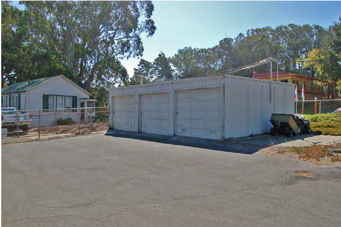
Photo 32. Garage; view to SE (D. Bradley, September 2013).
