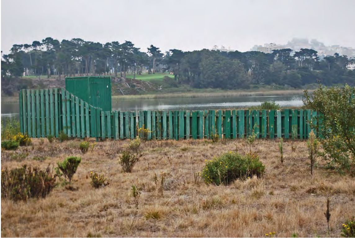
Photo 9. Safety fence (contributing feature) on west side of Skeet Field 4; facing east; 15 October 2019.
