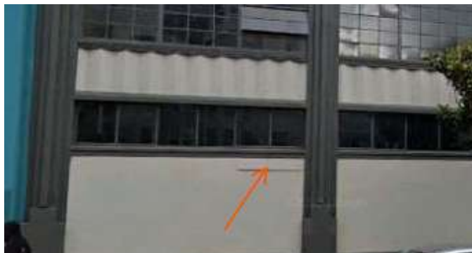
Figure 18. The eastern part of the Howard Street façade. There is a board attached to the stucco infill (red arrow). Google Street View.
