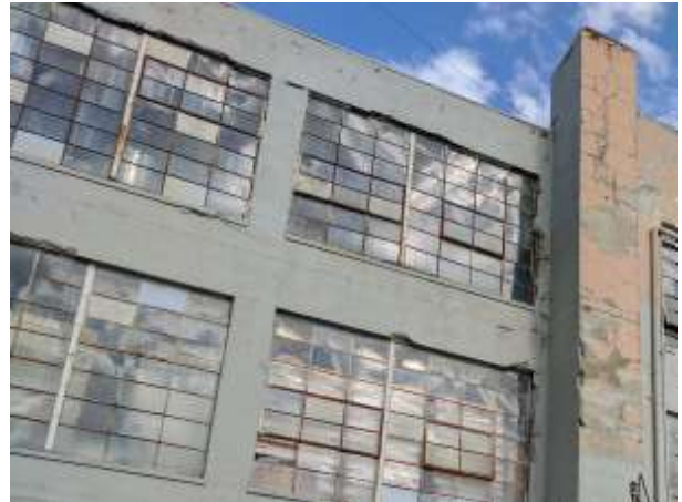
Figure 6. Undecorated southern façade. Knapp Architects photo, 2017.
