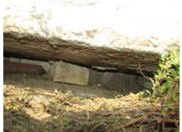
Figure 42. Inside the gap under the first floor slab. Knapp Architects photo, 2019.
