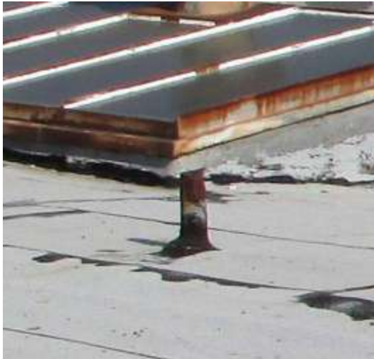
Figure 69. Typical vent stack penetration at the roof. Knapp Architects photo, 2019.
