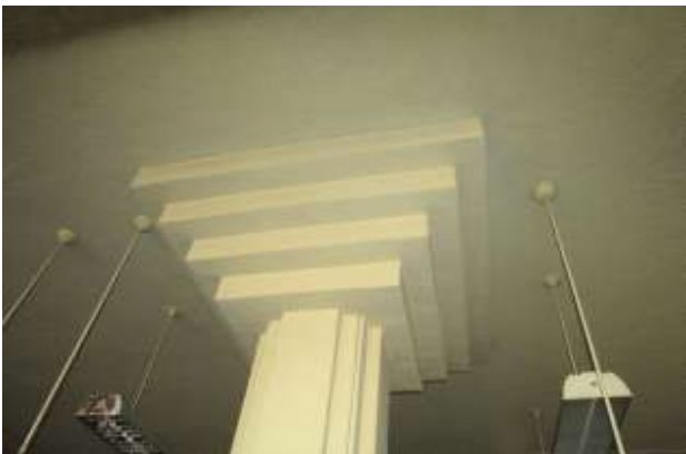
Figure 13. Typical stepped column and capital. Knapp Architects photo, 2019.
