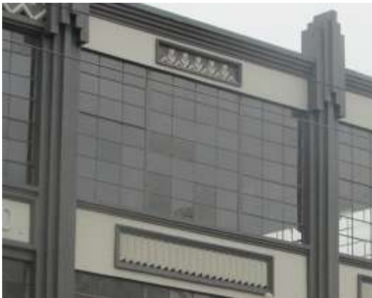
Figure 7. Typical window at decorated façade, also showing stepped column and finial capital and decorated spandrel panels. Knapp Architects photo, 2018.
