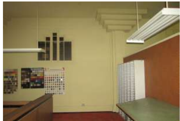
Figure 14. Rear wall of office showing stepped pilaster and capital and stepped window to mezzanine. Knapp Architects photo, 2018.
