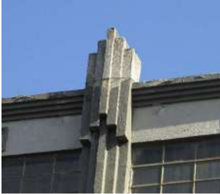
Figure 23. Wire around stepped finial capital. Knapp Architects photo, 2019.
