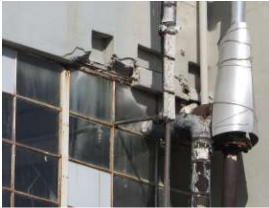
Figure 43. There is a substantial spall at the window head of the second floor window of the westernmost bay on the south facade. Knapp Architects photo, 2019.
