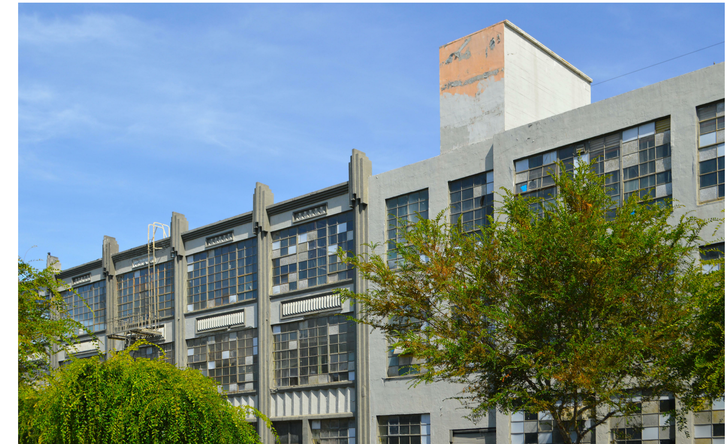
Russ Street Facade Detail
