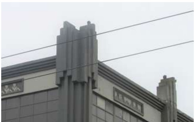
Figure 10. Finial capitals at building corner. Knapp Architects photo, 2018.
