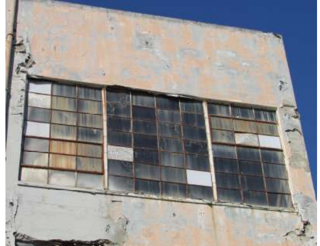
Figure 54. The third-floor window of the easternmost bay. Knapp Architects photo, 2019.
