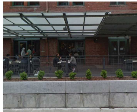
PANEL TO PANEL - EXISTING CONDITION
