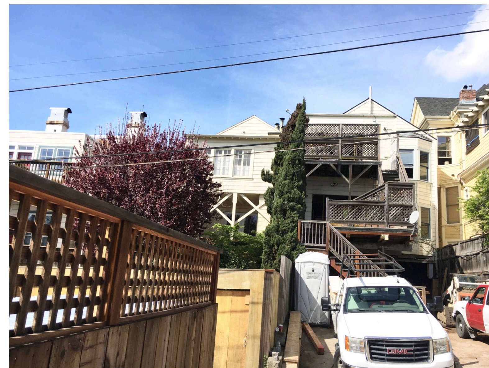
ADJ BLDG SOUTH
