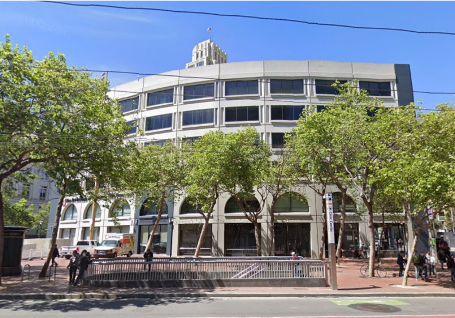
*Market Street façade.
