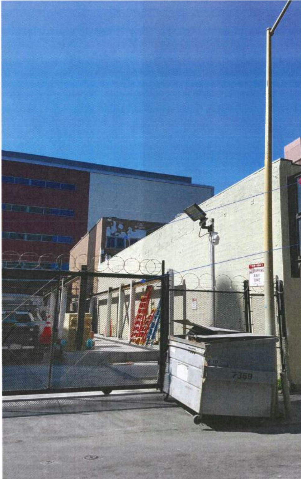
NRG-barbed wire fencing and a new structure encroaching on our ability to maintain our building. Behind that, a run-down small building waiting to get permits.
