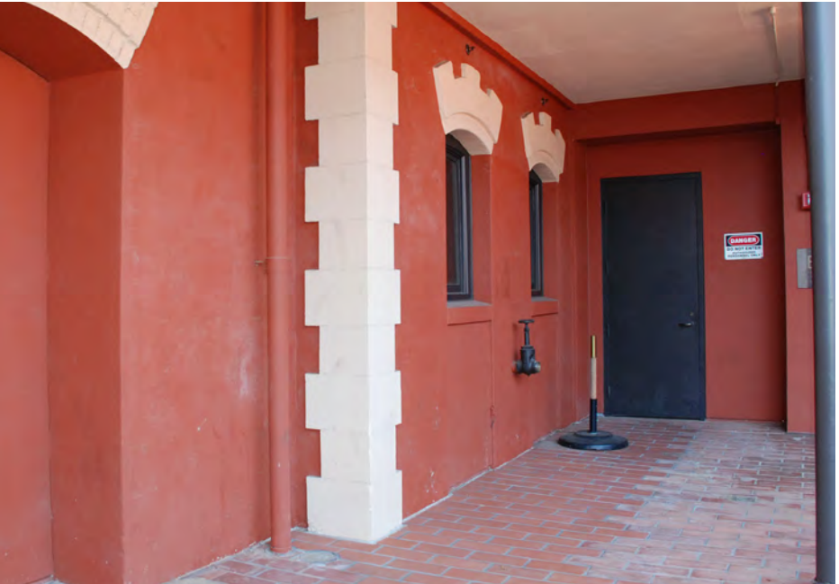
Inappropriate - some of the original Ghirardelli Buildings have areas where the original brick was refinished with cement plaster and painted to match the brick paving.
