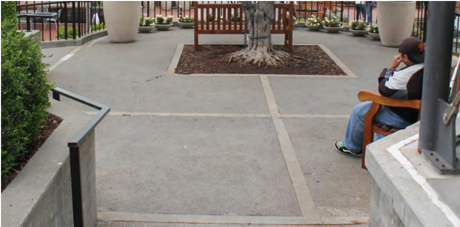
Existing seeded aggregate paving with concrete banding
