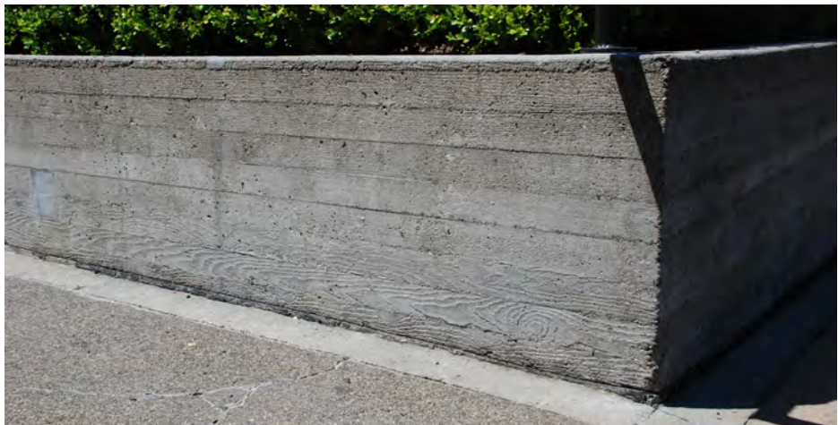
Appropriate existing paving and walls at Ghirardelli Square includes seeded concrete and board formed concrete.
