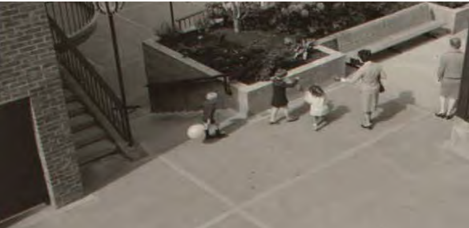
View of Upper Plaza in the 1960’s demonstrates the character defining angular board form concrete walls and planters from that era (Environmental Design Archives)
