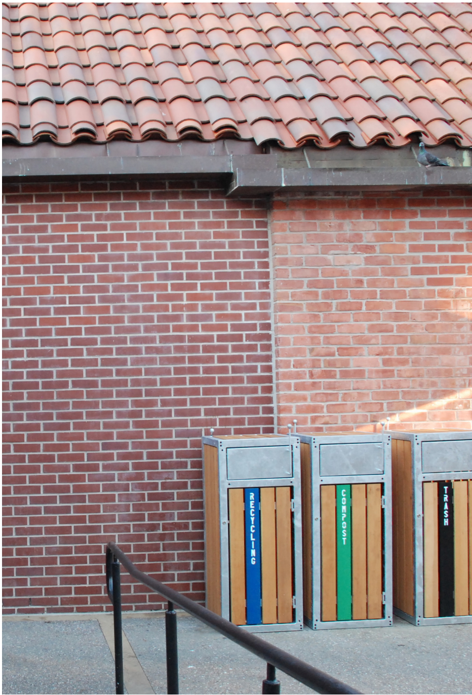
6. View of Restroom Building brick (left) and Wurster Building sand mold brick (right).
