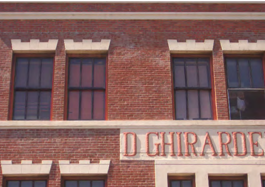
Several of the original Ghirardelli Buildings have double-hung steel windows.
