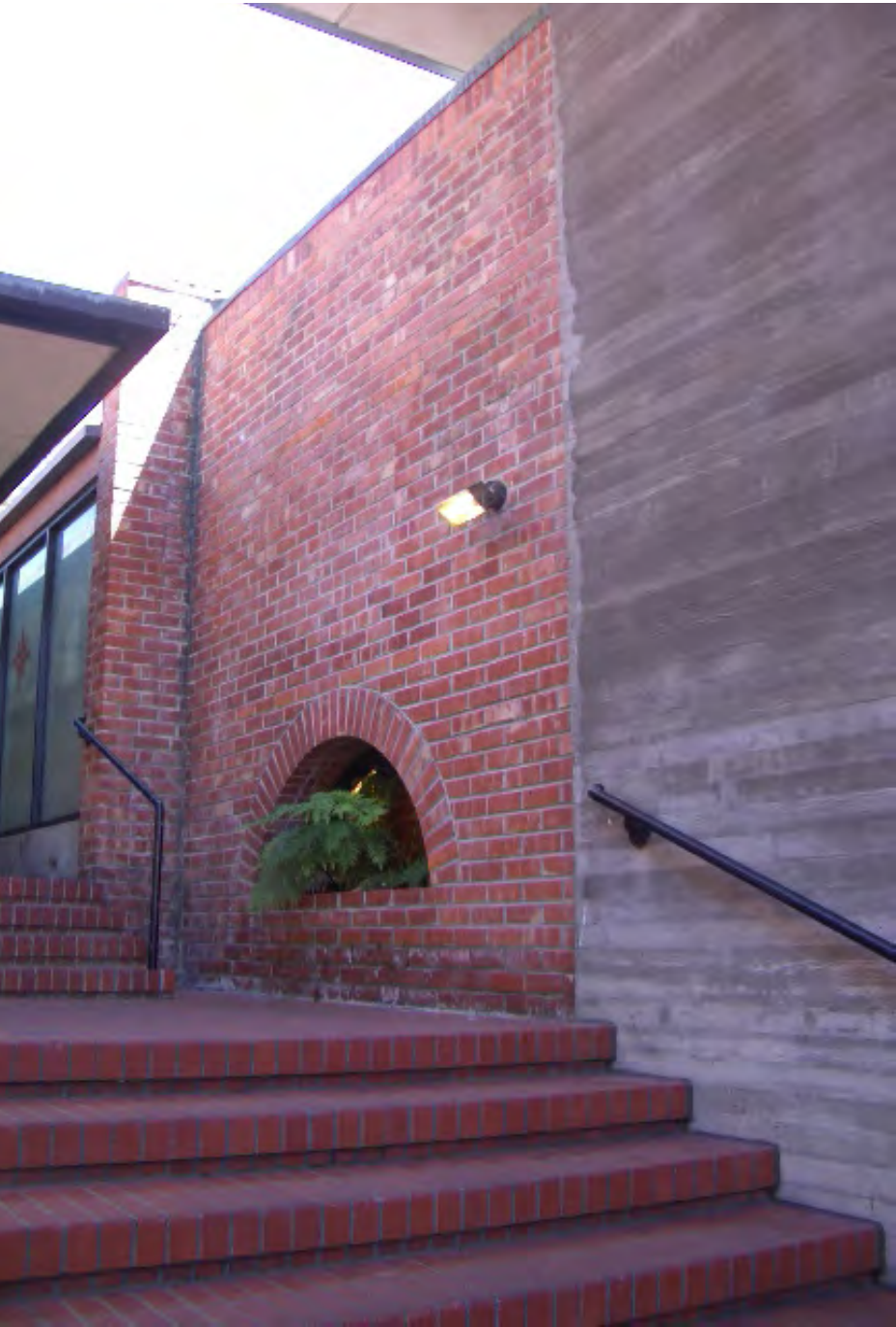
Several of the 1960s buildings incorporate board form concrete.
