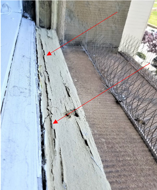
Figure 5 - Compromised sill, checking and cracking.
