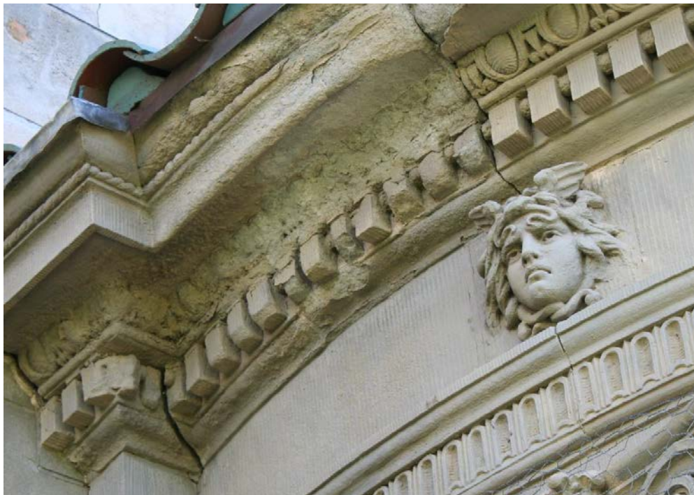
IMAGE 18. Detail of displacement and severe deterioration at portico cornice.
