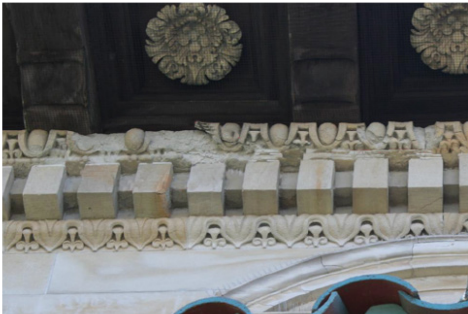
IMAGE 9. Detail of material loss and incipient spalling at cornice.
