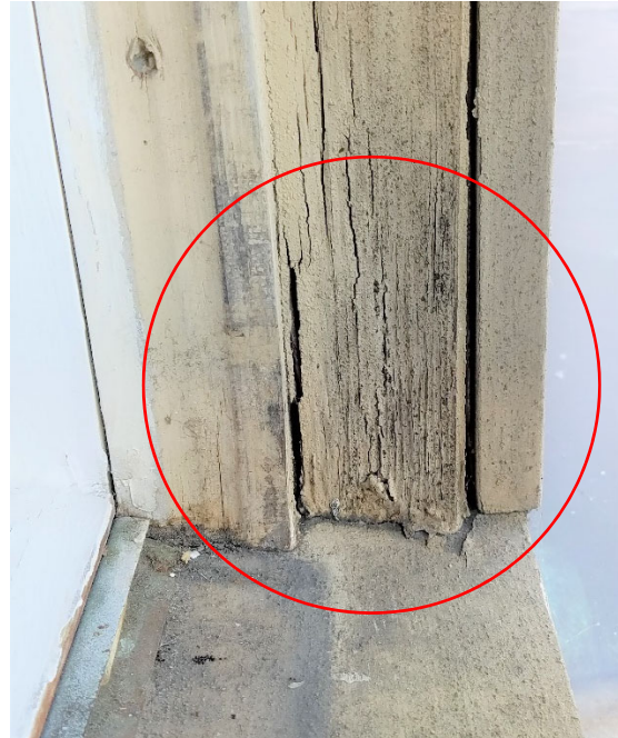
Figure 6 - Failing jamb, checking and separation.
