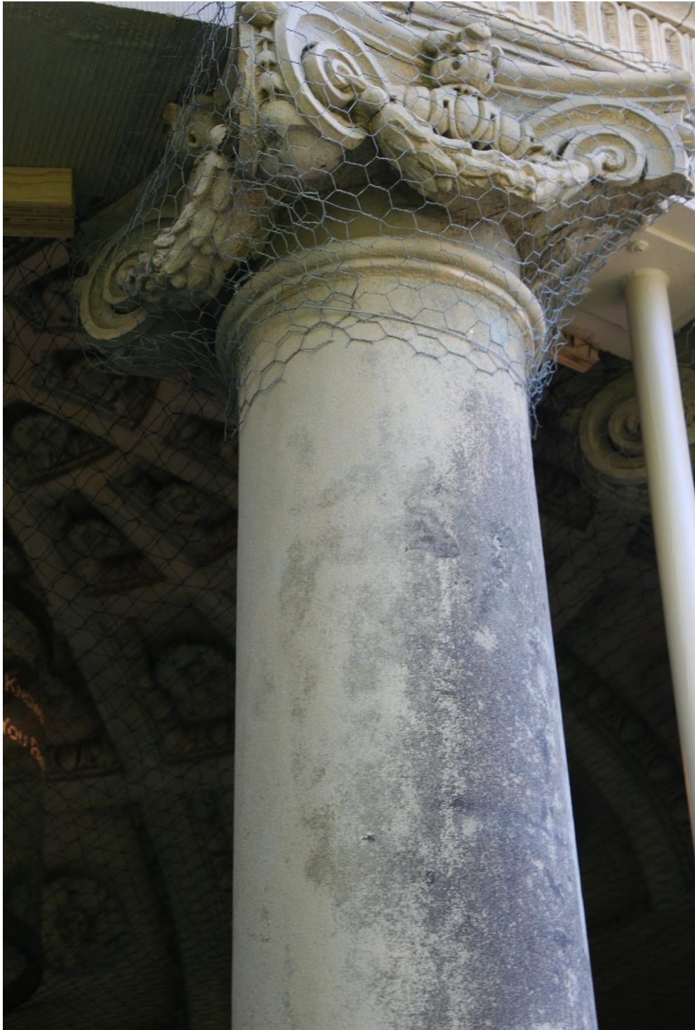
IMAGE 12. Material loss and environmental staining at portico column.
