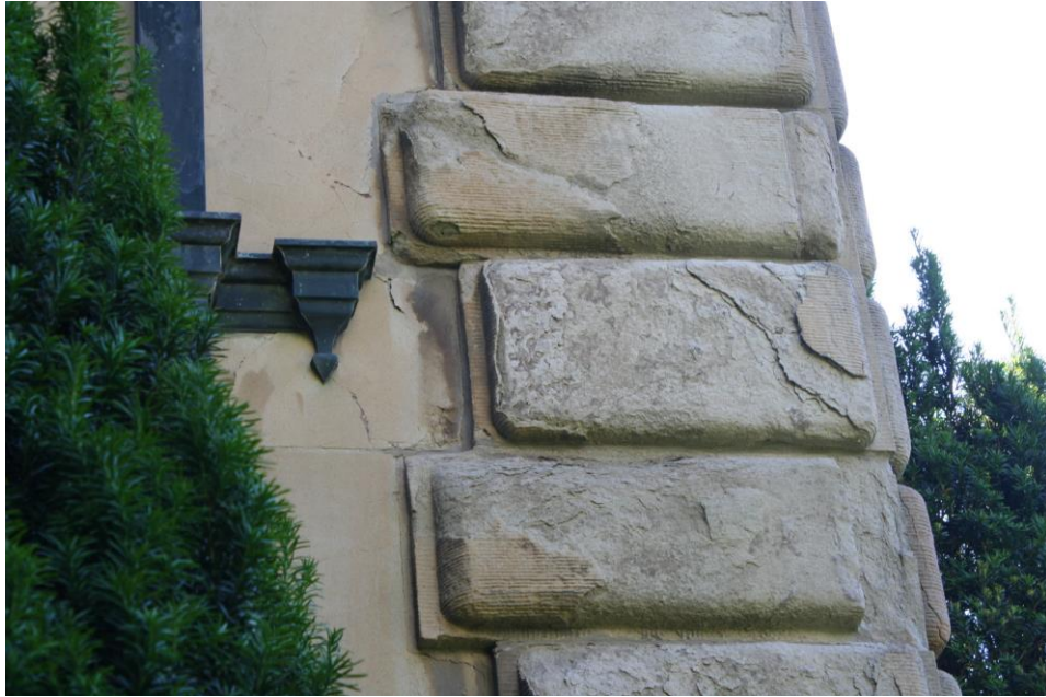
IMAGE 8. Deterioation and material loss at quoins.
