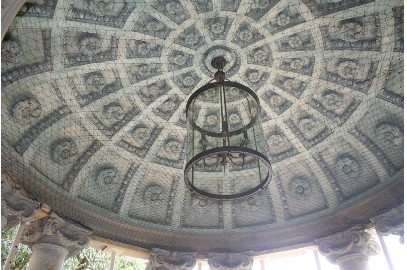
IMAGE 24. Overview of decorative plaster dome at interior of portico. This area will be protected and suspended in place during the stone restoration work.
