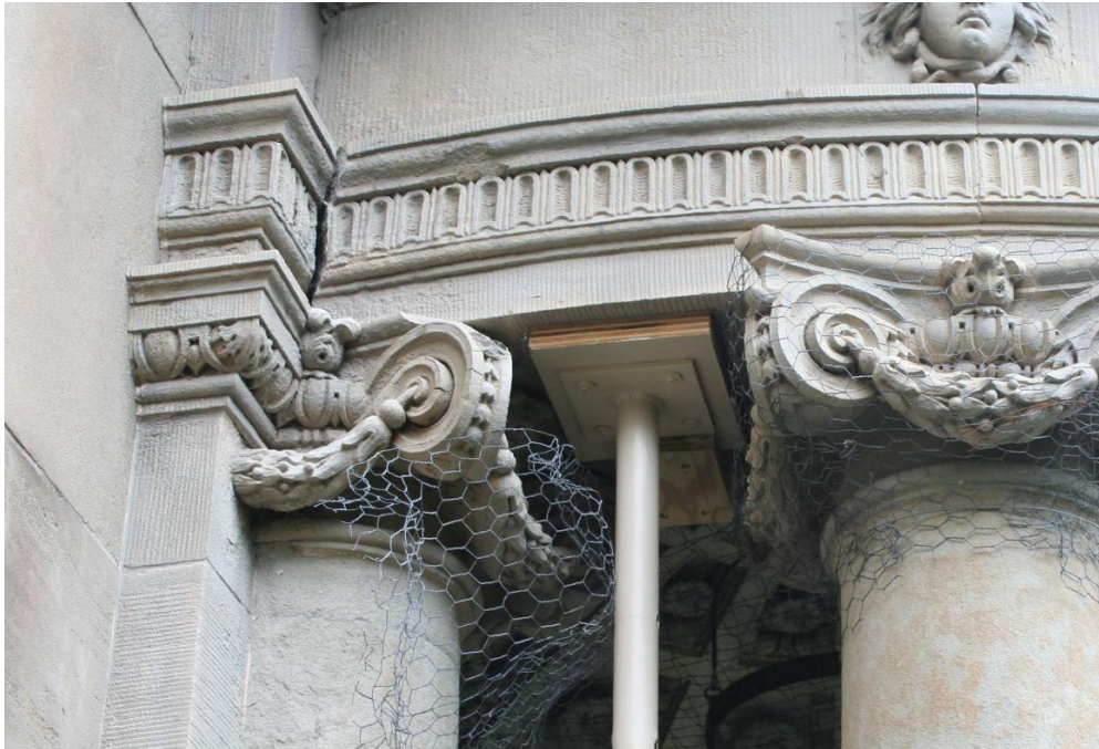
IMAGE 17. Displacement and structural cracking at portico.
