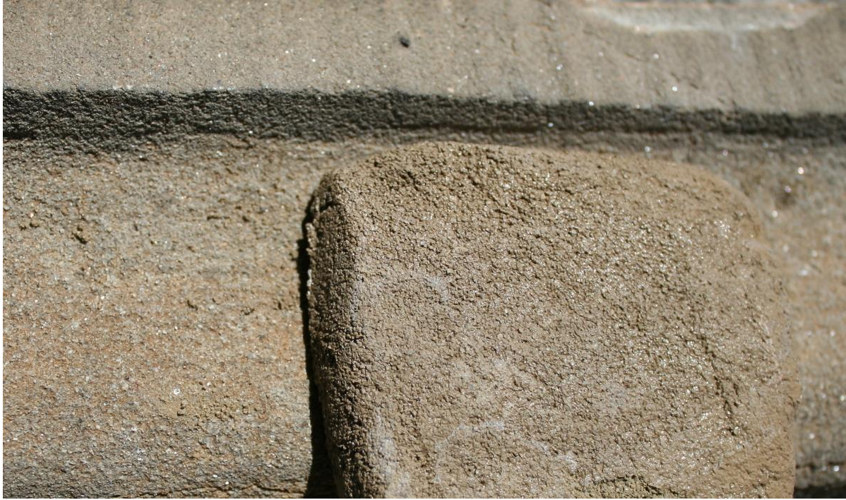
Image 10. Color match at heavily patinated stone with mortar sample TM-265C in sunlight.
