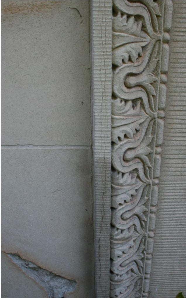
Image 2. Moistened crack prior to repair.
