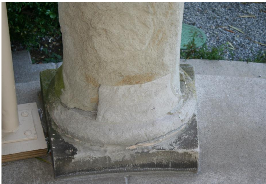
IMAGE 15. Detail of deterioration and previous Dutchman repair at column base.
