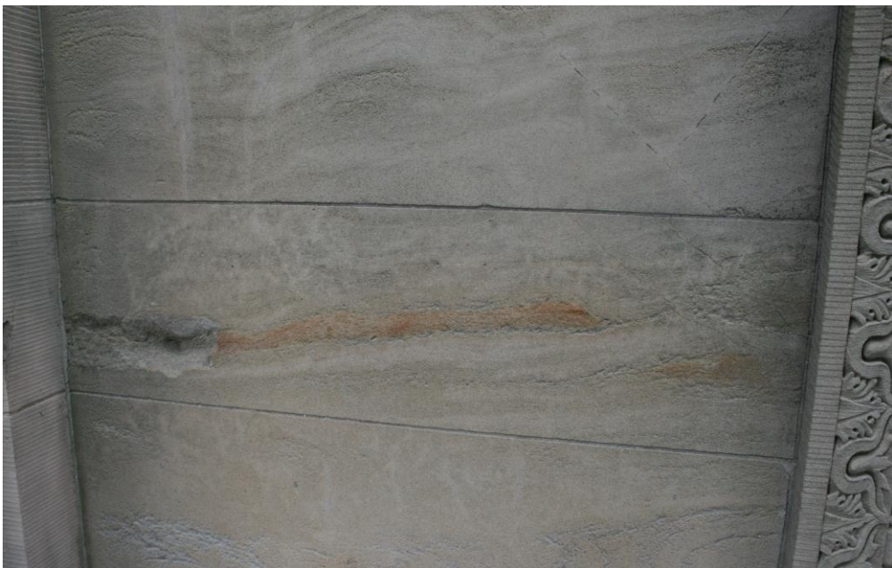
IMAGE 11. Spalling and delamination at ashlar masonry.
