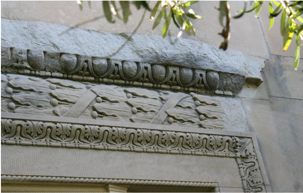
IMAGE 10. Detail of deterioration and material loss at decorative window surrounds.
