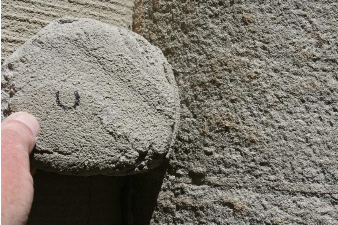
Image 12. Mortar color match of heavily weathered column at portico.
