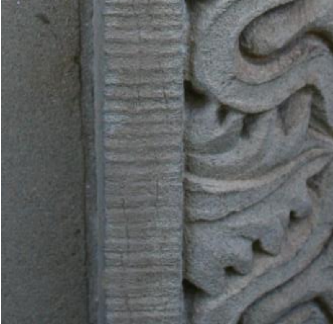
Image 5. Detail of hairline crack at decorative element after repair using color code TM-273C.
