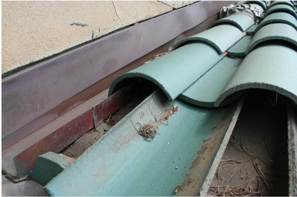
IMAGE 22. Detail of reglet installed in the mid to late 1990's at portico roof flashing.
