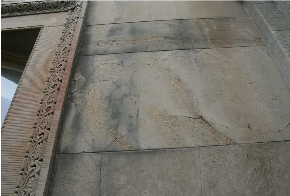
IMAGE 16. Delamination and hairline cracking at ashlar masonry.
