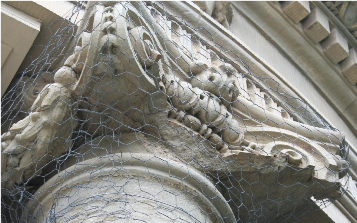
IMAGE 7. Detail of material loss at Portico Capital.
