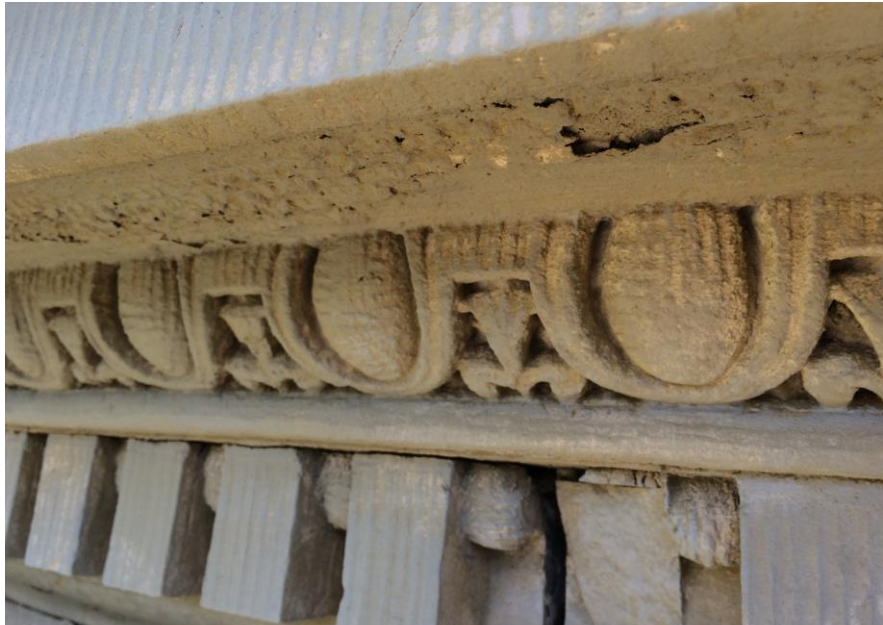
IMAGE 14. Detail of deterioration and coating at portico egg and dart.
