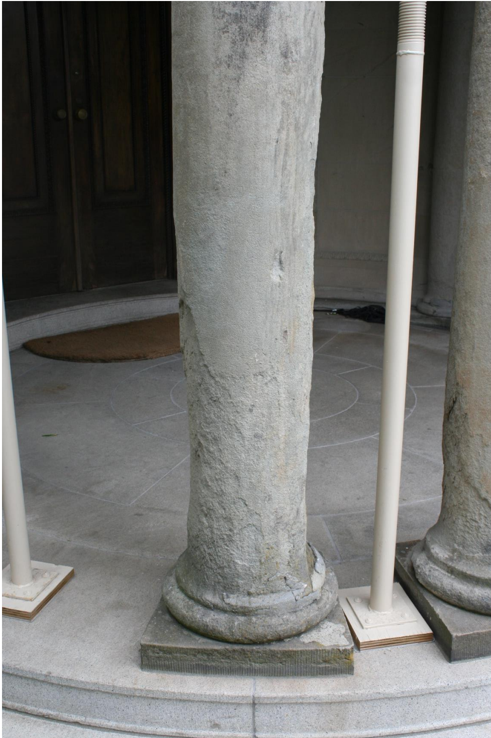
IMAGE 13. Detail of material loss and deterioration at at portico column, area where replacement is necessary.
