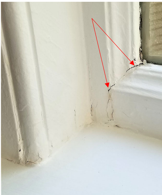
Figure 3 - Signs of water leakage at bottom rail corner.
