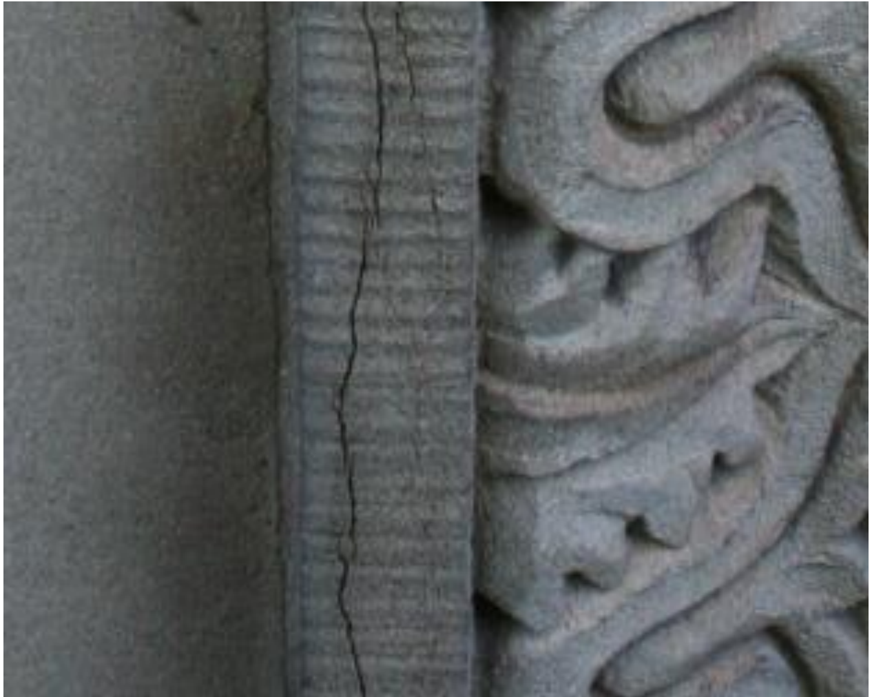
Image 4. Detail of hairline crack at decorative element prior to repair.
