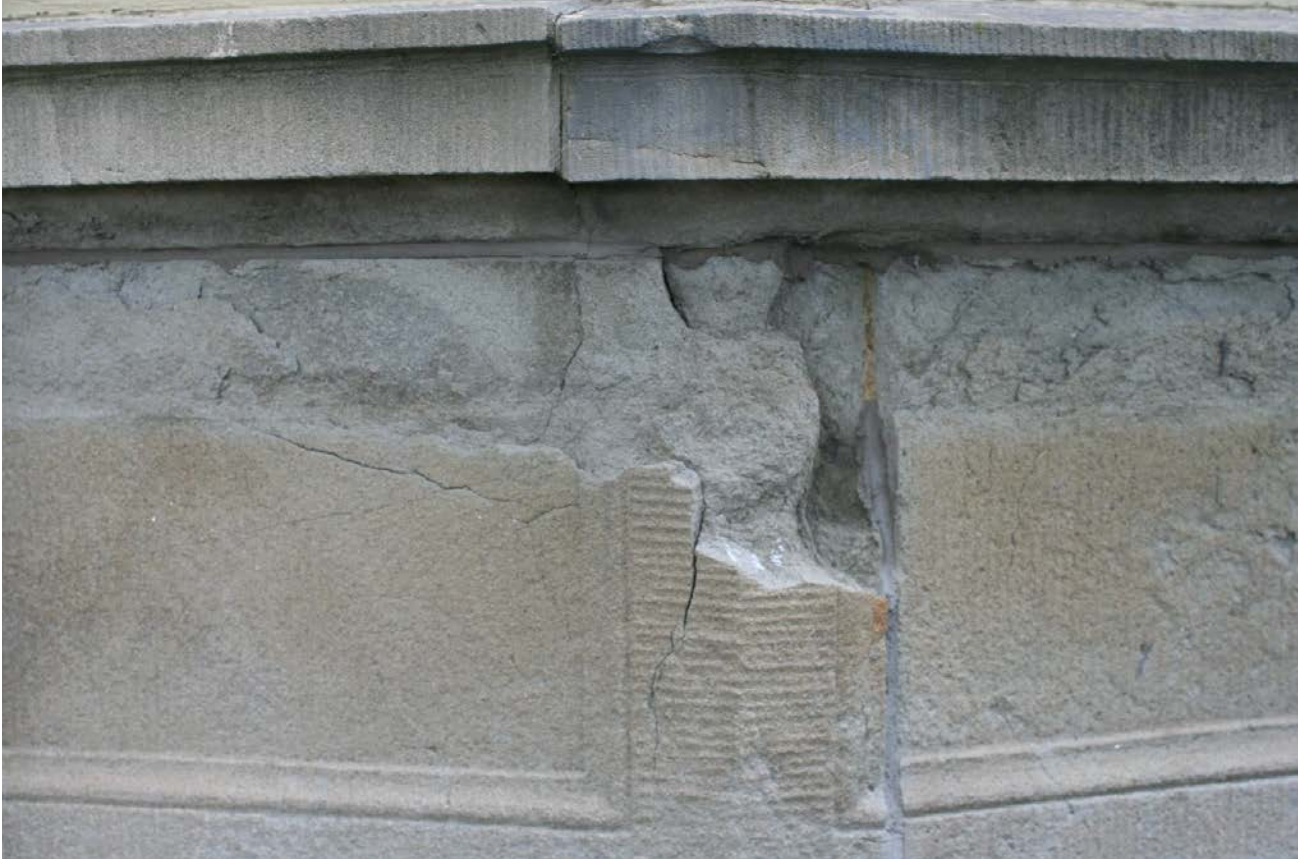
IMAGE 6. Detail of deterioration due to landscape irrigation and capillary action, area where dutchman repair is required.
