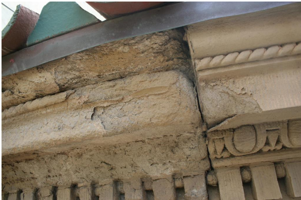
IMAGE 23. Detail of deterioration from previous waterproofing deficiencies.
