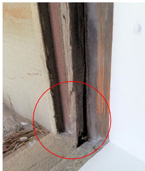
Figure 4 - Deterioration of parting bead.
