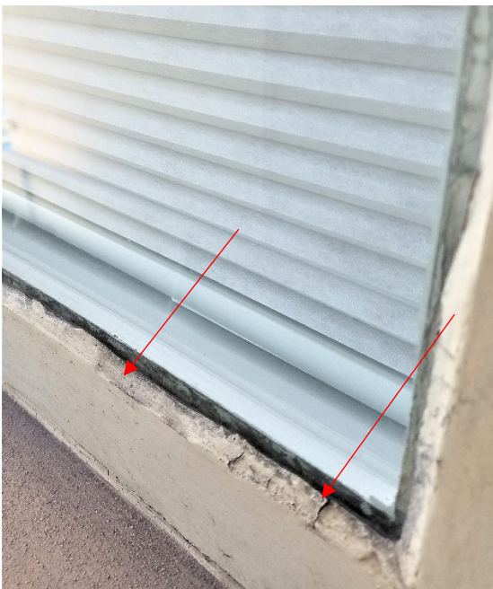
Figure 7 - Deteriorated putty at glazing.
