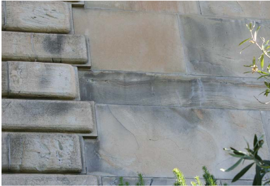
IMAGE 19. Environmental staining and delamination at ashlar masonry.
