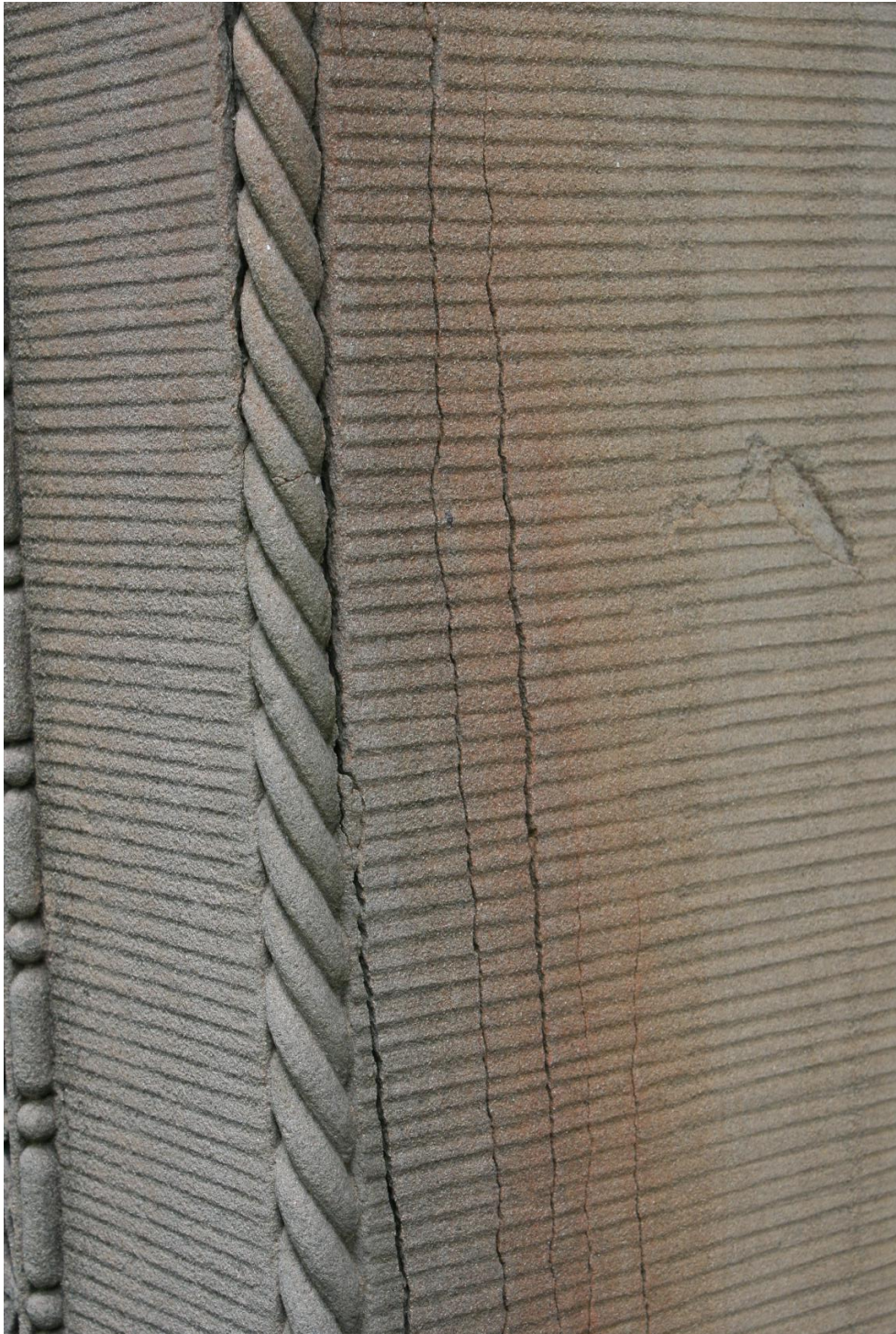
IMAGE 21. Detail of delamination at decorative fenestration surrounds.
