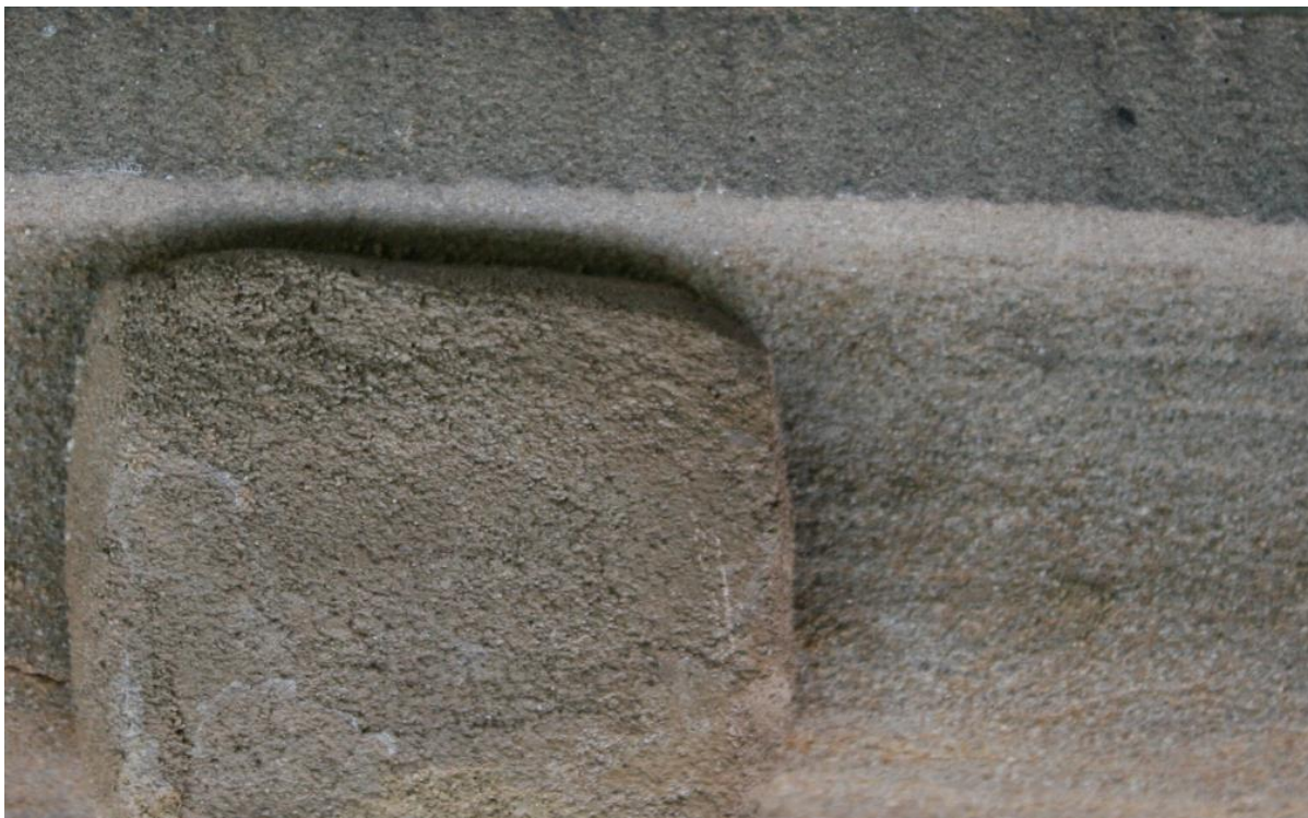
Image 11. Color match at heavily patinated stone with mortar sample TM-265C in shade.
