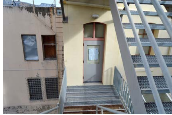
Figure 28: Typical steel door with upper lite and transom along rear (south) façade. Looking north from stairs.
