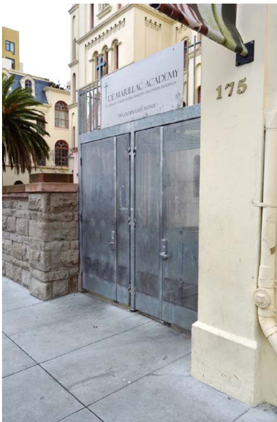
Figure 8: Steel gated entrance with steel mesh screen doors at east end of north façade. Looking southwest.
