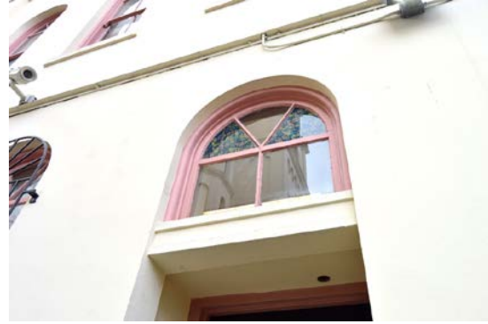
Figure 22: Arched transom with divided-lite glazing above main entry door. Looking west.
