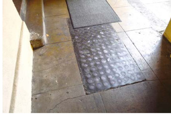
Figure 20: Rectangular glass vault lights along first story concrete pathway. Looking north.
