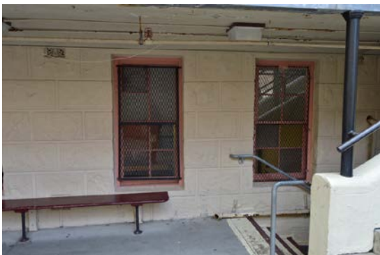
Figure 12: Four-over-four wood-sash basement windows with metal security screens. Looking west.
