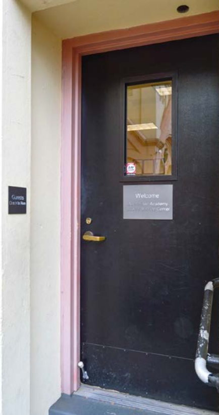
Figure 21: Replacement steel door at main entrance to subject building. Looking west.
