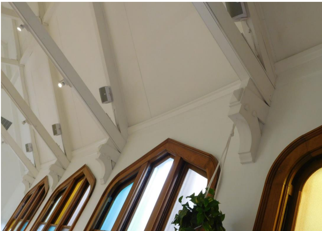
Figure 36. Corbels supporting the scissors trusses inside the former sanctuary; view toward southwest.
