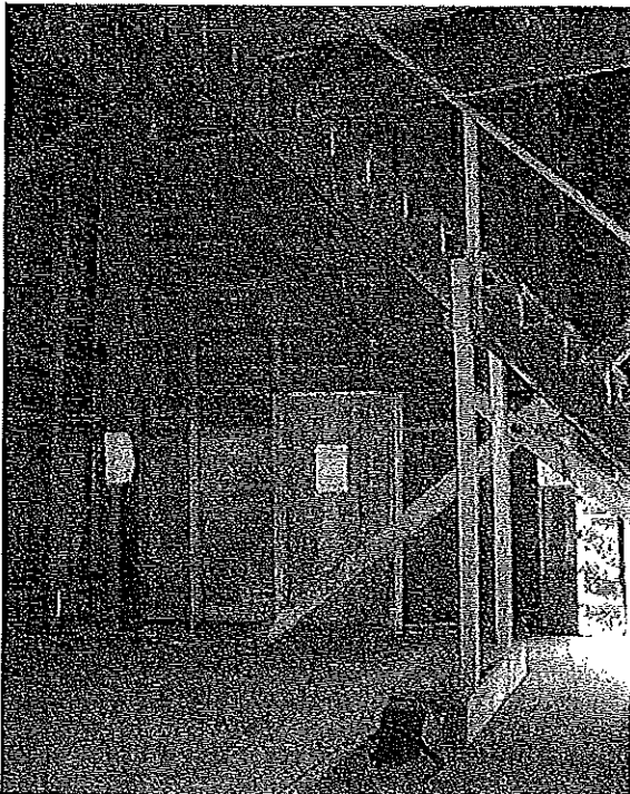
Figure 23: Water staining is visible on the wood cladding.
