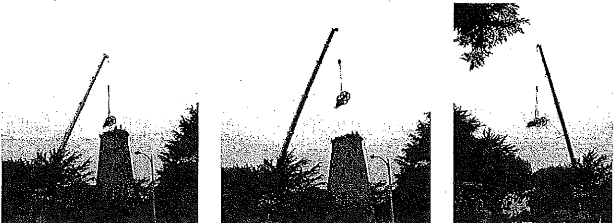
Figure 8: The removal of the cap and machinery, June 26, 2002.
