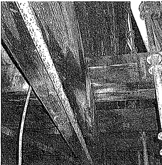
Figure 25: Dry rot has spread to structural members.
