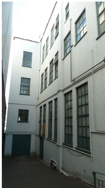
East elevation, view southeast.
