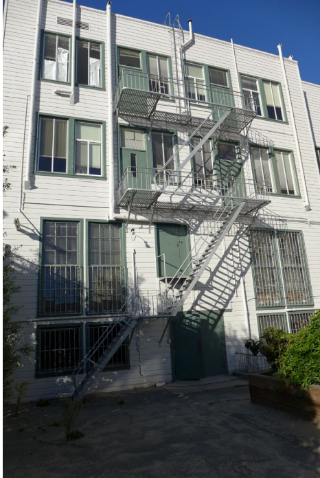
Rear (south) façade, view north.
