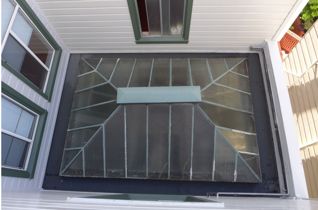
Skylight in light well at west elevation.
