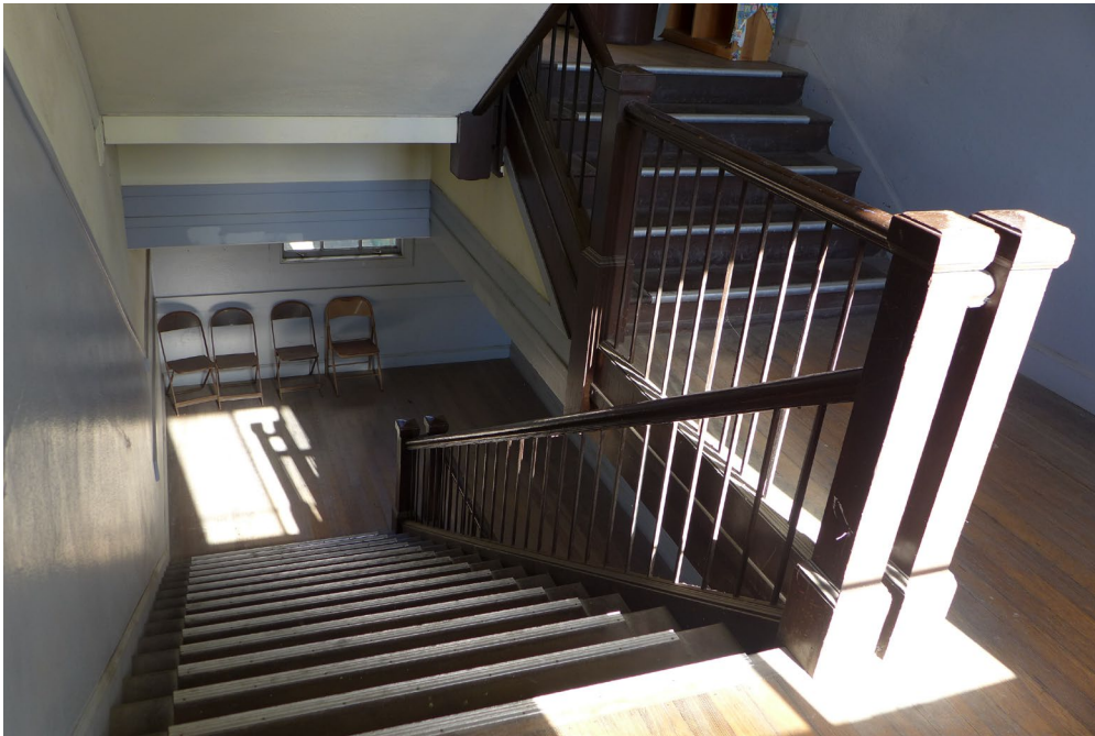
Dogleg, closed string wooden stairs with railing.
