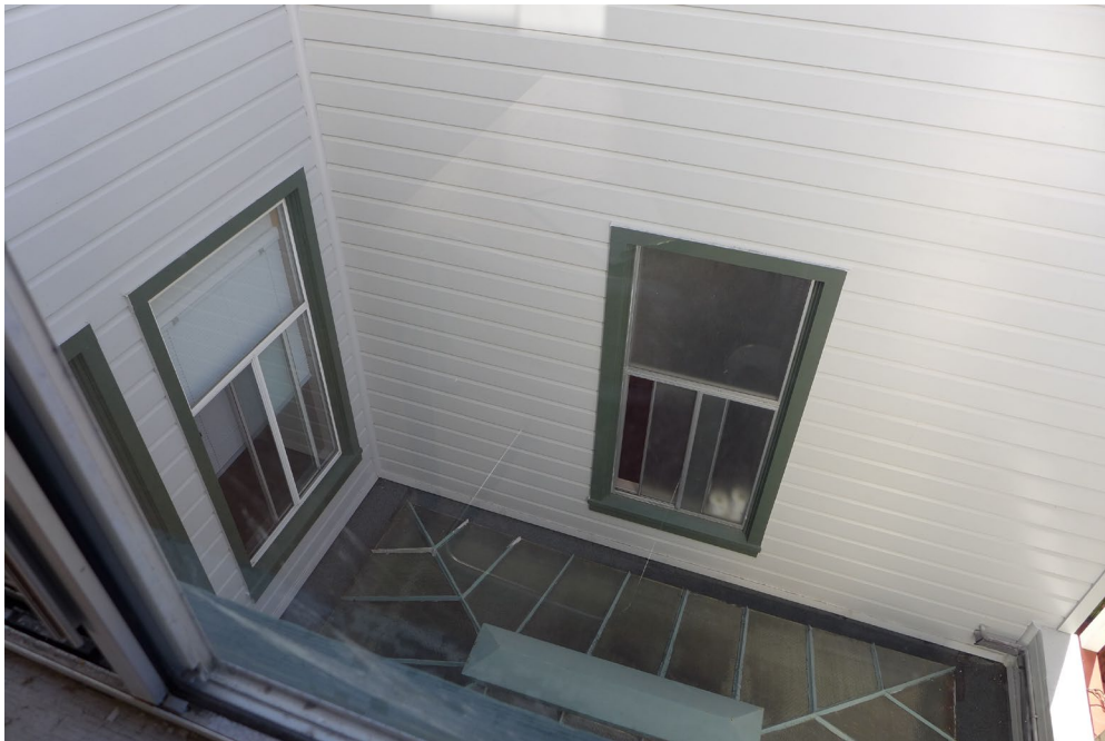
Light well at west elevation with view of skylight.
