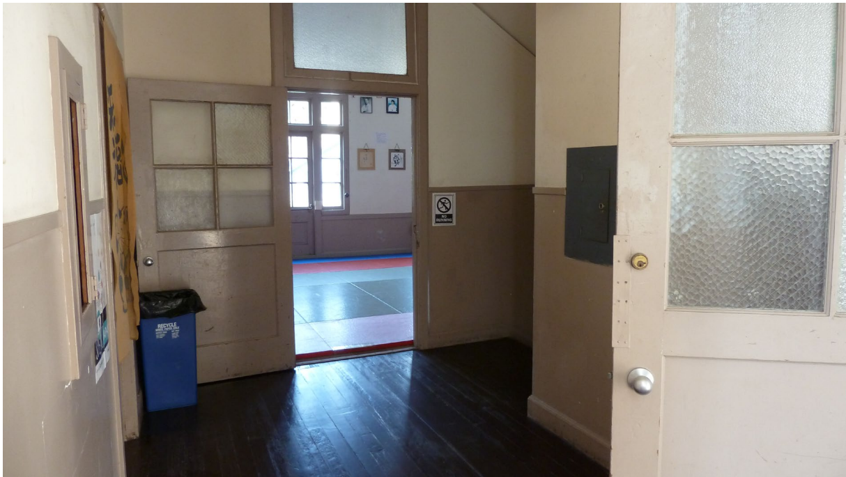
Entrance to classroom at north end of third floor.
