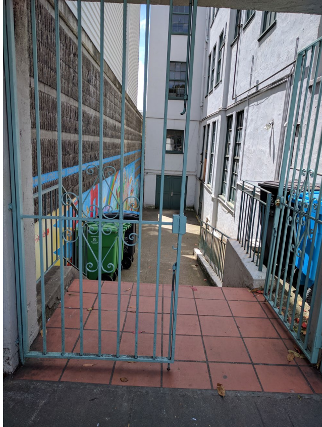
Wrought-iron entry gate leading to side yard at the eastern portion of building, view south.
