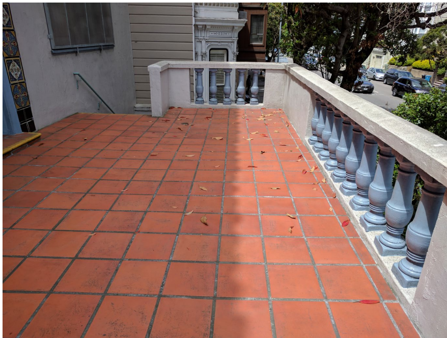
Terra cotta tile at the water table located at the second story of the entry stair, view west.
