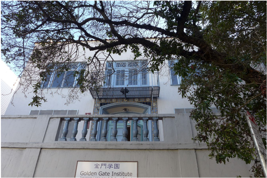
Primary (north) façade, view south.
