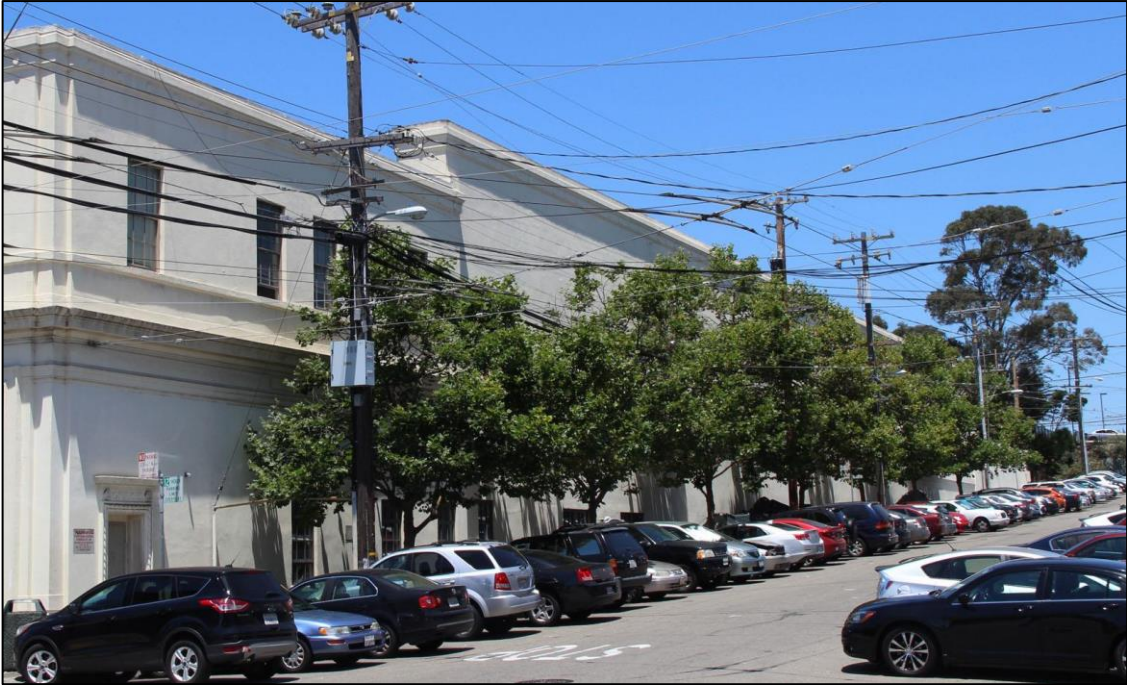
Figure 2: SFMTA Potrero Trolley Coach Division Facility, view northwest of east elevation facing Hampshire Street, (photo courtesy of HRE Part 1). The two story office wing connection is visible where the two parapet walls meet.
