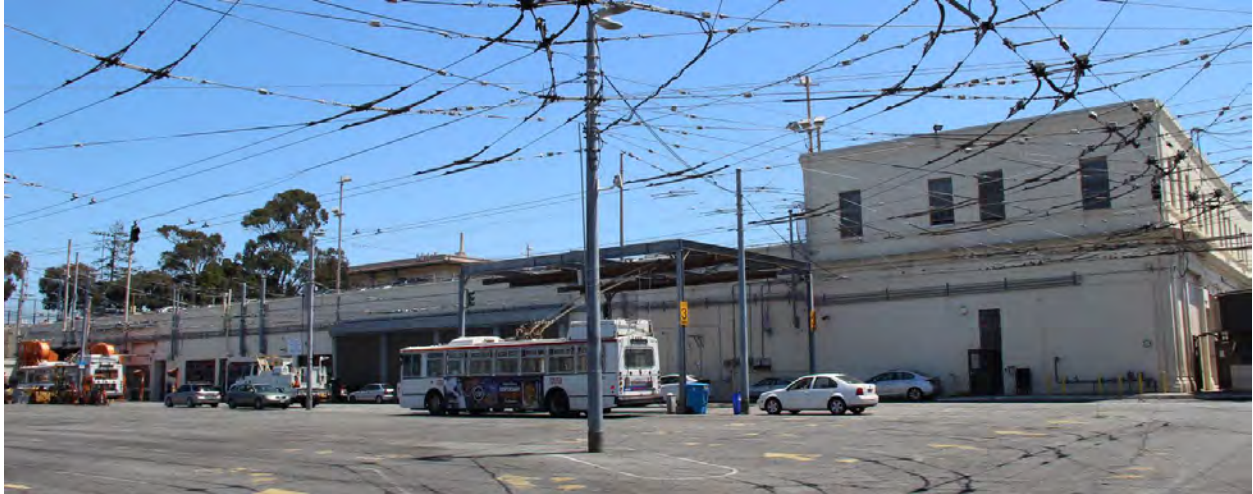
Figure 47. West façade of maintenance /operations building, looking northeast from bus yard.
