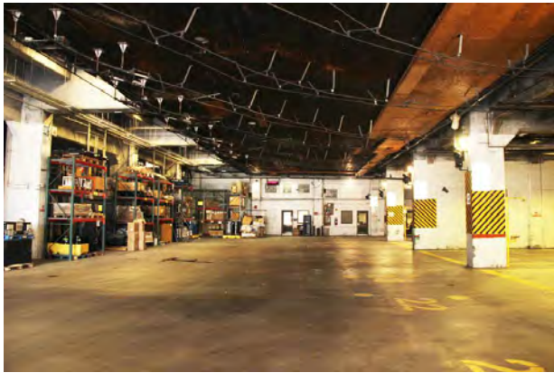
Figure 59. Storage rooms and driveway on north side of first floor level, looking east.
