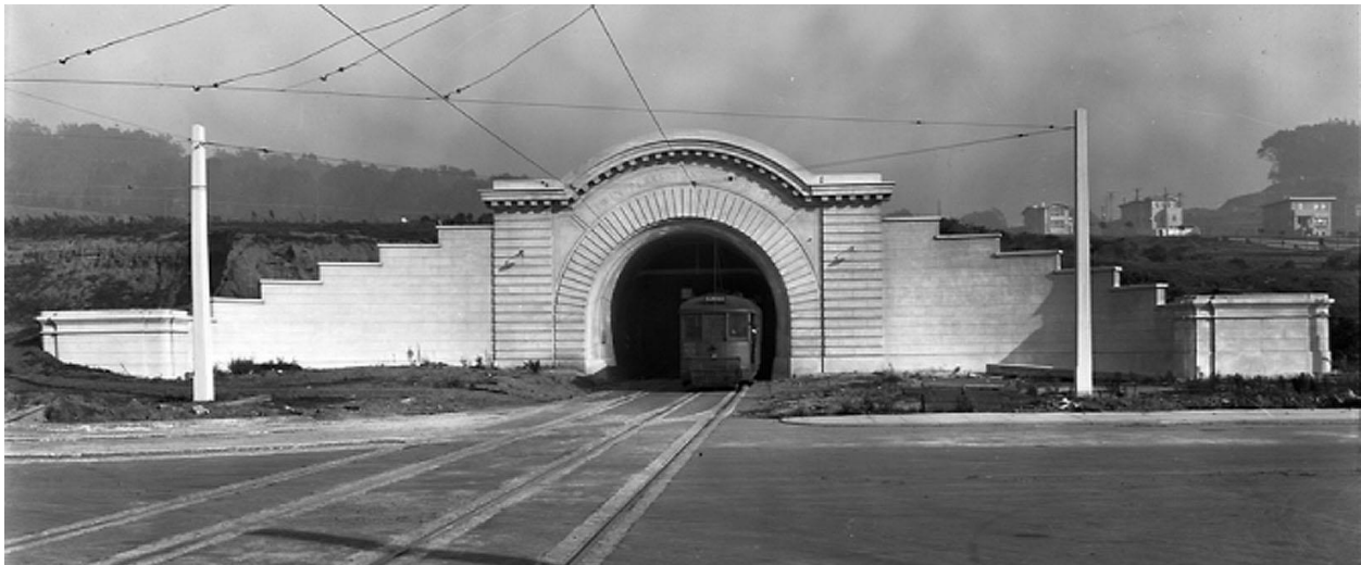
Figure 86. West Portal of Twin Peaks Tunnel, 1919.
