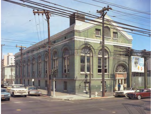
Figure 90. Turk and Fillmore Substation, 1966; built 1895. Source: SFMTA Photography Department and Archive, Image No. X9762_1
