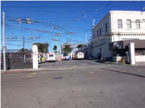
100_5702.JPG, 11/20/2007, view to N
