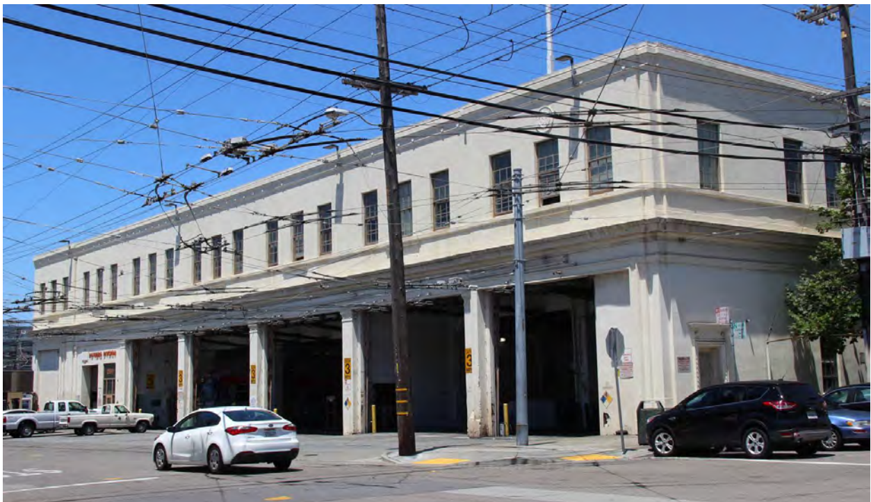
Figure 34. Primary façade of maintenance/operations building, looking northwest from Hampshire and Mariposa Streets.
