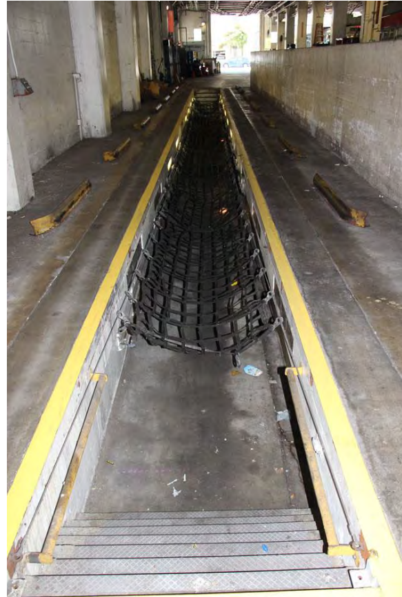
Figure 56. Maintenance pit, looking south.
