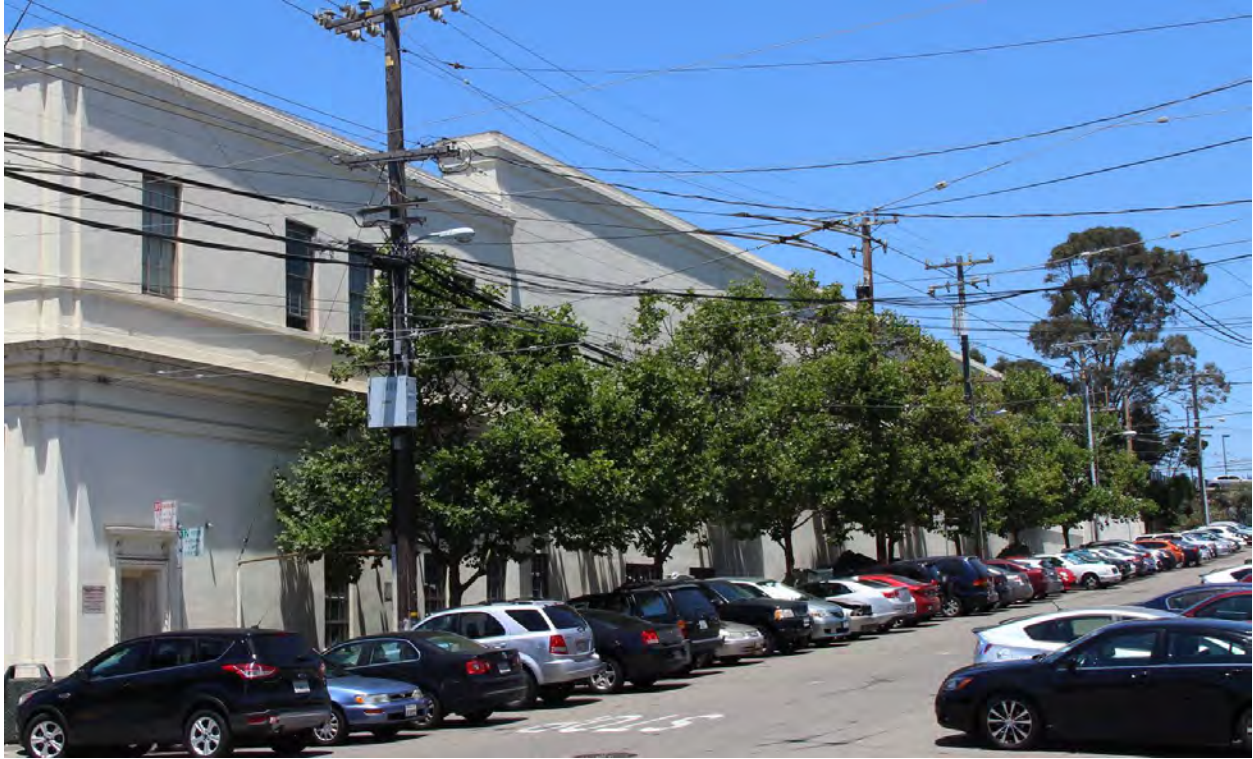
Figure 39. Secondary façade, looking northwest from Hampshire and Mariposa Streets.
