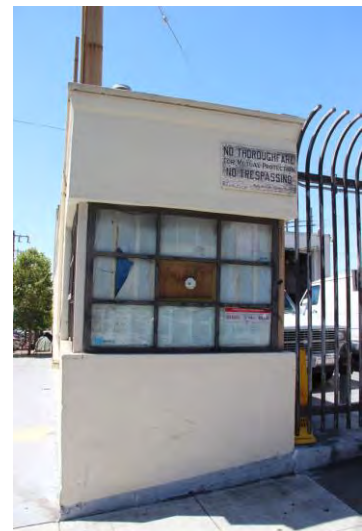
Figure 44. North wall of former control room
