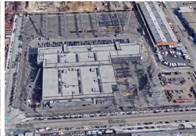
Figure 94. Muni Metro East Light Rail Center; view toward east.
