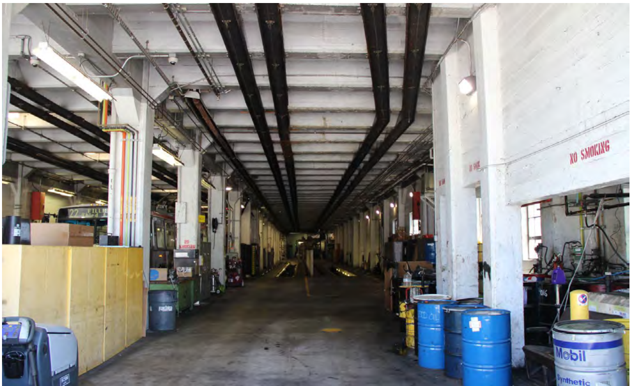
Figure 54. Detail of Bay 29, looking north.
