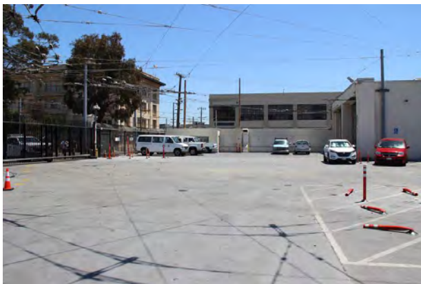
Figure 26. Parking deck, looking east.
