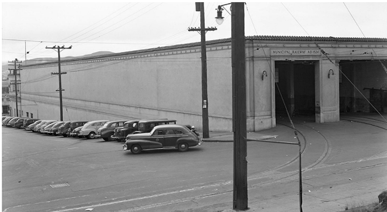
Figure 78. Hampshire and 17 th Street façades of Potrero Car House, November 16, 1948. Source: SFMTA Photography Department and Archive, Image No. D5486
