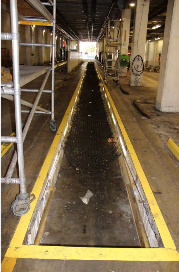
Figure 55. Maintenance pit, looking south.
