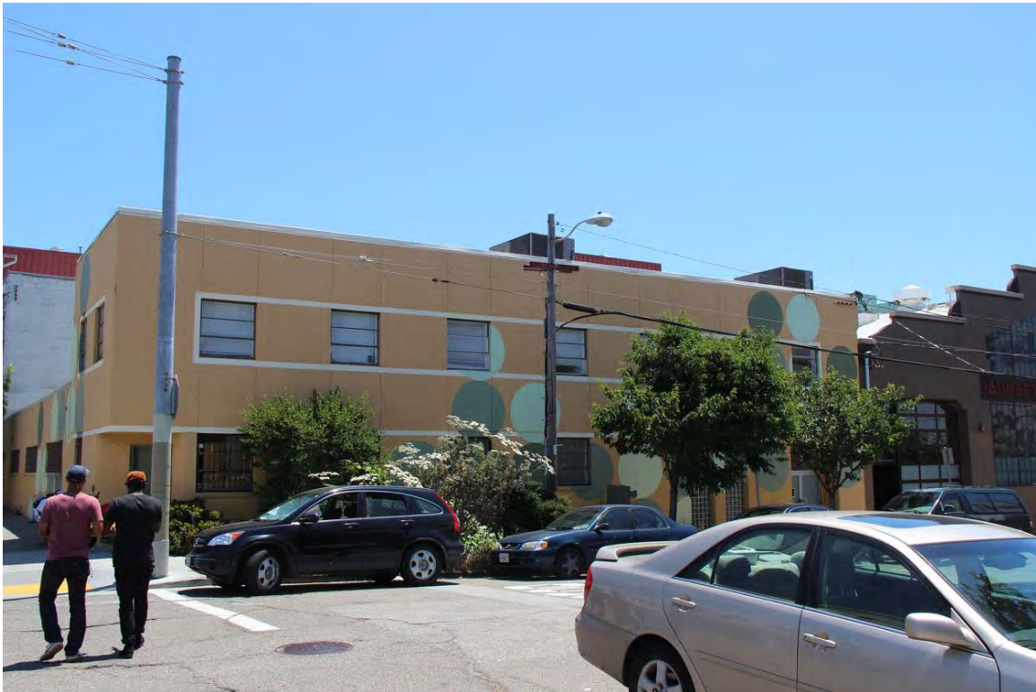
Figure 6. 501 York Street, looking southeast.
