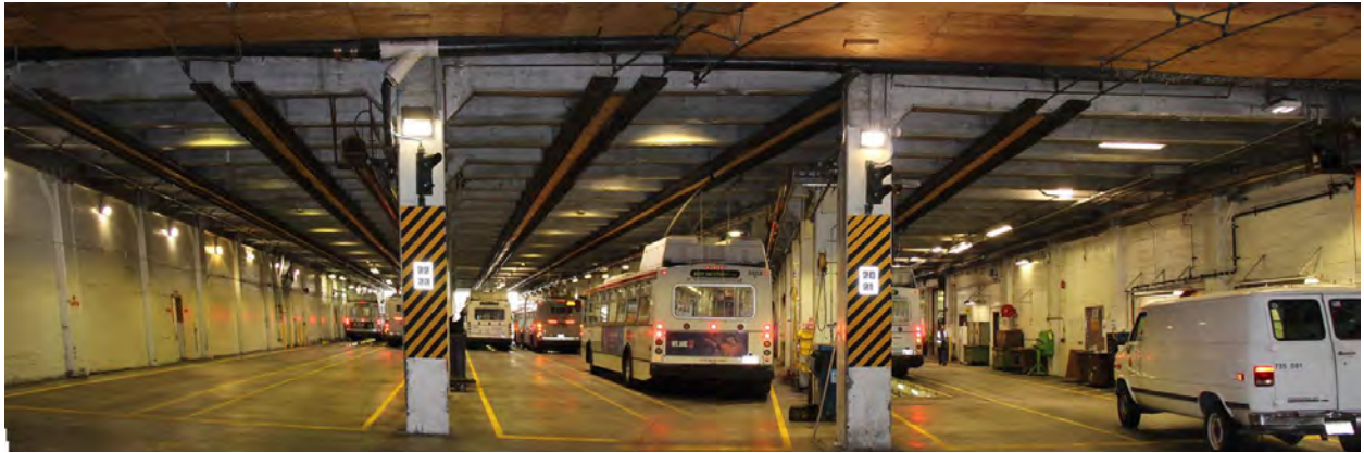
Figure 53. Maintenance bays, looking south.
