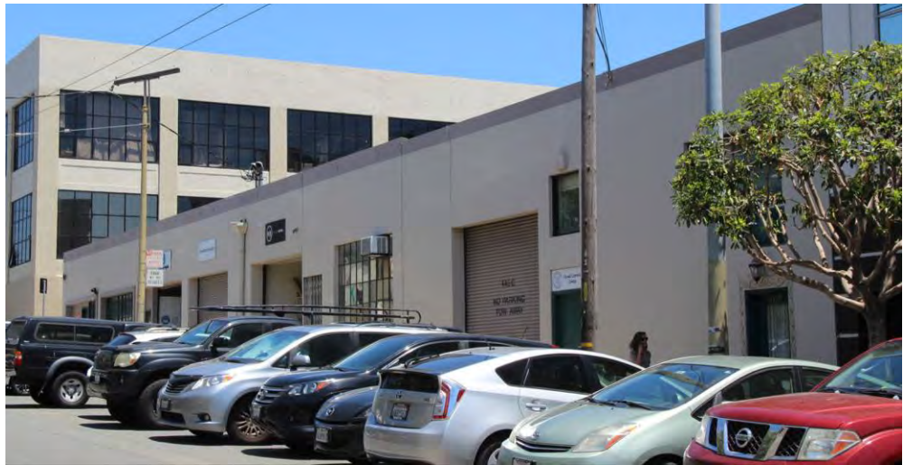
Figure 21. 445 Hampshire Street, looking northeast.
