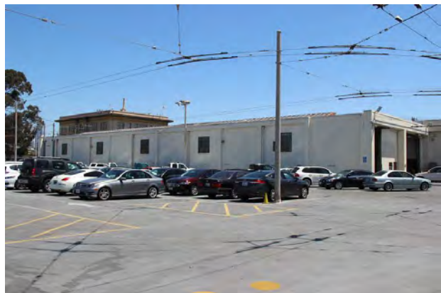
Figure 27. Parking deck, looking northeast.
