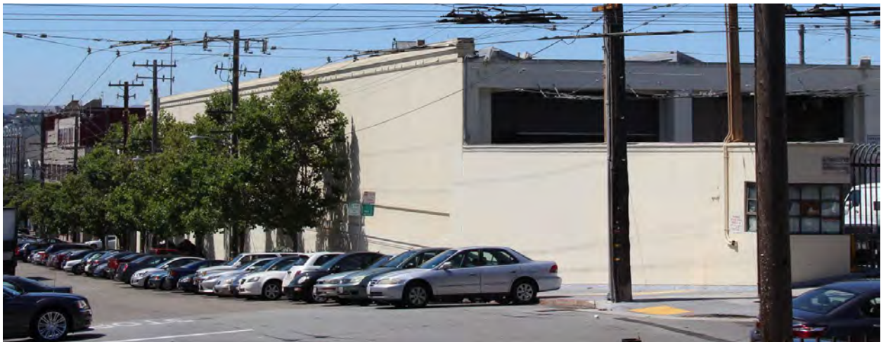
Figure 40. Secondary façade, looking southwest from Hampshire and 17 th Streets.
