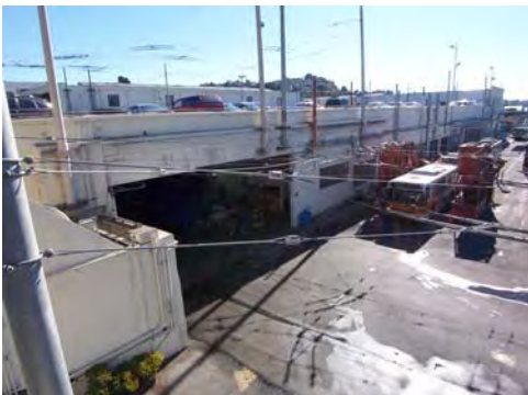
100_5696.JPG, 11/20/2007, view to E
