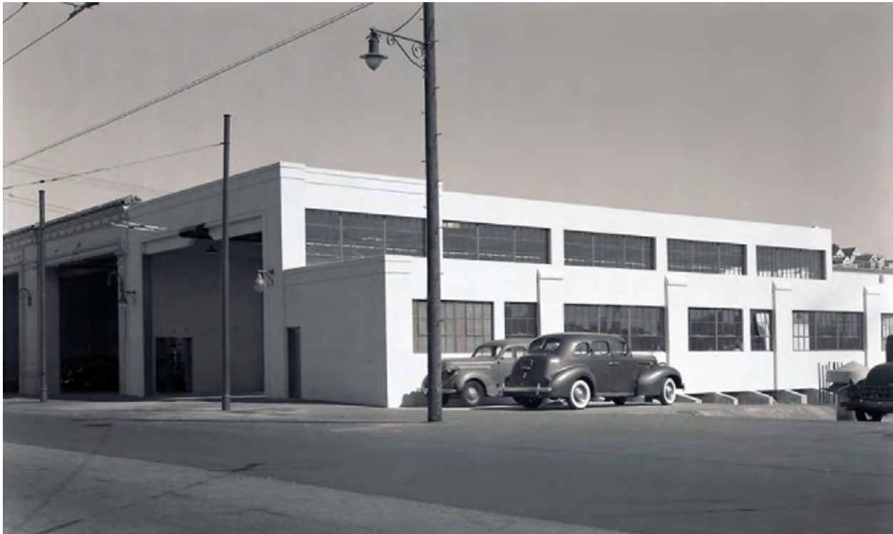
Figure 80. 1940-41 Trolley Coach maintenance shop addition to the Potrero Car Barn, August 25, 1941. Source: SFMTA Photography Department and Archive, Image No. D4675
