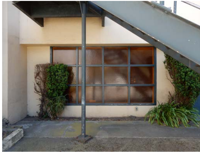
Multi-lite, wood sash windows with textured yellow glass at first floor, near northeast corner of north façade, view south.
