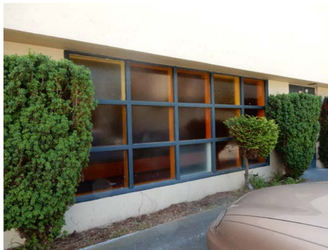
Multi-lite, wood sash windows with textured yellow glass at first floor, near northwest corner of north façade, view southwest.
