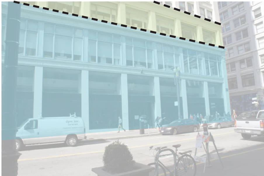
KMMS FACADE: TWO STORY STOREFRONT BASE, THIRD FLOOR MIDDLE EXPRESSION, TOWER TOP ABOVE
