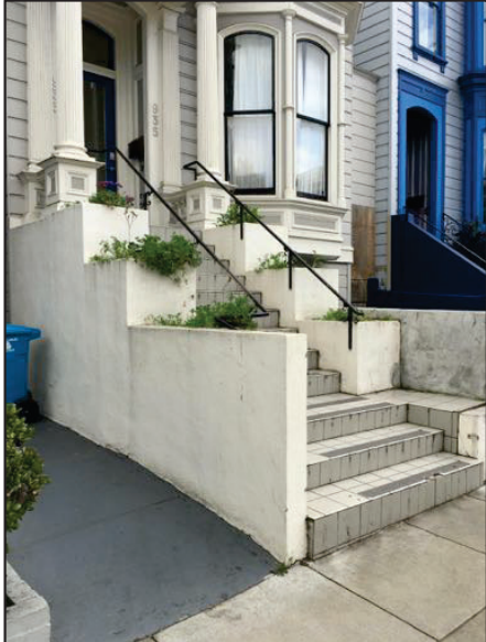
EXISTING STAIRS (AS SEEN FROM NORTH)
