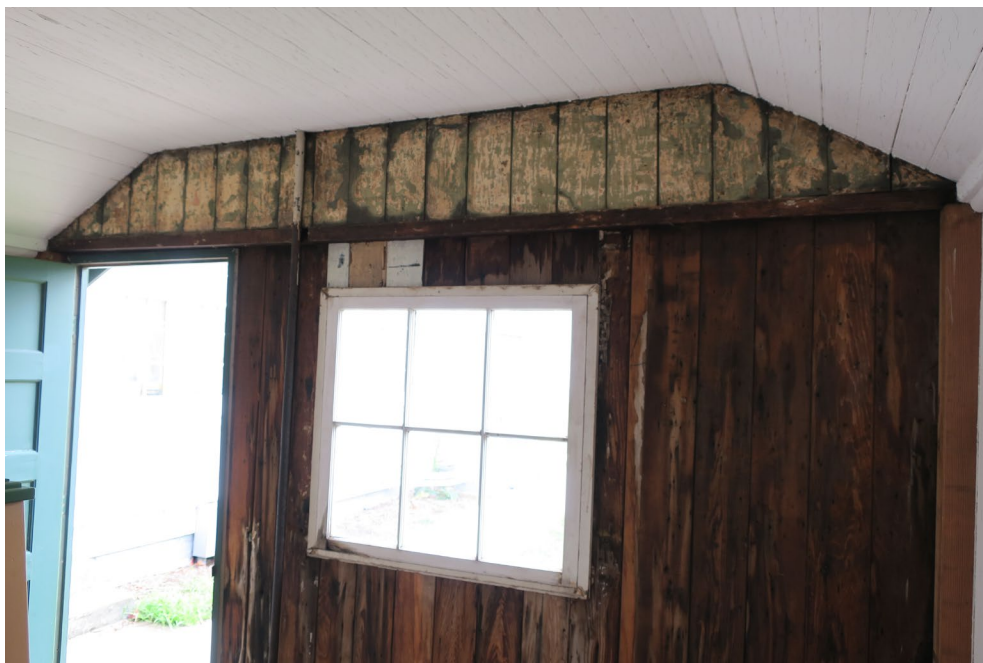
Fig. 25. Interior detail of the cove ceiling visible in one the Goldie Shacks at the Presidio. (Source: Arianna Urban.)
