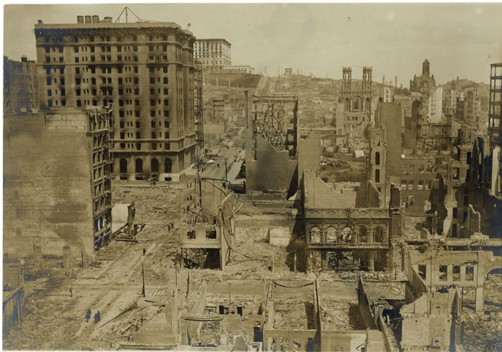
Fig. 1. The resulting fire caused widespread damage to the downtown business district. The structure of some steel frame buildings remained including the Saint Francis Hotel and the Fairmount Hotel in the distance.
