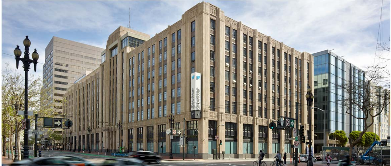
Figure 49. Western Furniture Mart, aka, the “Twitter Building.” Source: Page & Turnbull, Inc.
