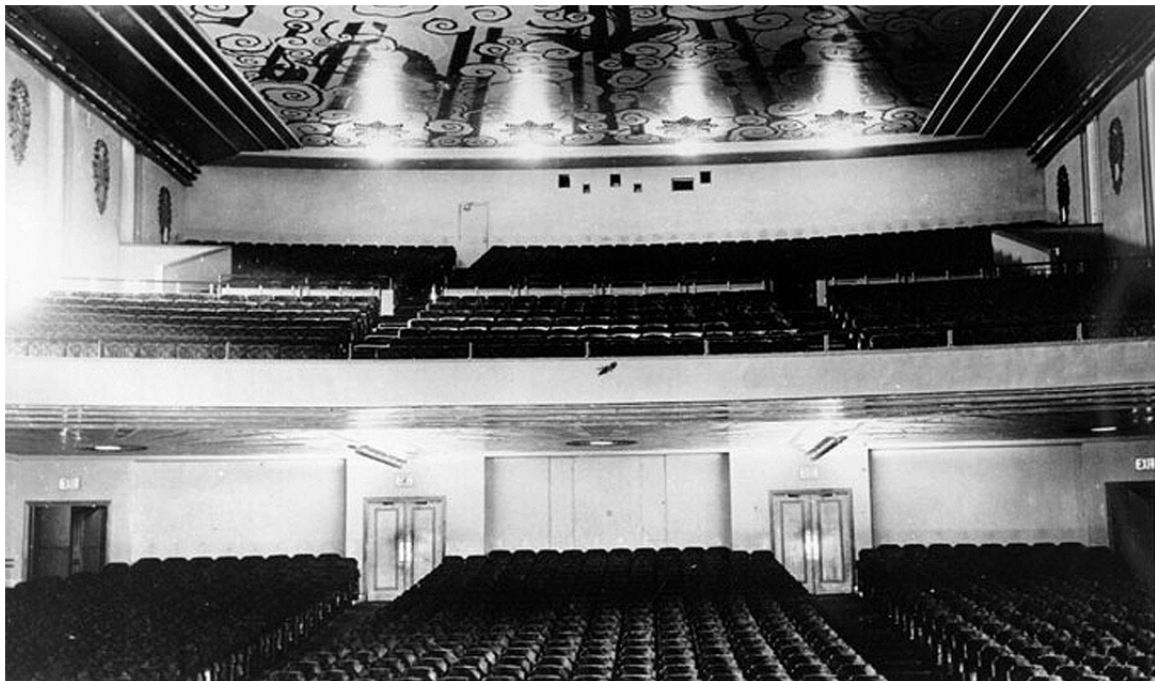
Figure 32. El Rey Theater Auditorium, looking south, 1942.
