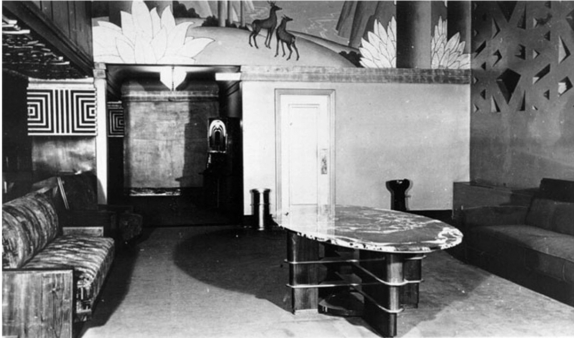
Figure 31. El Rey Theater Mezzanine Lounge, looking east, 1942.
