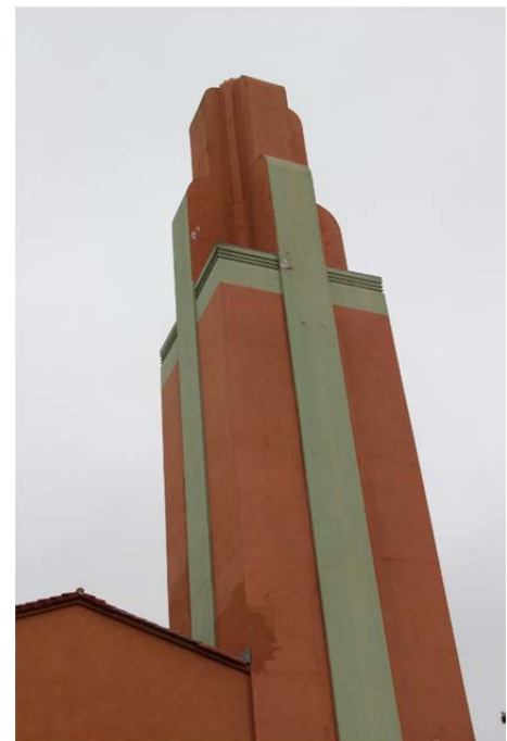
Figure 10. Tower. Source: Christopher VerPlanck
