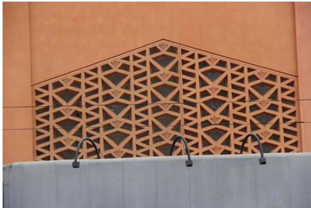
Figure 8. Concrete grille above main entrance. Source: Christopher VerPlanck
