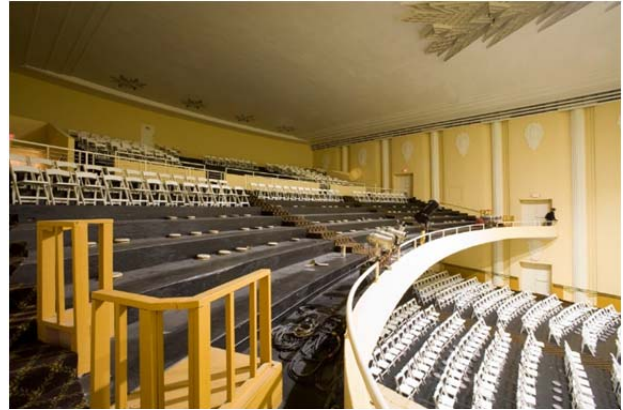
Figure 23. Balcony, looking southwest. Source: Tom Paiva
