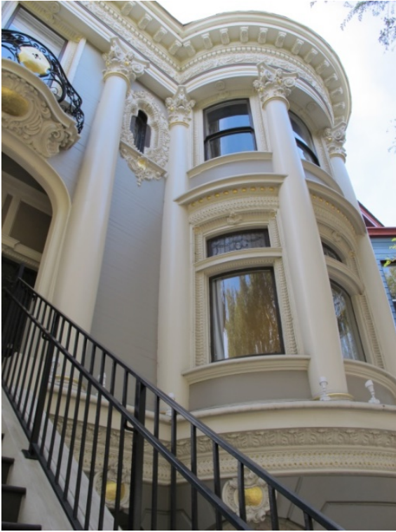
Figure 12: Double height Corinthian engaged columns.
