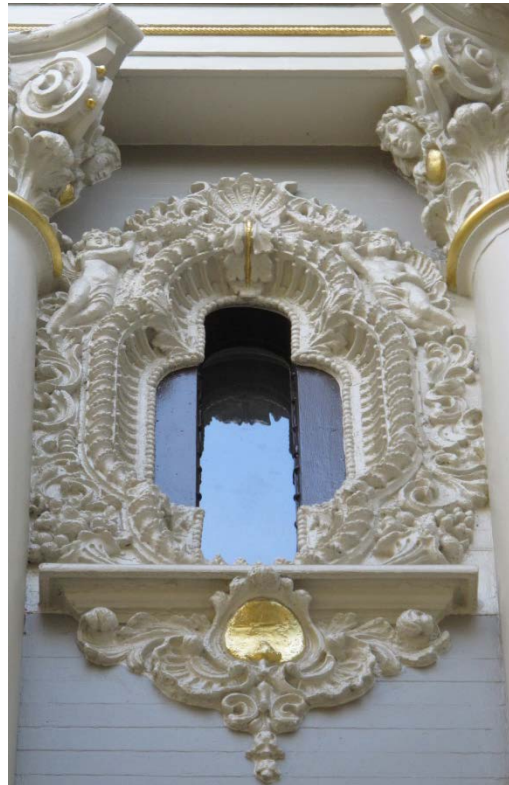
Figure 17: Vertically elongated quatrefoil surround with oval pane (north of turret).
