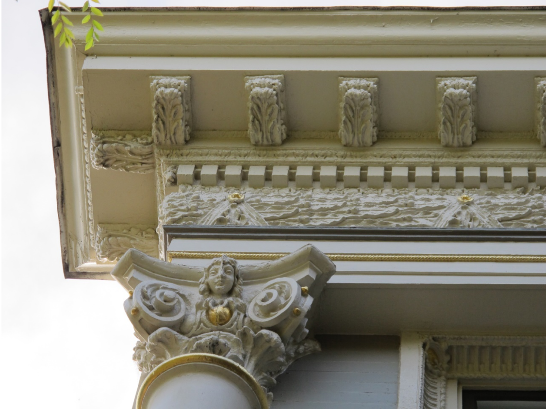
Figure 19: Entablature detail.
