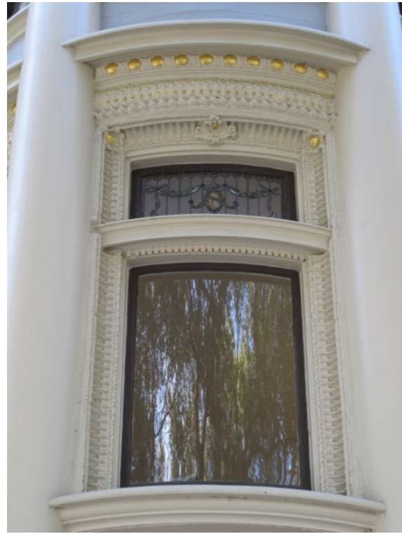
Figure 13: Second story rounded bay window with transom.
