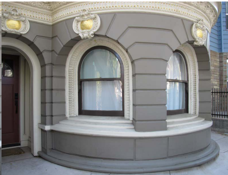
Figure 6: Ground level rounded bay base.
