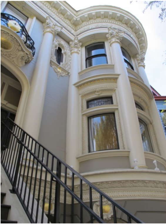
Figure 12: Double height Corinthian engaged columns.
