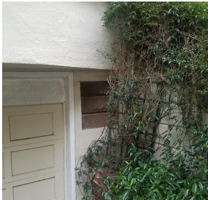
Exploratory demolition showing horizontal wood siding near garage.
