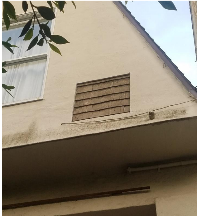
Exploratory demolition showing wood shingles at the gable.
