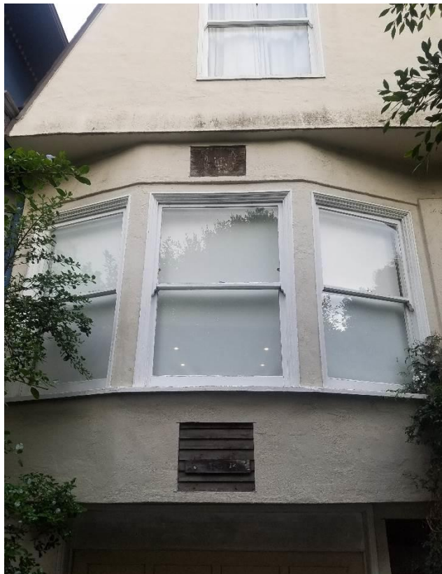
Exploratory demolition revealing flat wood fascia and horizontal wood siding.
