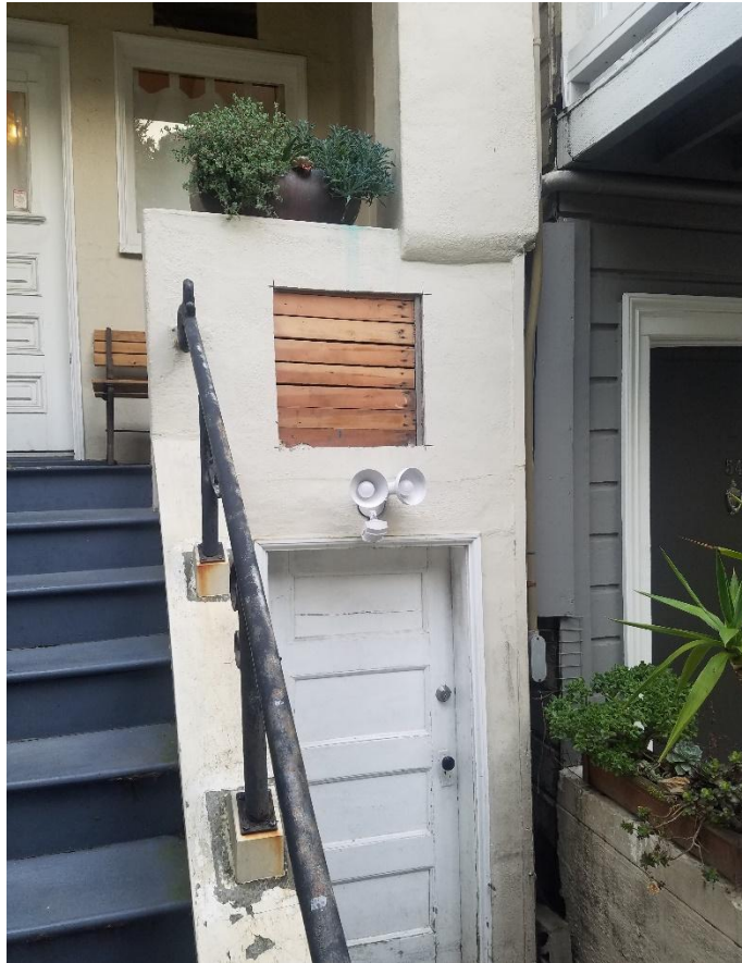
Exploratory demolition at front porch railing
