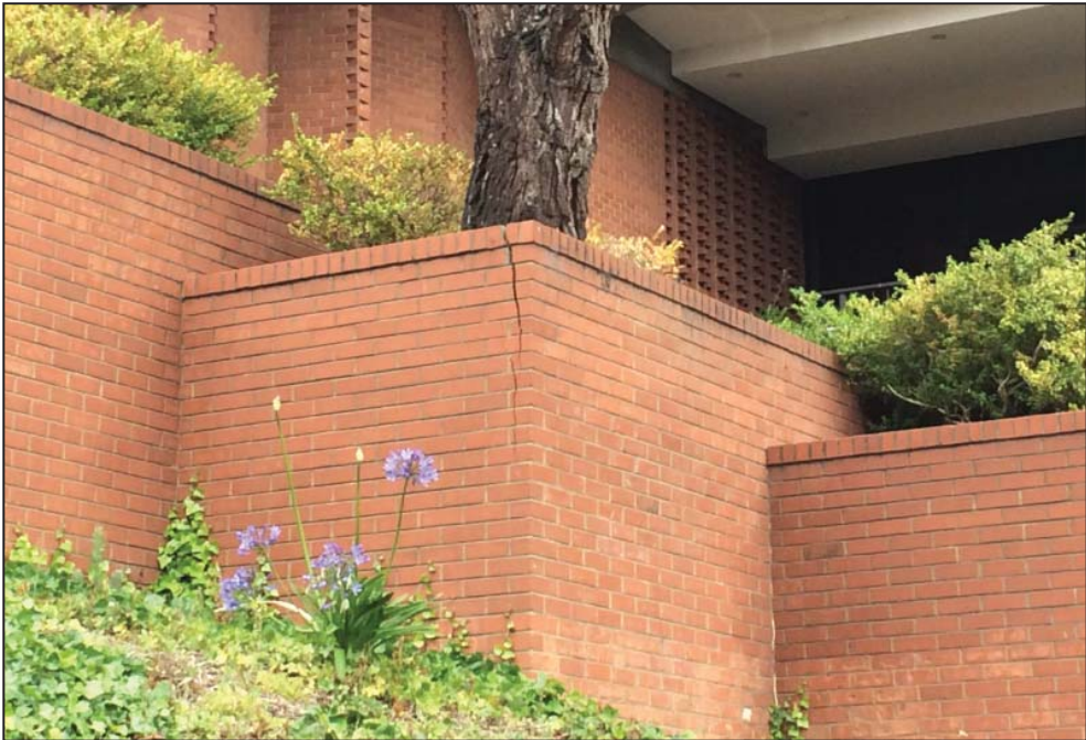
4. Brick perimeter walls, integrated planter boxes, and retaining walls of reinforced concrete and clad in stretcher bond pattern
