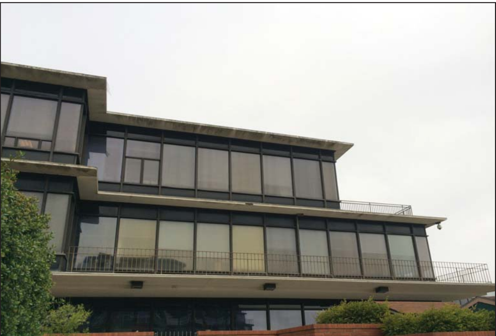
3. Midcentury Modern architectural style with little ornamentation 4. Flat, cantilevered roof with projecting eaves 5. Continuous full-height, slightly recessed curtain wall glazing on most sides and along all levels of the building
