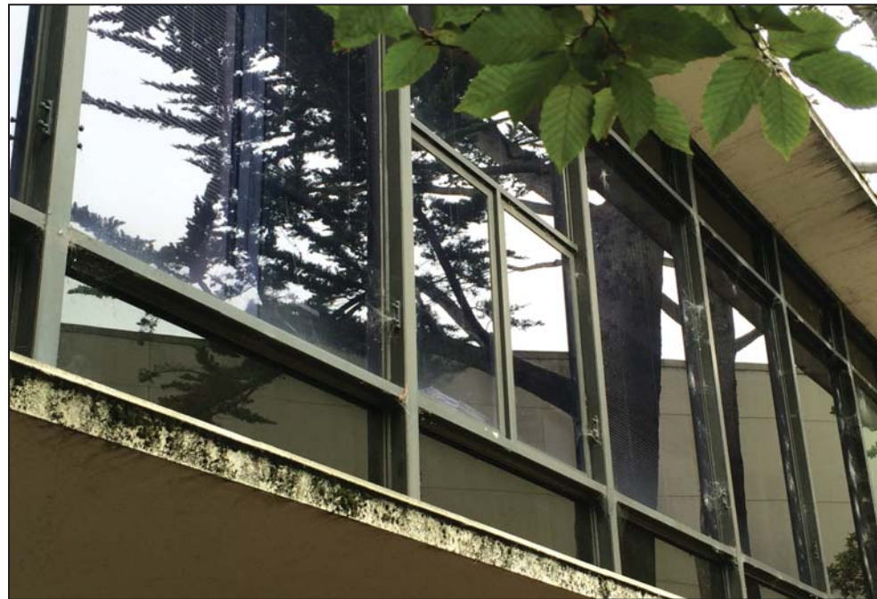
6. Glass curtain wall composed of bronze powder-coated aluminum framing system in a regularly spaced pattern of mullions and muntins, typically with a small spandrel panel of obscure glass below a larger pane.
