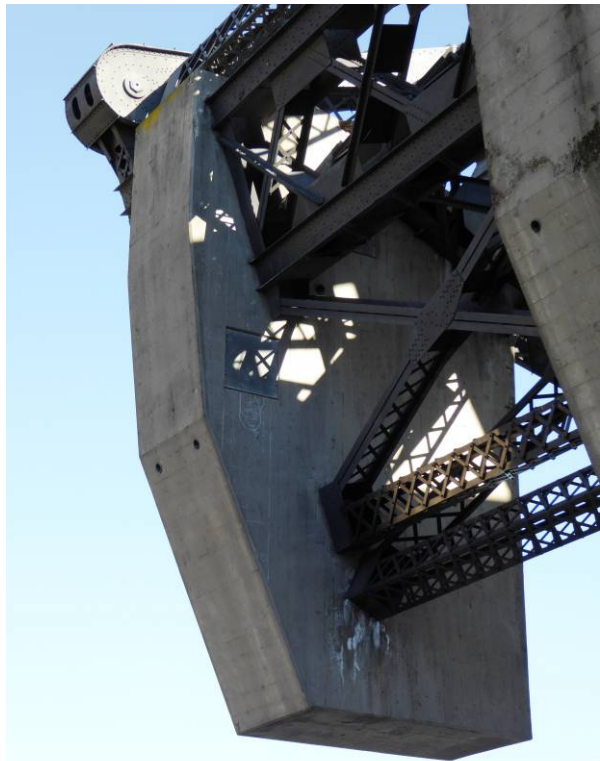
Photograph 20: East concrete counterweight; facing southeast.
