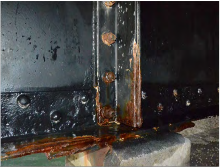
Floor beam 12 (@ location with 1975 retrofit blocks) EXAMPLE OF REPAIR WORK
