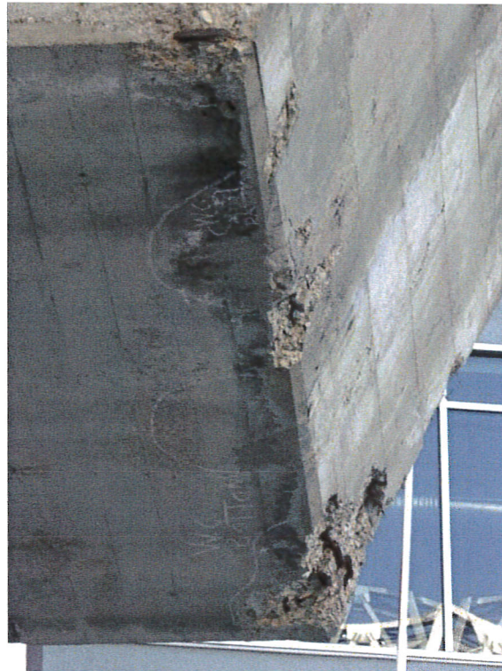
Photograph 26: West concrete counterweight showing deterioration on bottom corner; facing west.
