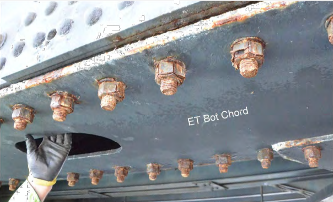
Bottom of bottom chord of the east truss EXAMPLE OF REPAIR WORK (NOTE THAT FASTENERS WILL BE REPLACED)
