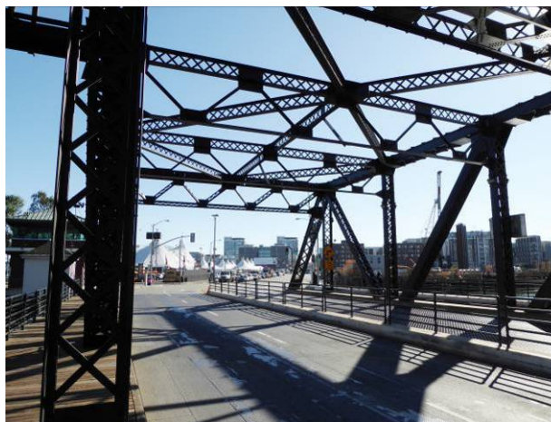
Photograph 4: Showing steel through truss and steel deck with composite surface with decorative plank design on northbound lanes; facing southwest.
