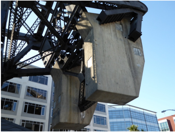
Photograph 17: Concrete counterweights; facing west.
