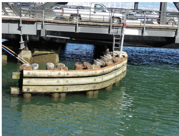
Photograph 30: Wood fender and piles on northwest corner of bridge; facing east.
