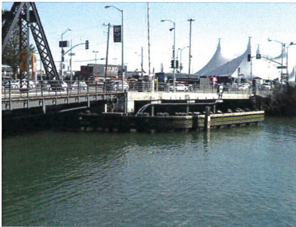
Photograph 35: Wood fenders and piles on southwest corner of bridge; facing south.
