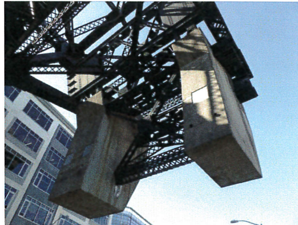
Photograph 18: Concrete counterweights facing northwest.
