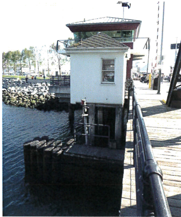
Photograph 34: Watchman's House, showing concrete piles and wood fender piles in foreground; facing south.
