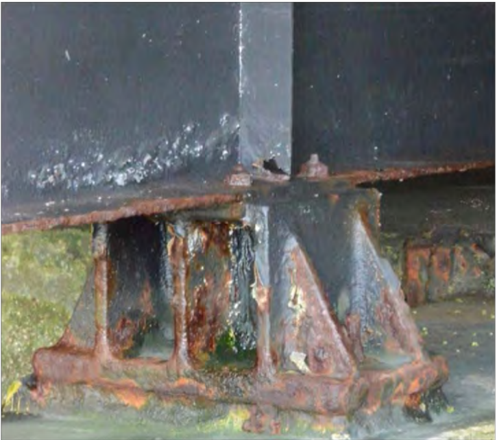
Steel bearing on top of Pier 2 EXAMPLE OF REPAIR WORK
