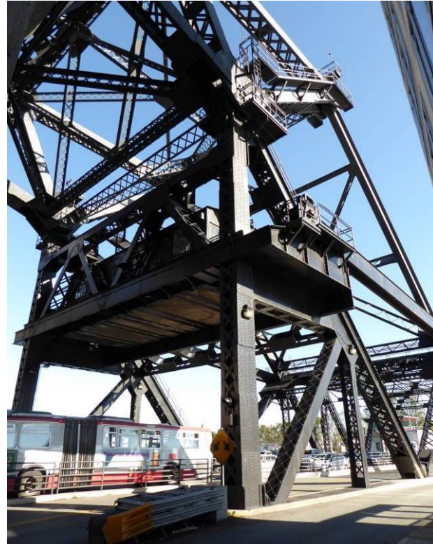
Photograph 10: Trunnion section of bridge including north side of Machinery Room; facing southeast.
