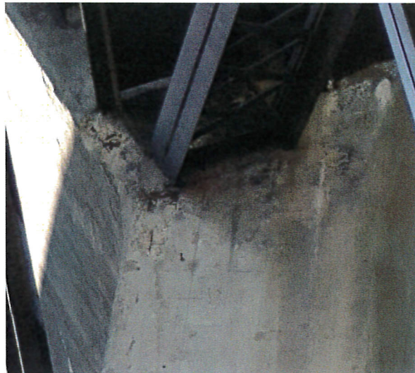
Photograph 22: West side of east counterweight showing deterioration near top where attached to girder on bottom corner; facing east.
