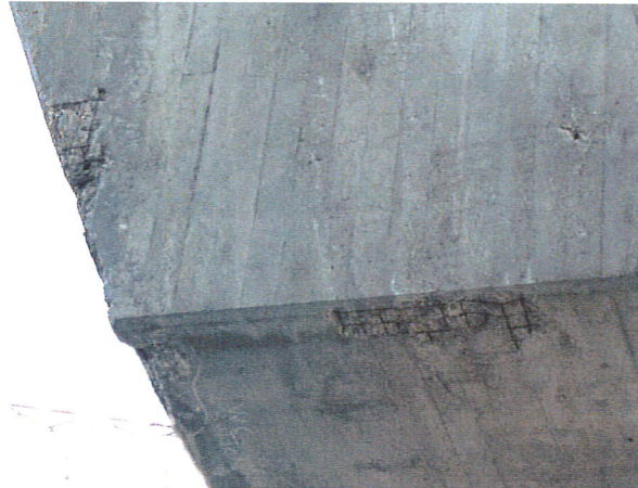
Photograph 30: West side of west counterweight showing deterioration on side and bottom; facing east.
