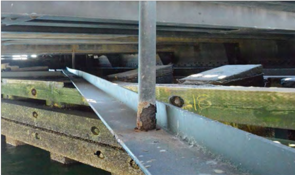
Hanger rod and sleeve near south fender system EXAMPLE OF REPLACEMENT WORK
