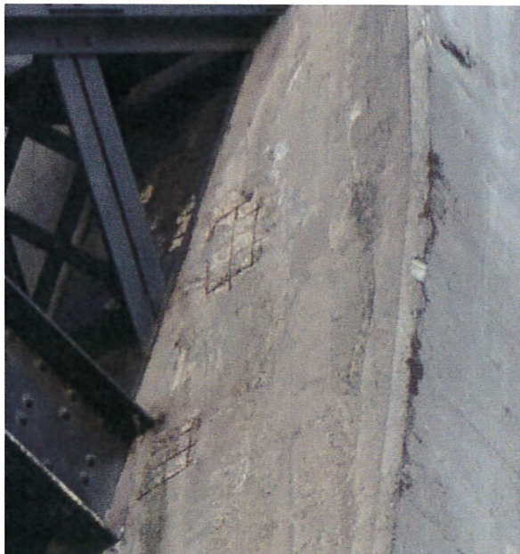
Photograph 28: East side of west counterweight showing exposed metal mesh near top where attached to girder; facing southwest.
