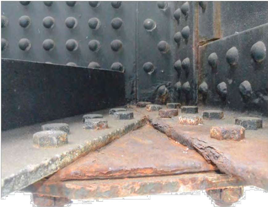
Top of gusset plate connecting floor beam, bottom chord and lateral brace EXAMPLE OF REPAIR WORK
