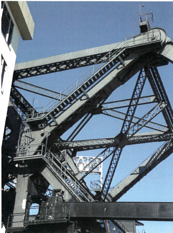
Photograph 13: First link pin (upper right) and counterweight trunnion (center left); facing west.
