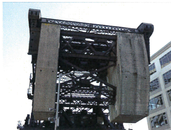
Photograph 16: Concrete counterweights; facing south.
