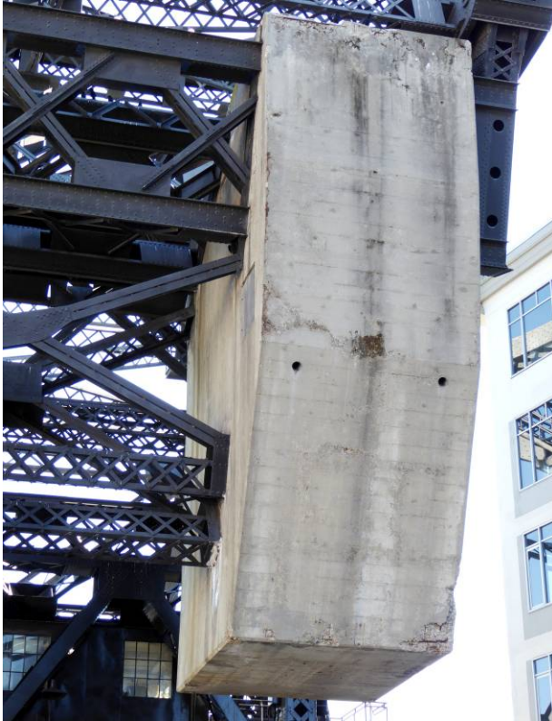
Photograph 21: West concrete counterweight; facing south.
