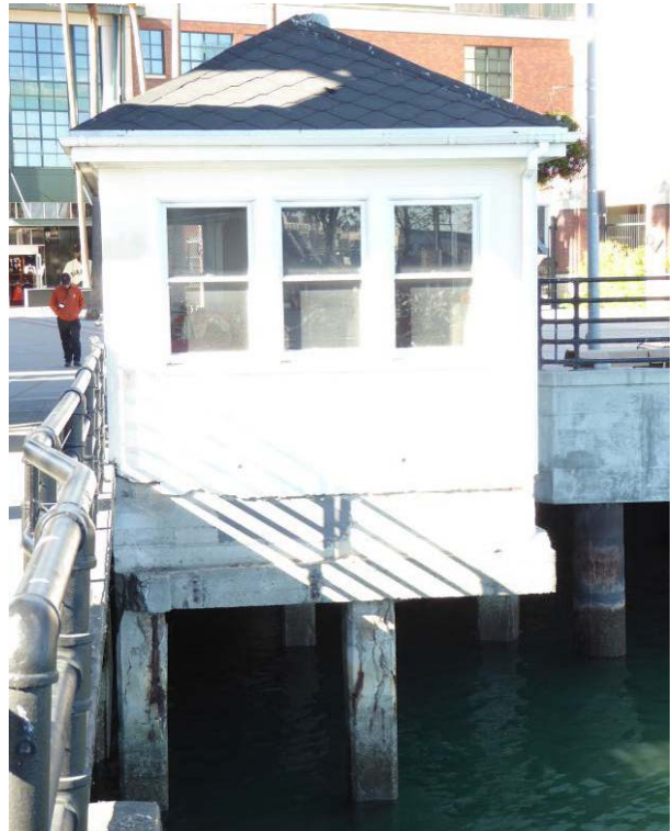
Photograph 26: Operator's House, showing concrete piles; facing north.
