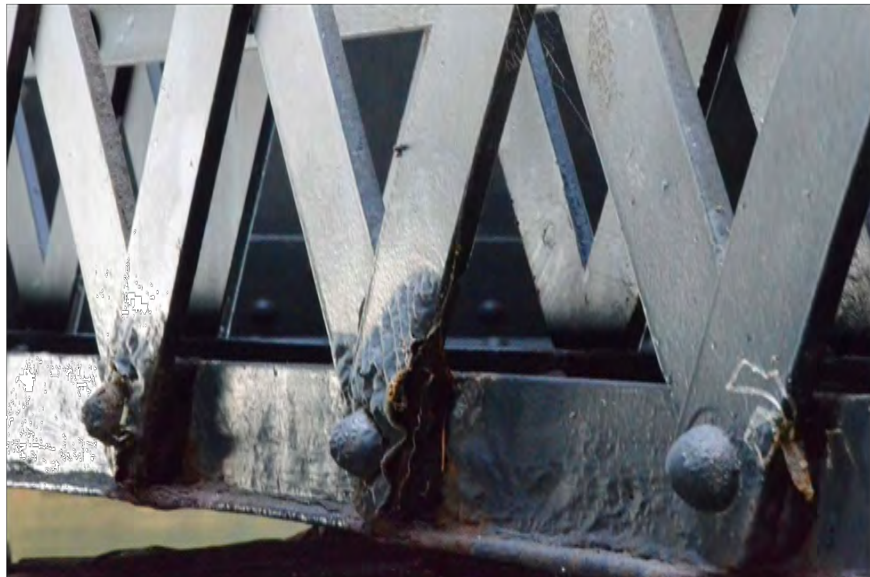
Damaged laces on sway brace EXAMPLE OF REPAIR WORK
