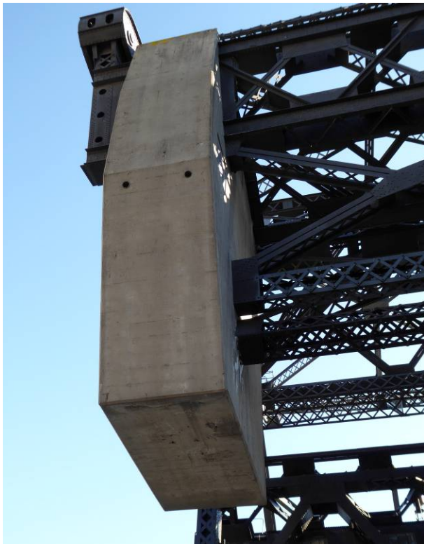
Photograph 19: East concrete counterweight; facing south.
