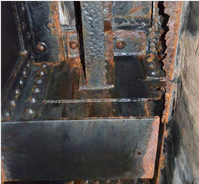
At Pier 1, looking up at cantilver stingers north of Floor Beam 16B EXAMPLE OF REPLACEMENT WORK
