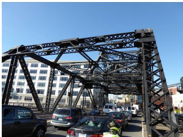
Photograph 3: Steel Through truss, facing northwest.
