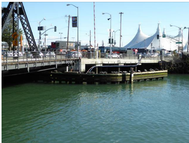
Photograph 29: Wood fenders and piles on southwest corner of bridge; facing south.
