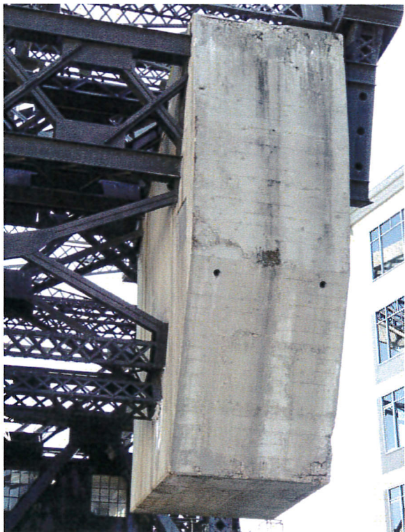
Photograph 23: West concrete counterweight; facing south.
