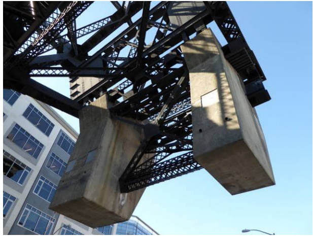
Photograph 18: Concrete counterweights facing northwest.
