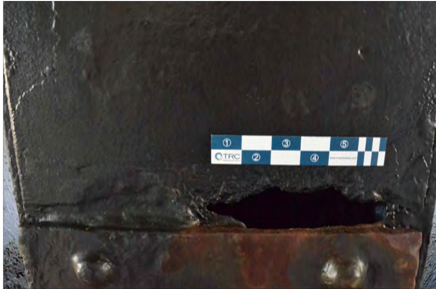
Looking up a hole in sway brace just south of Floor Beam 10 EXAMPLE OF REPAIR WORK
