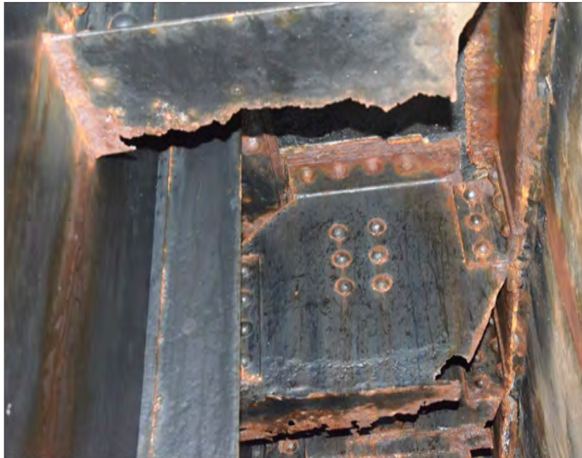
At Pier 1, looking up at cantilver stingers north of Floor Beam 16B EXAMPLE OF REPLACEMENT WORK
