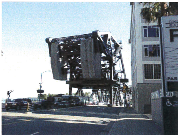
Photograph 15: North side of bridge showing concrete counterweights; facing southeast.
