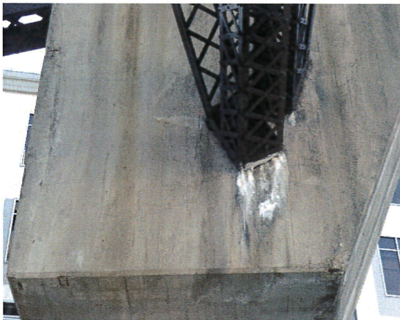
Photograph 21: West side of east counterweight, showing damage near bottom where attached to girder, facing east.
