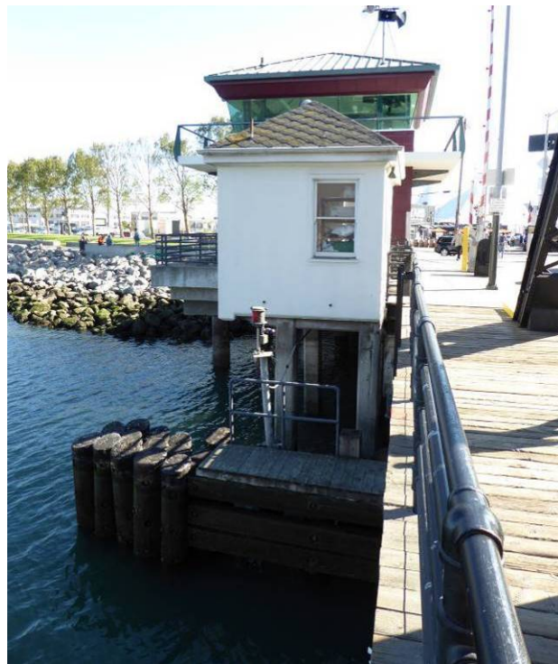
Photograph 28: Watchman's House, showing concrete piles and wood fender piles in foreground; facing south.
