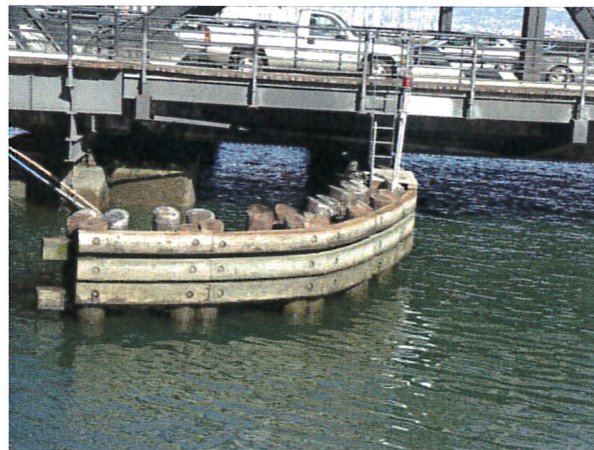
Photograph 36: Wood fender and piles on northwest corner of bridge; facing east.
