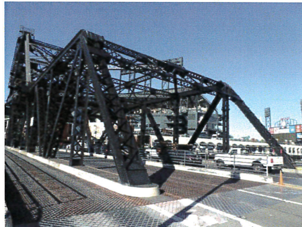
Photograph 2: Showing through truss and metal grate deck on southbound lanes, facing northeast.
