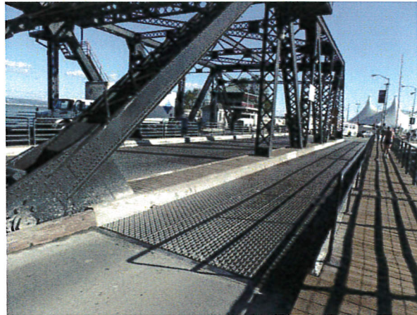
Photograph 6: Steel grate deck for southbound traffic and pressure treated wood sidewalk; facing southeast
