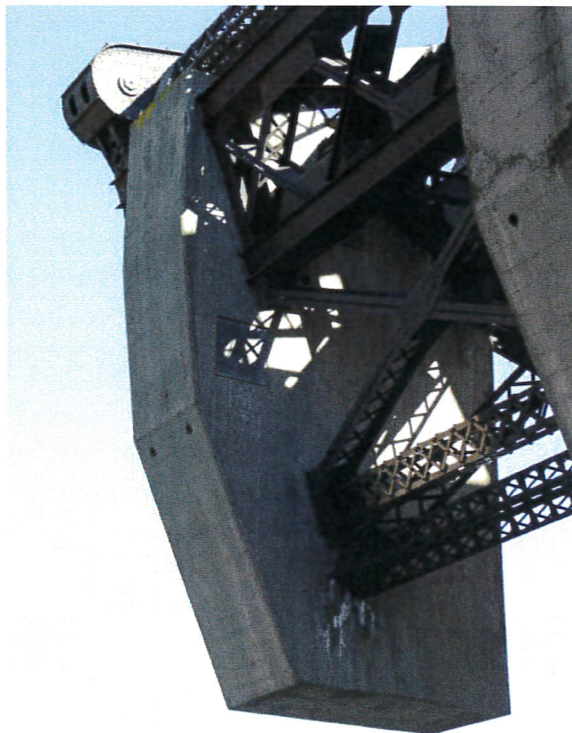
Photograph 20: East concrete counterweight; facing southeast.
