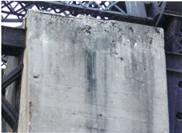
Photograph 25: West concrete counterweight, showing deterioration on top corner, facing south.
