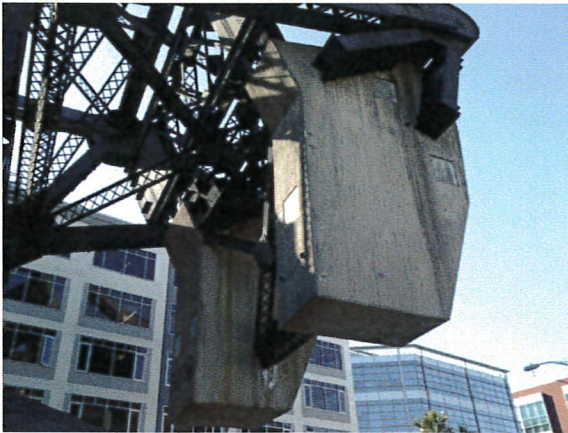
Photograph 17: Concrete counterweights; facing west.
