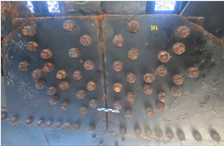
Gusset plate connecting Floor Beam 6 and bottom chord of west truss EXAMPLE OF REPAIR WORK (NOTE THAT FASTENERS WILL BE REPLACED)
