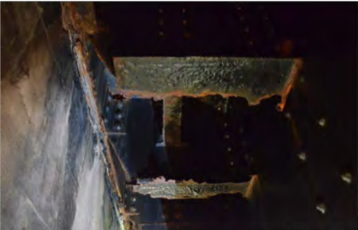
Photo 1: Floorbeam 16 Corroded Stringer Members
