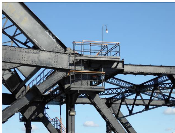
Photograph 14: Second link pin in trunnion system; facing southeast.
