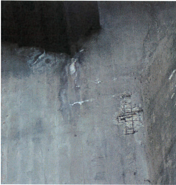
Photograph 29: West side of west counterweight, showing deterioration in areas near top, facing east.
