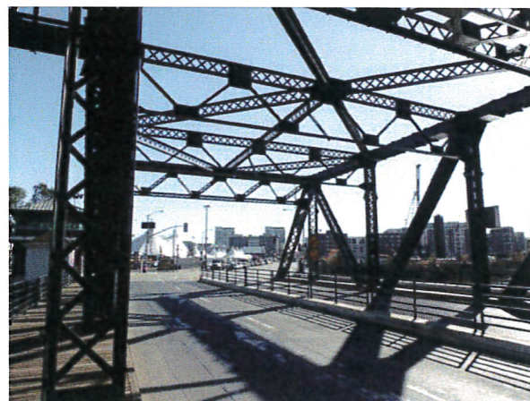
Photograph 4: Showing steel through truss and steel deck with composite surface with decorative plank design on northbound lanes; facing southwest.
