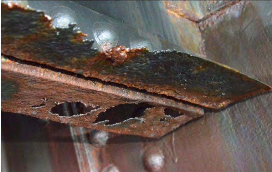
Bottom flange of stringer EXAMPLE OF REPLACEMENT WORK
