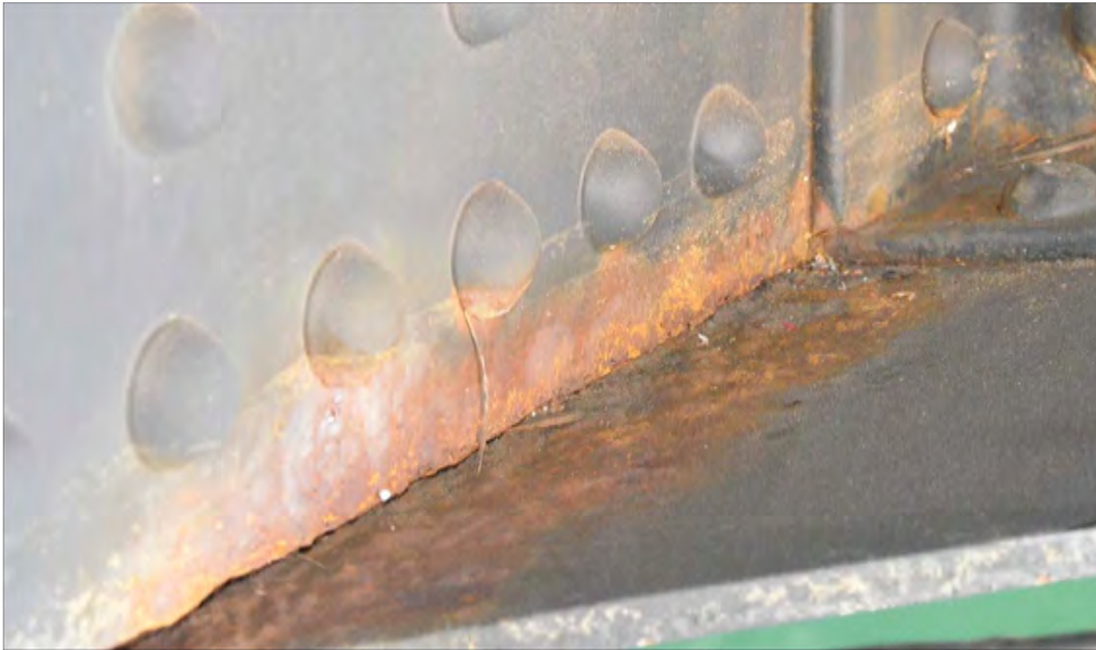
Top of gusset plate under west cantilever EXAMPLE OF REPAIR WORK
