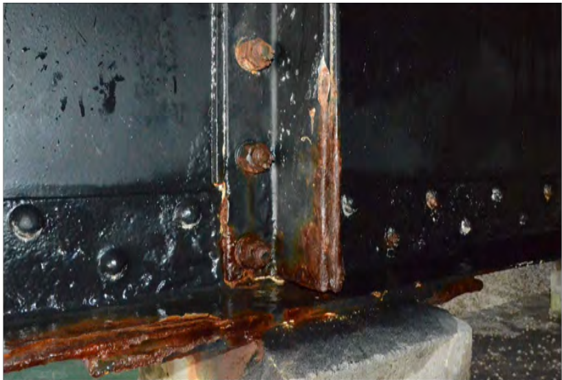
Looking at stiffener on north face of Floor Beam 12 EXAMPLE OF REPAIR WORK
