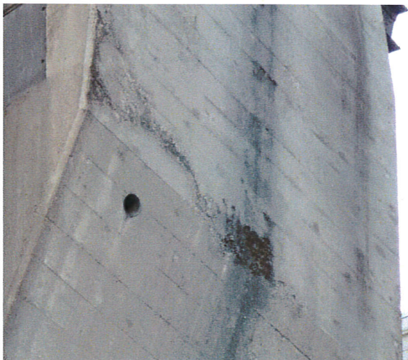
Photograph 27: North side of west counterweight, showing areas of deterioration, facing southwest.
