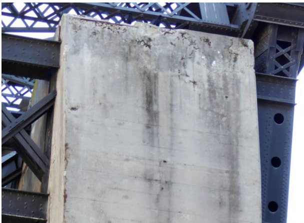
Photograph 23: West concrete counterweight, showing deterioration on top corner, facing south.
