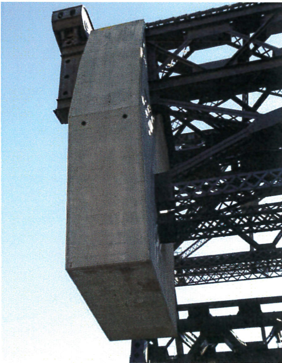
Photograph 19: East concrete counterweight; facing south.
