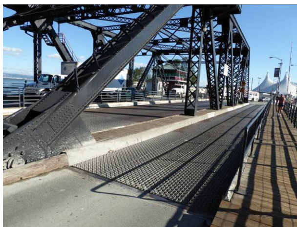
Photograph 6: Steel grate deck for southbound traffic and pressure treated wood sidewalk; facing southeast
