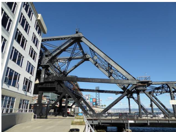
Photograph 11: Trunnion section of bridge; facing east.
