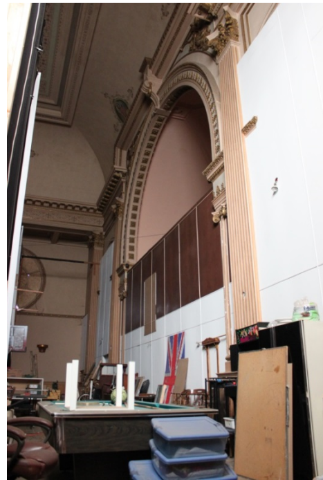
FIGURE 32. CHURCH: SANCTUARY SHOWING SEALED ALTAR NICHES, 2016.
