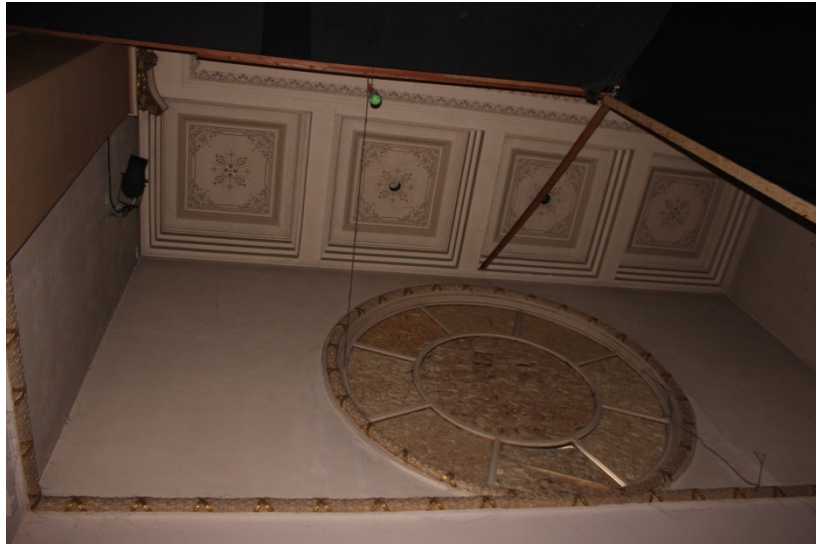
FIGURE 30: CHURCH: NORTH TRANSEPT SHOWING DECORATIVE DETAILING, 2016.
